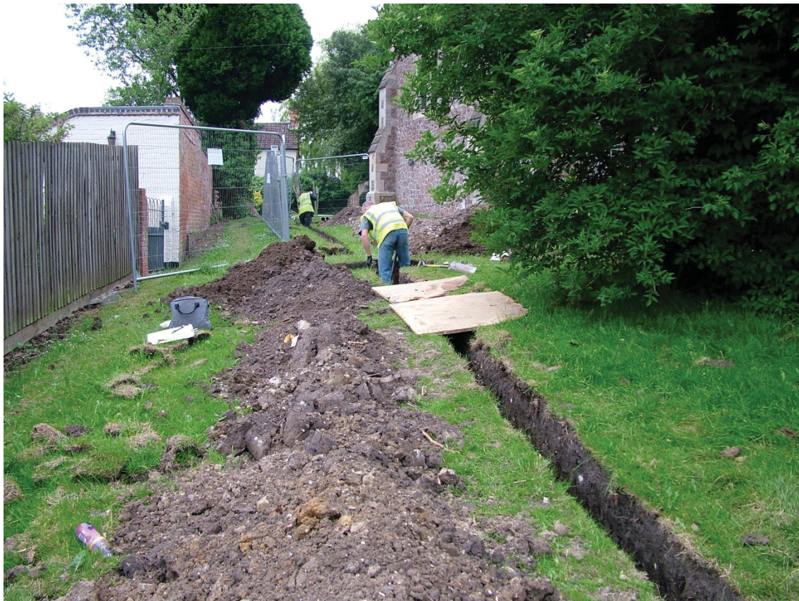
Figure 3: Work in progress, looking south-west
