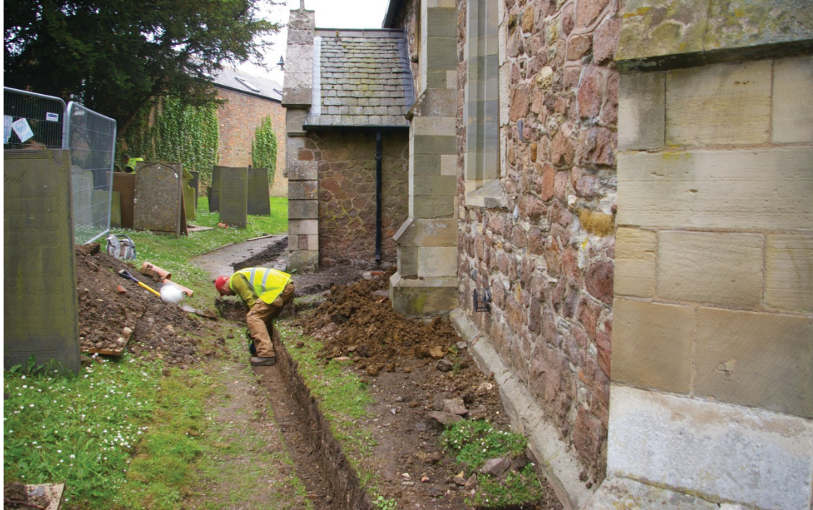
Figure 5: Work in progress around manhole, looking west
