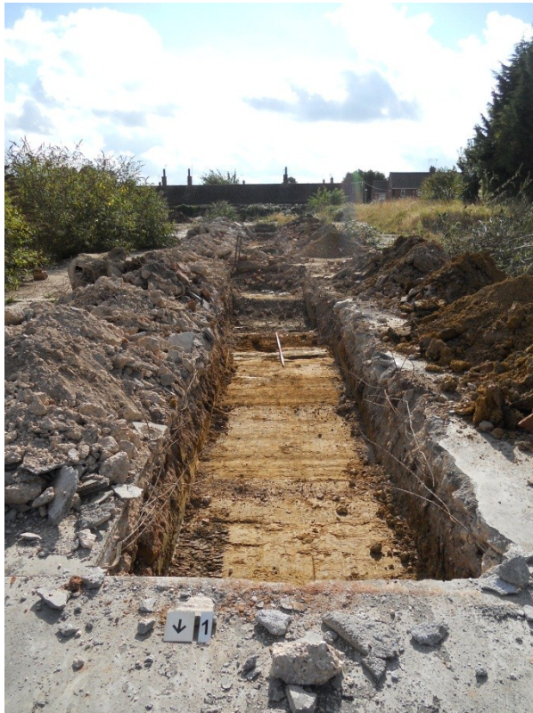
Figure 3: Trench 1, looking south
