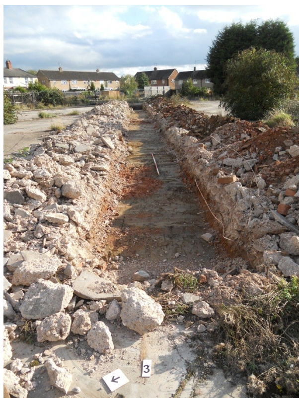
Figure 5: Trench 3, looking south-east
