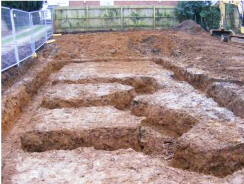
Figure 4: Trenches on the east side of the site, looking south
