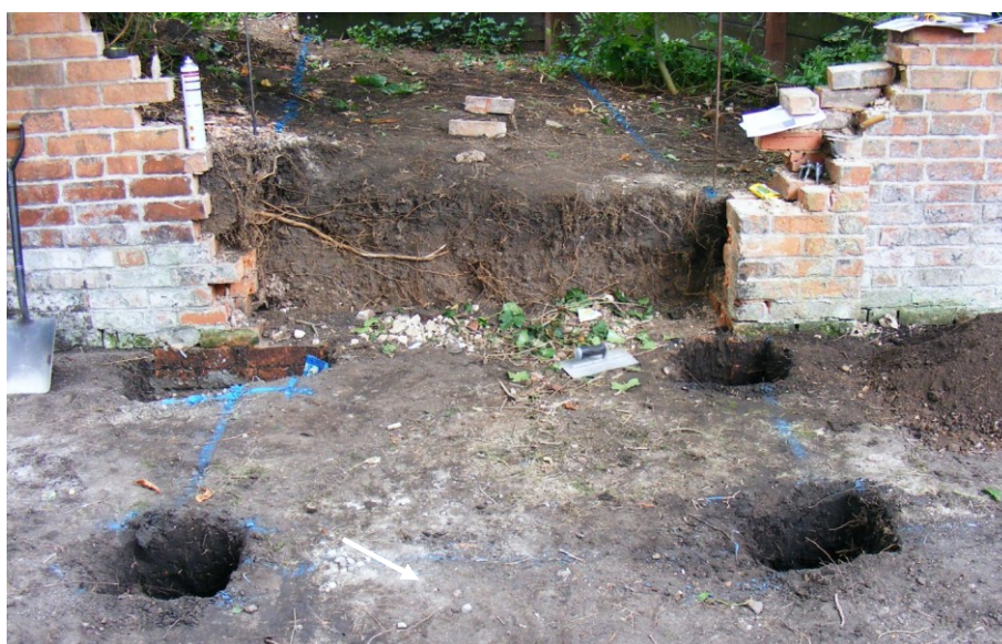
Figure 7: Cross section through the build-up behind the garden wall. Post holes 1-3 in foreground. Looking south.
