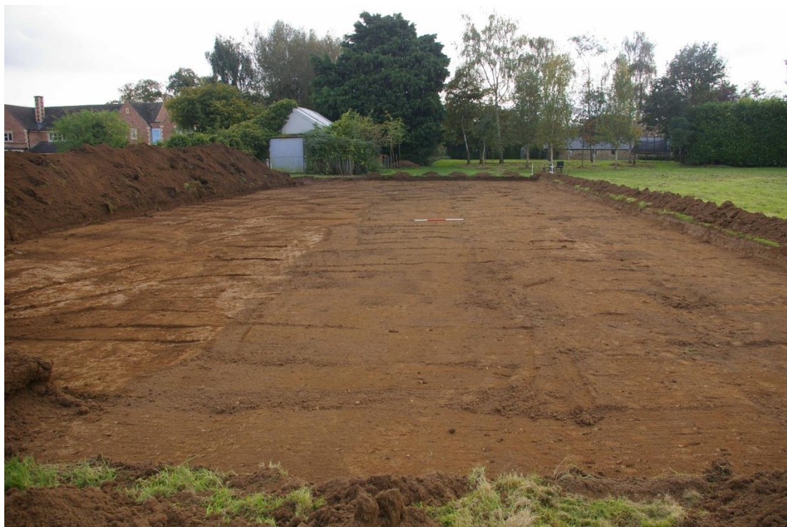
Figure 5 Tennis court after topsoil strip Looking south. 1.5m scale
