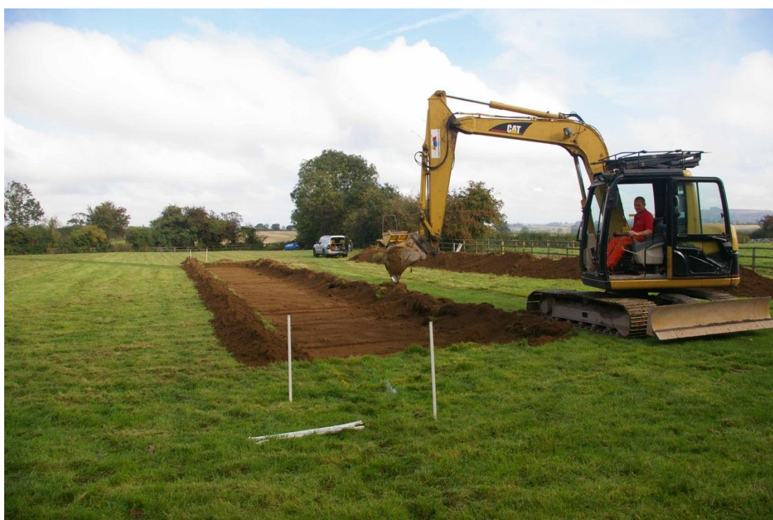
Figure 4 Initial topsoil strip Looking north-east.
