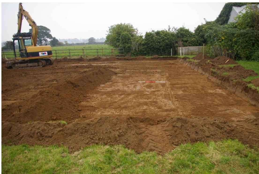
Figure 6 Southern area subsoil reduction Looking east. 1.5m scale
