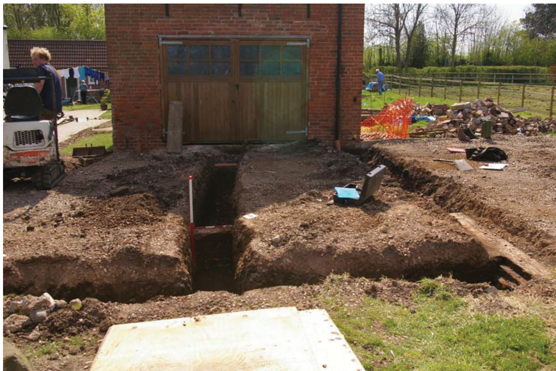
Figure 8 Exposed wall in central trench
