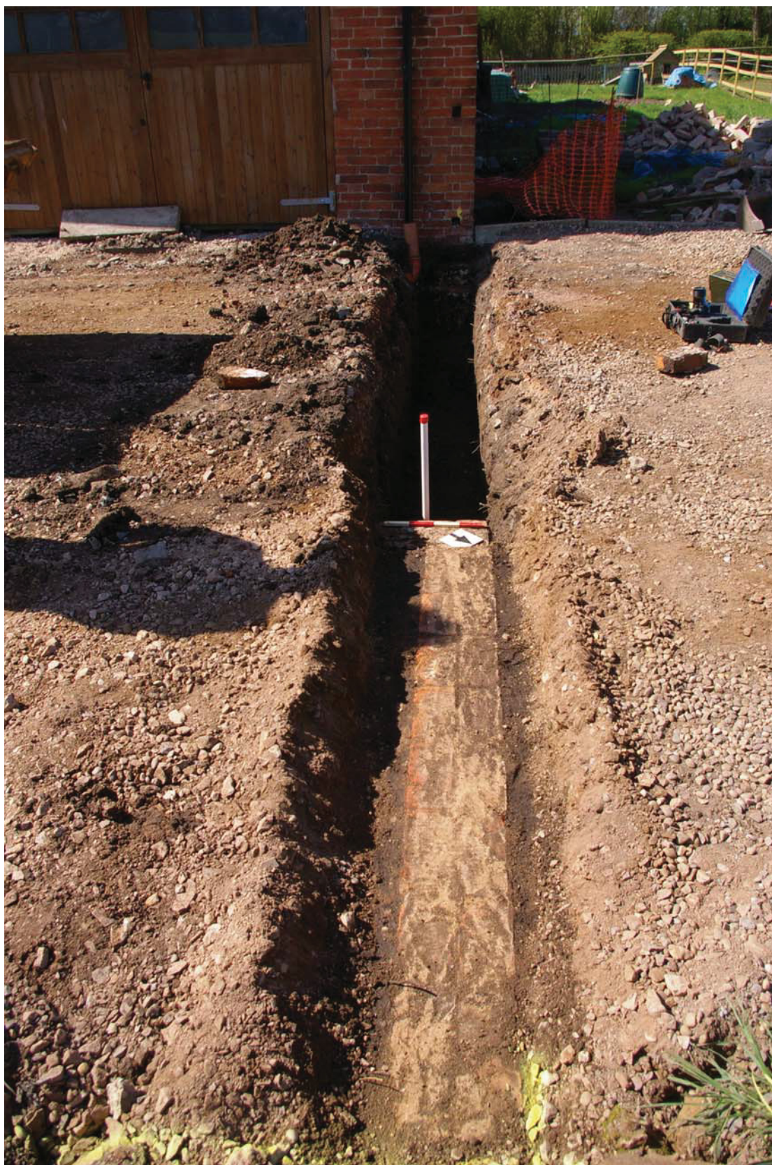
Figure 6 Exposed wall foundation in western trench Looking south-west
