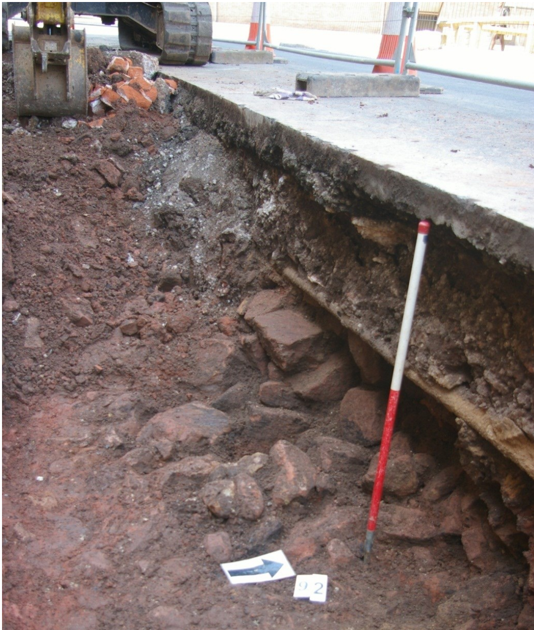
Figure 32: Rubble (92) seen in Grove Street trench
