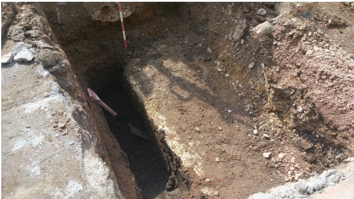
Figure 4: Initial test-pit to identify base of stanchion (at end of spade) showing garden soils only
