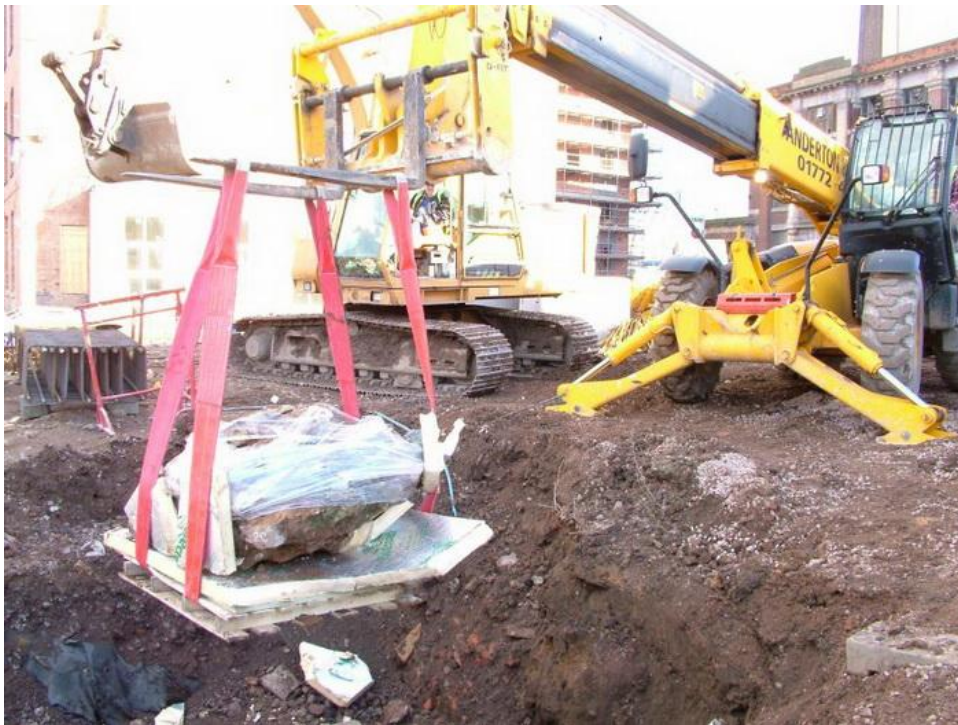
Figure 18 Lifting the town wall fragment
