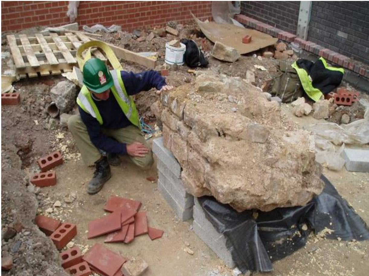
Figure 19 Consolidating the town wall fragment
