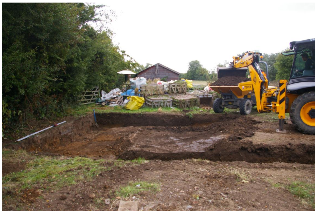
Plate 5: Work in progress on complete strip, looking east
