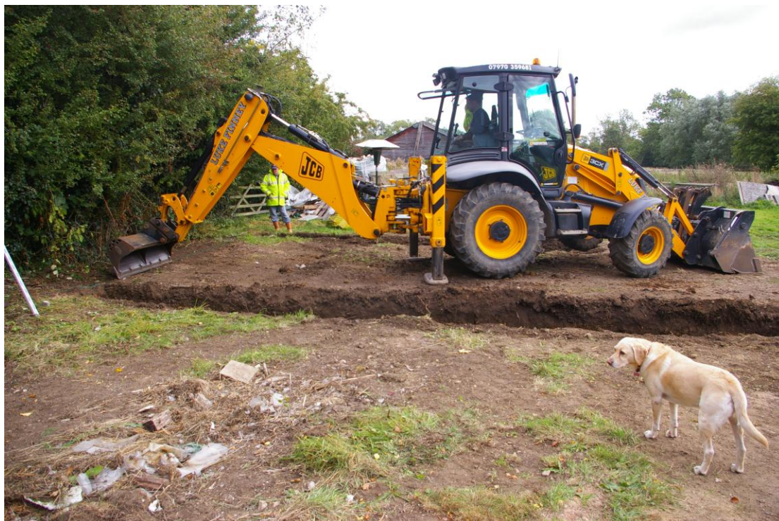
Plate 3: Work in progress on initial trench, looking east
