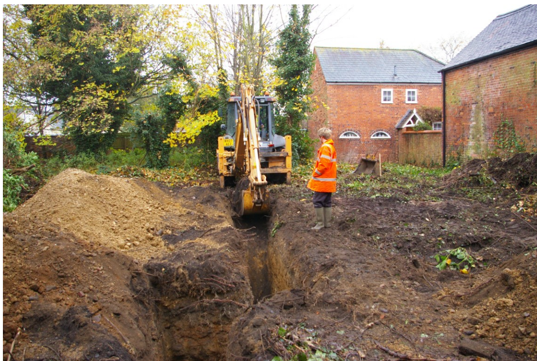
Plate 1: Work in progress, looking south
