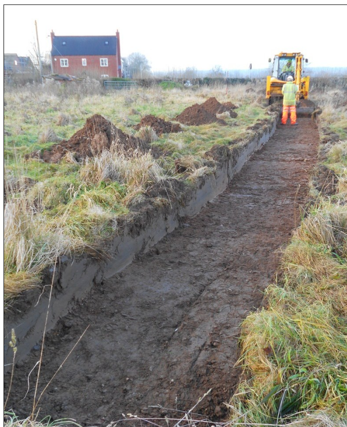
Figure 2: Machining in progress; view west
