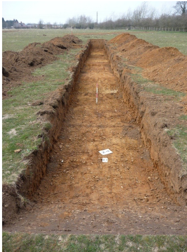
Figure 5: Trench 7: view northwest; 2m scale
