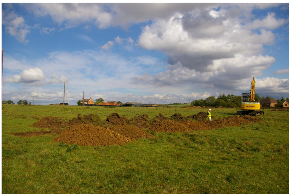
Plate 1: Work in progress on Trench 08, looking north-east to Scalford Road Lodge
