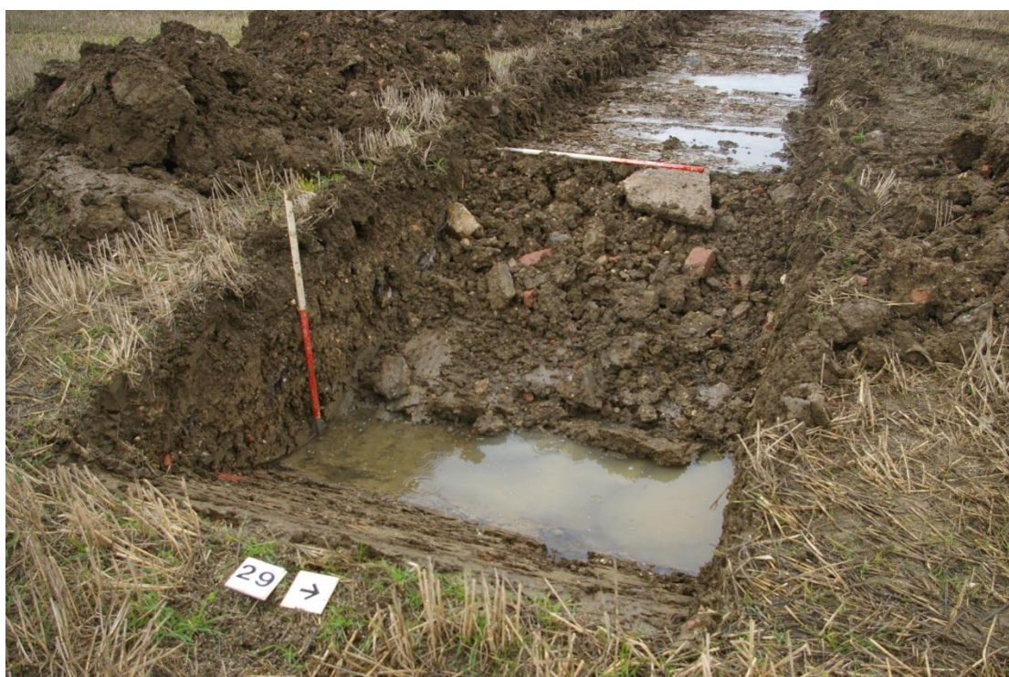
Plate 13: Trench 29, showing depth of made up ground, looking south-west
