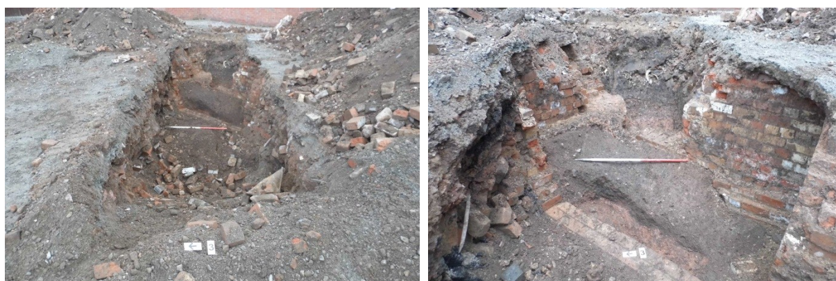
Figure 7: Left – Trench 3, looking east; right – the eastern end of Trench 3, looking east
