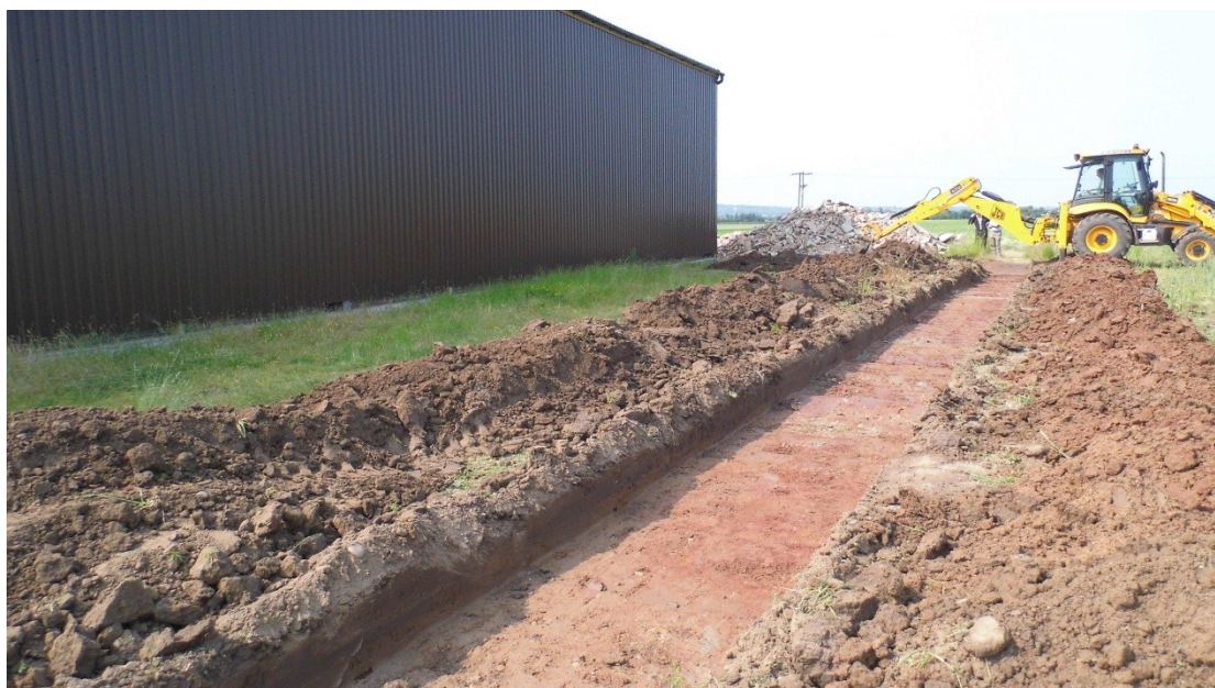
Figure 3: Machining in progress: view looking south-west
