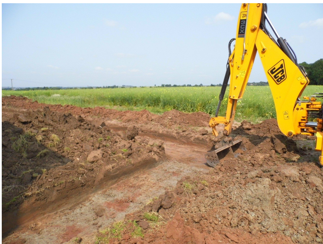
Figure 4: Machining in progress: view looking north-west
