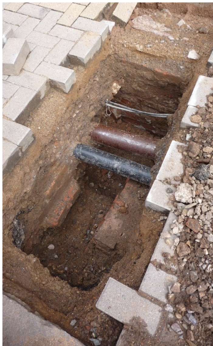
Figure 4: Trial trench 2: view north-west
