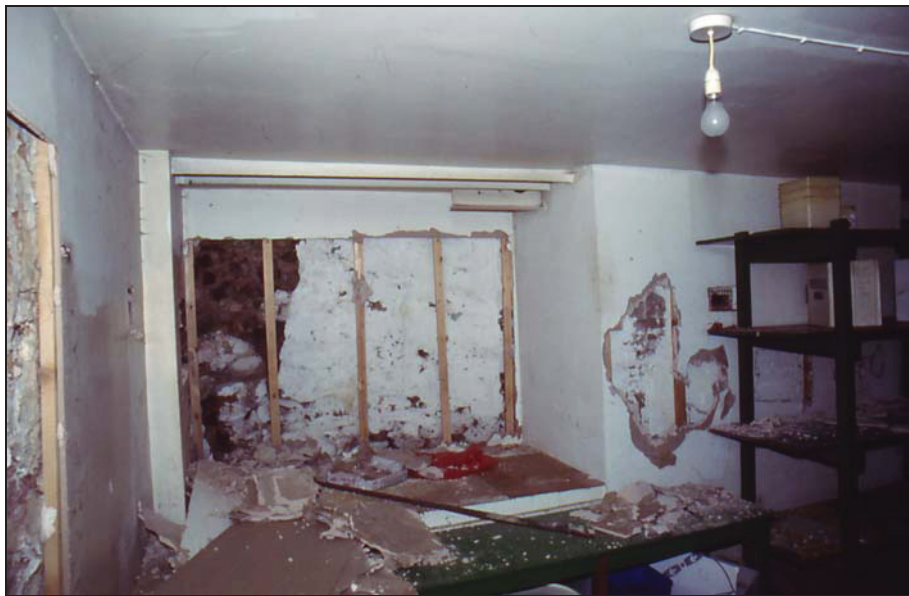
Plate 19. Cellar 1, showing stone wall behind plaster-board. Looking west.
