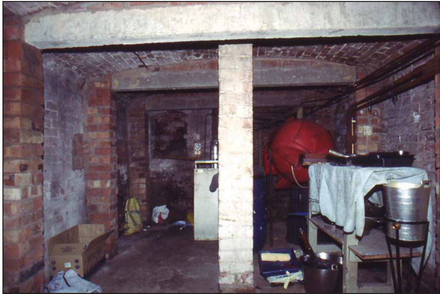
Plate 20. Cellar 2. Looking east.
