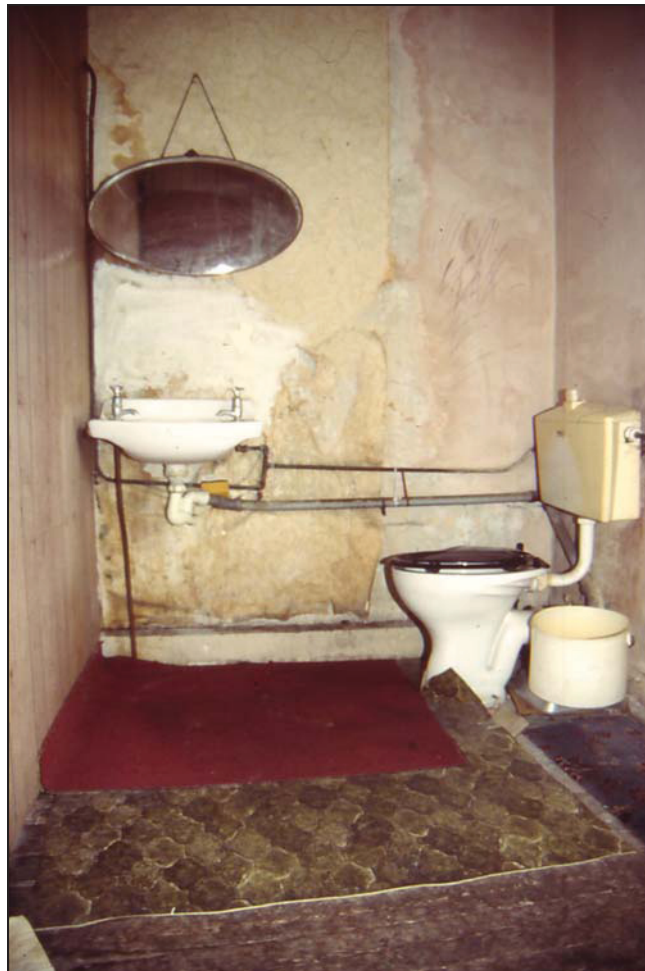
Plate 10. Room 7 Bathroom. Looking north.
