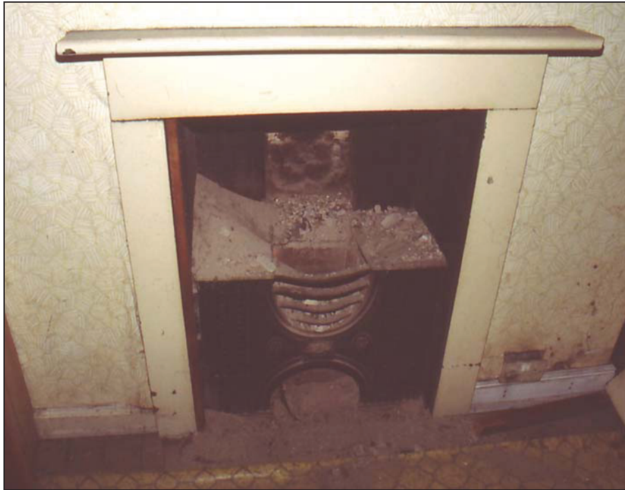
Plate 11. Room 7 fireplace. Looking west.
