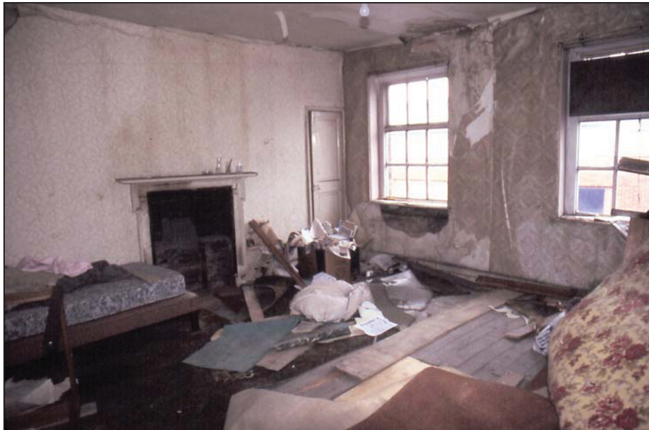
Plate 8. Second floor, Room 6, looking south-west.
