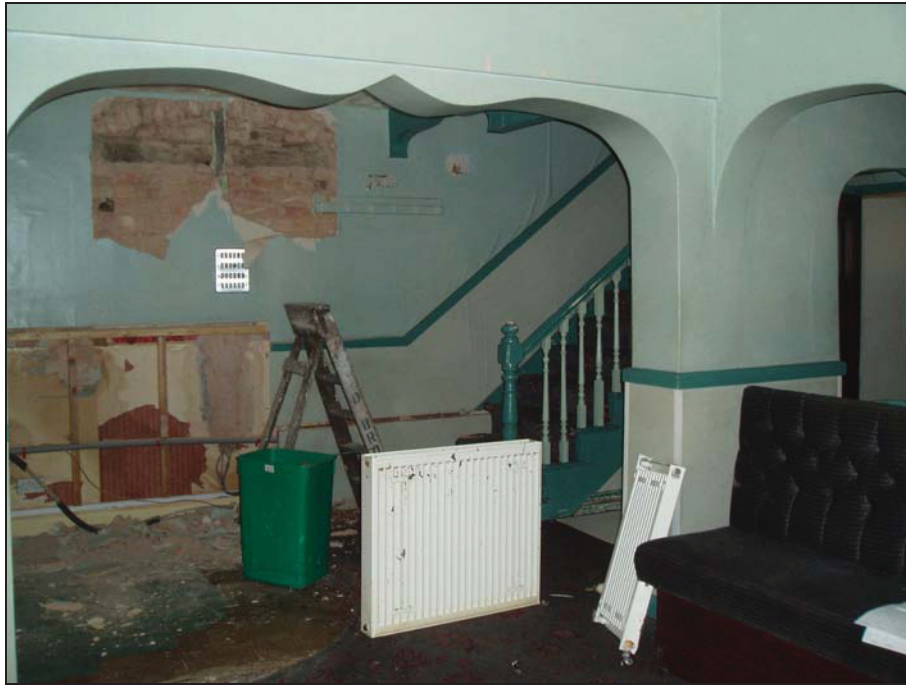
Plate 3. Room 1, showing staircase and blocked doorway through to Room 9. Looking north.
