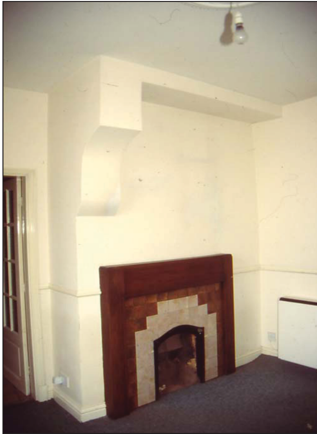
Plate 15. Room 11. c. 1910/20 fireplace within chimney stack. Looking east.
