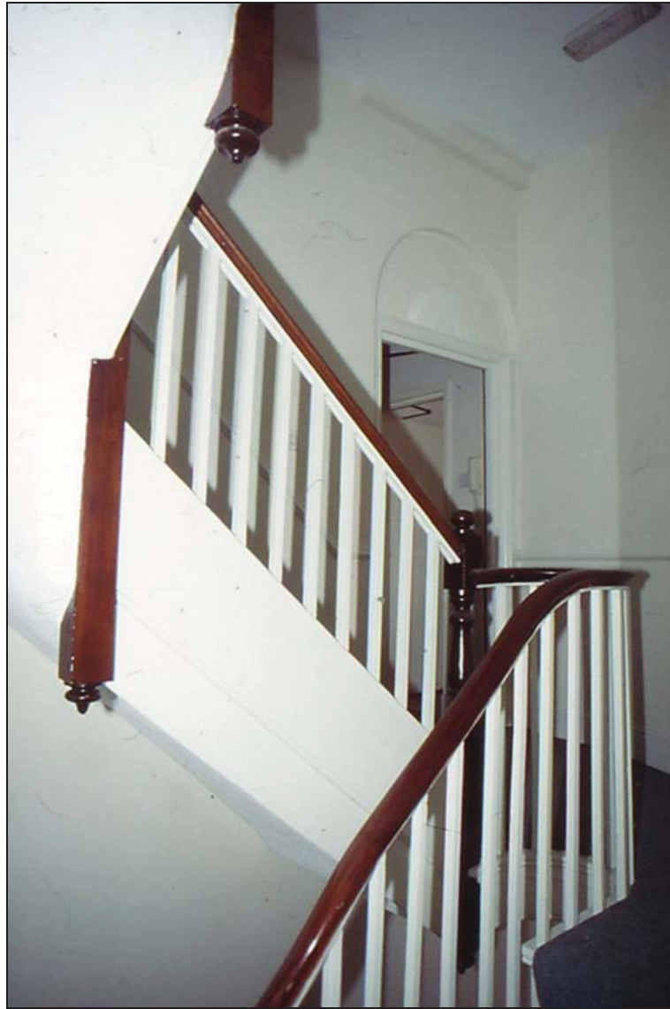
Plate 17. 59a service staircase, showing position of former 1 st floor passage into Room 13. Looking north-west.
