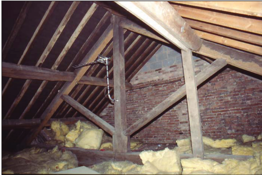
Plate 24: King-post roof structure above Rooms 17 and 18, frontage range. Looking north.
