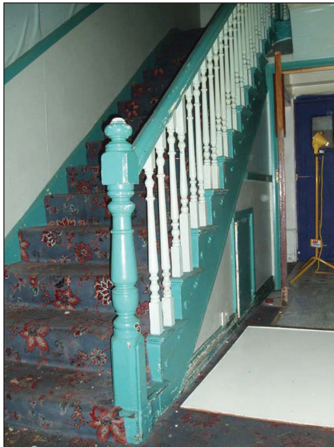
Plate 4. 59 Highcross Street, ground floor staircase detail. Looking east.
