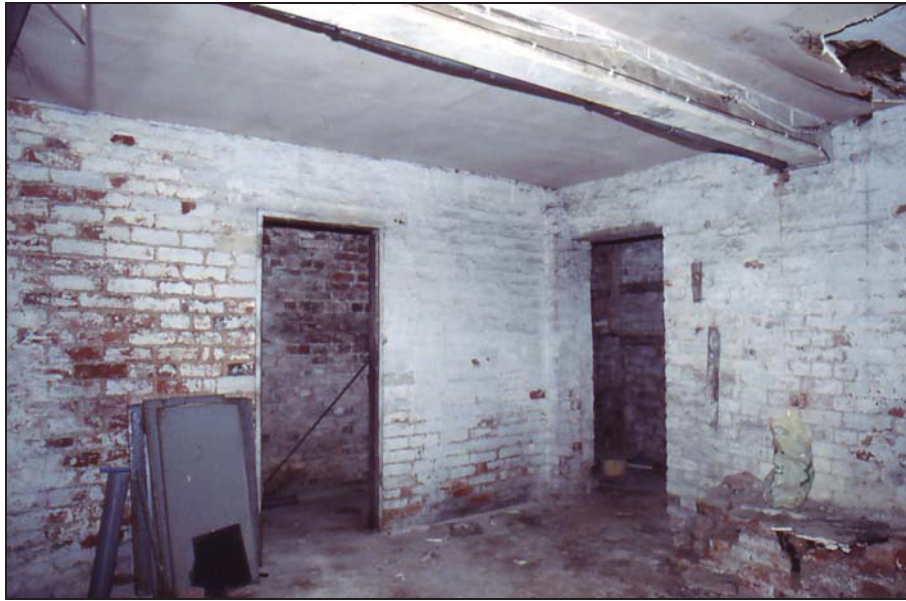
Plate 22. Cellar 4. Looking south.
