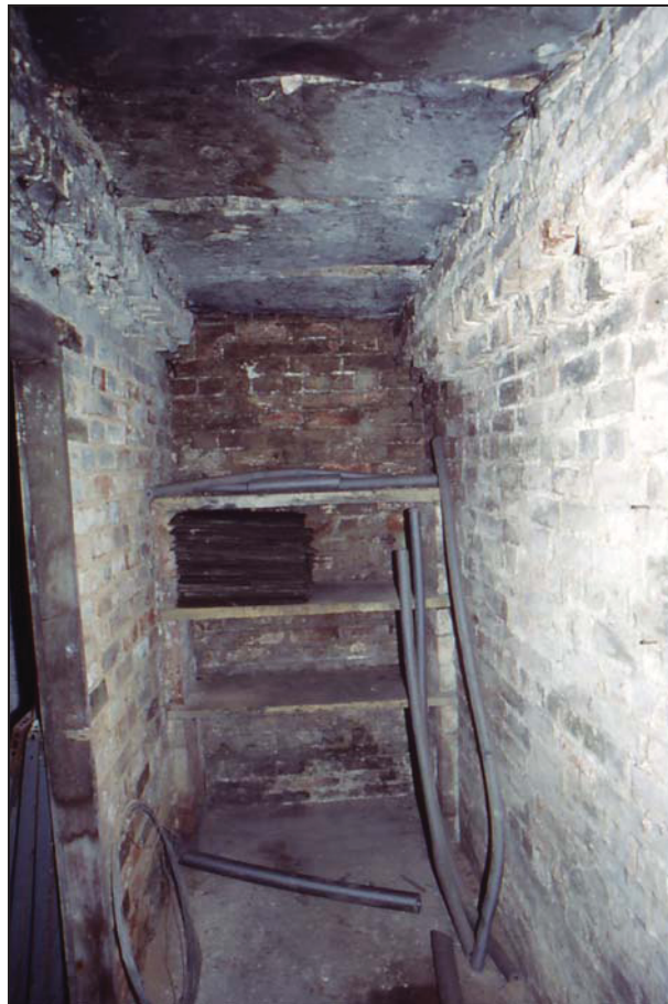
Plate 23. Cellar 5. Looking east.
