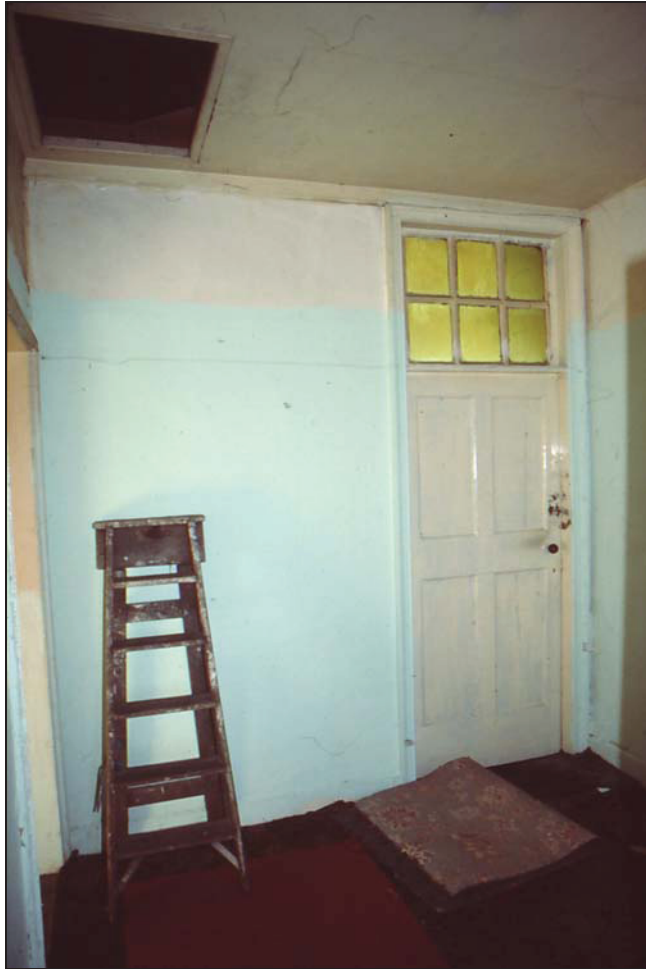
Plate 13. Second floor landing, four-panel door to Room 8, with overlight. Looking north-west
