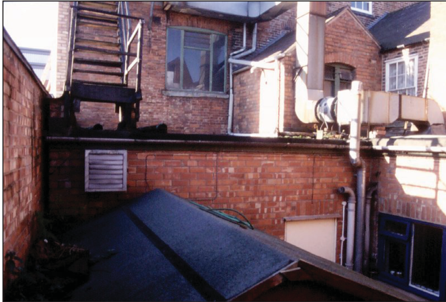
Figure 2. Rear of 59 Highcross Street showing the late 20th century single storey flat roofed range (centre of frame).
