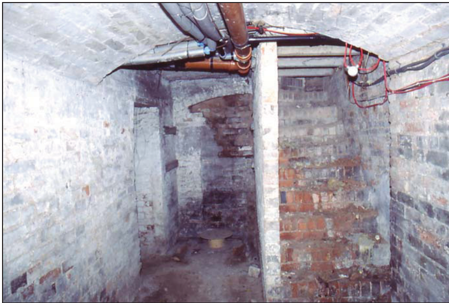
Plate 21. Cellar 3, showing blocked staircase leading up to 59a Highcross Street and blocked doorway through to cellars of number 59 to the left. Looking south.
