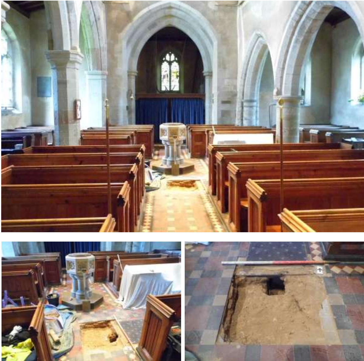
Figure 3: top, church nave looking west; bottom left, location of test pit in church floor; bottom right, test pit looking north, showing void into brick lined heating duct.
