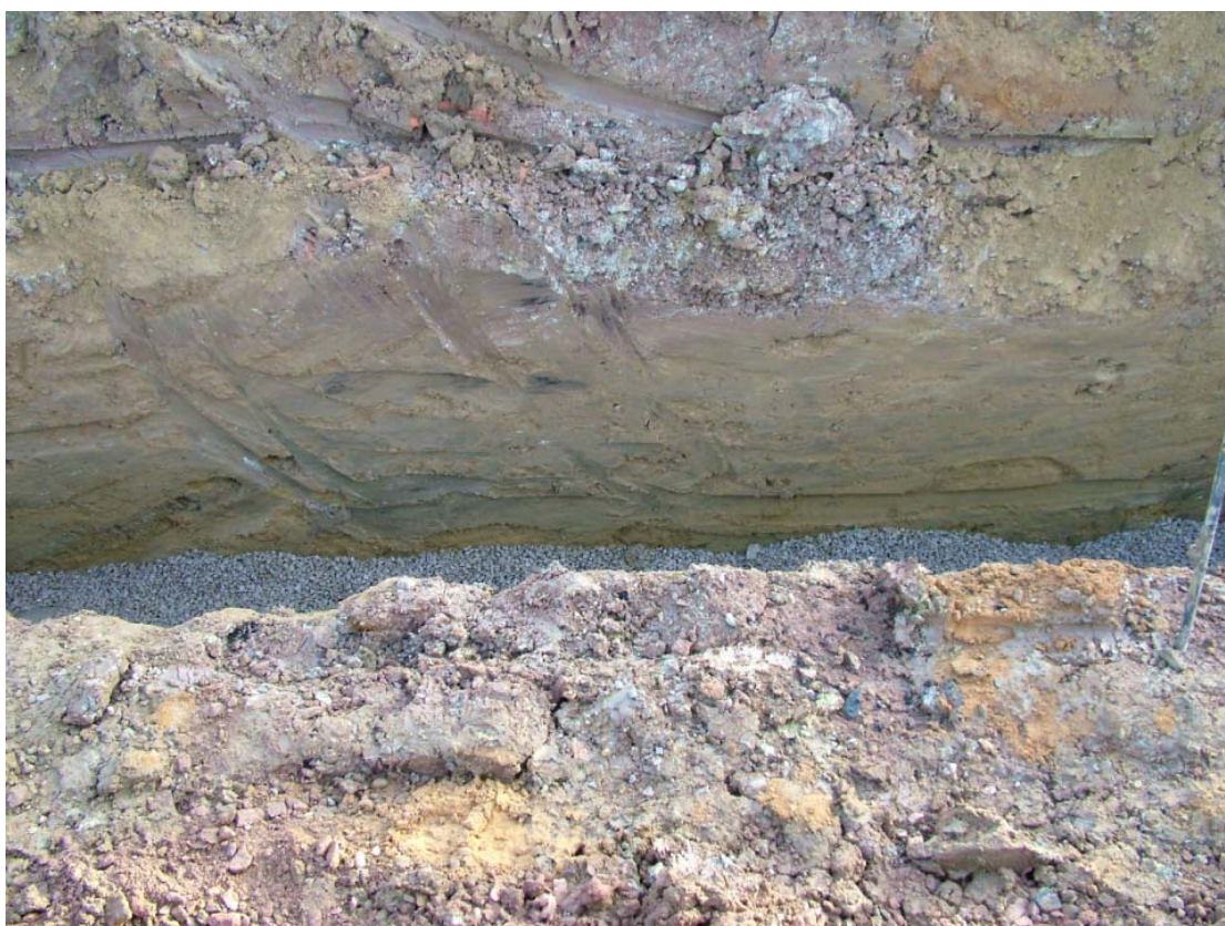
Plate 4: North west facing section of service trench
