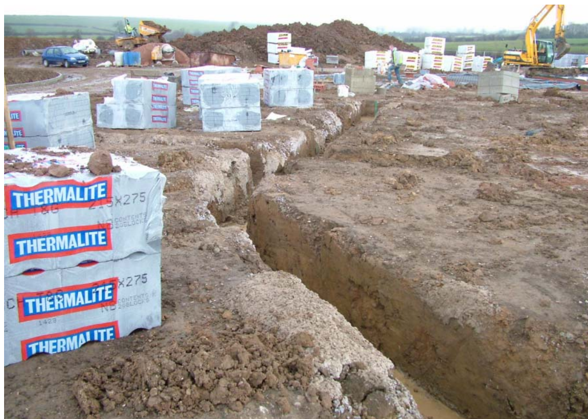
Plate 5: General shot of site with foundation trenches, looking north east
