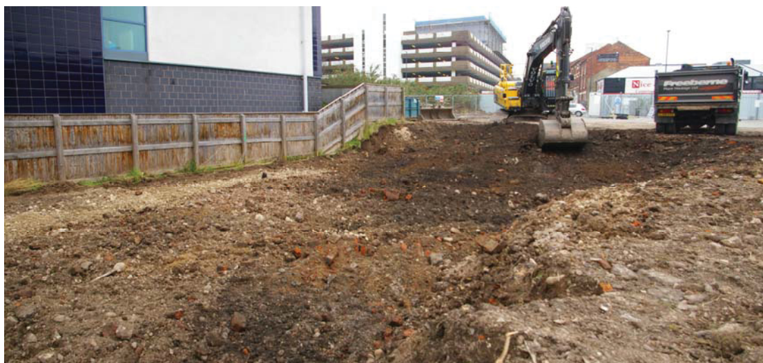
Plate 3: Northern part of site, after removal of tarmac and hardcore
