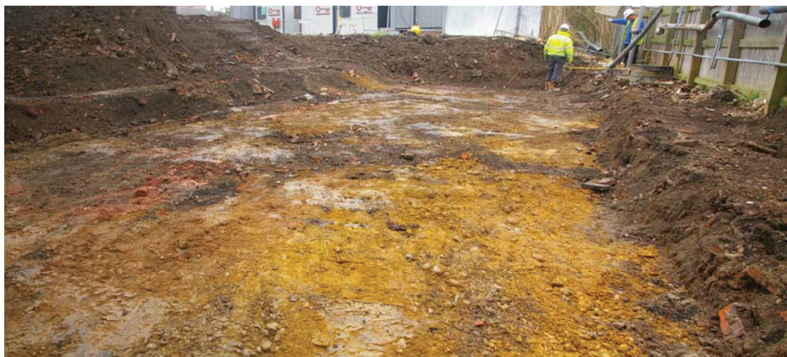
Plate 10: Western side of site complete, looking south
