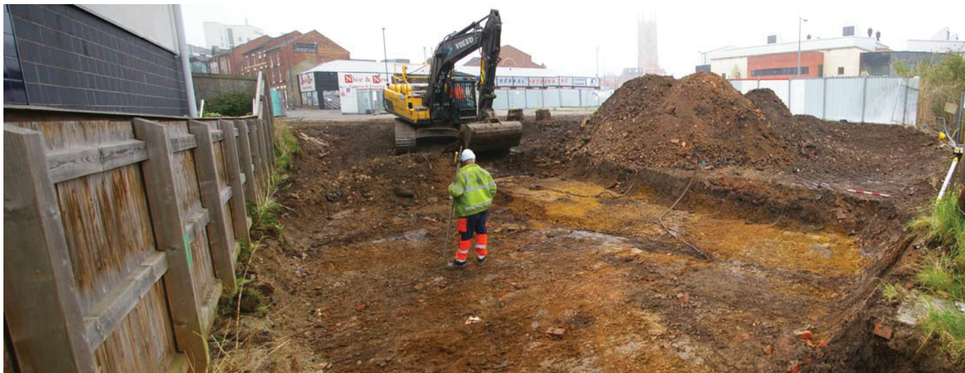
Plate 5: Work in progress on northern side, looking south-east
