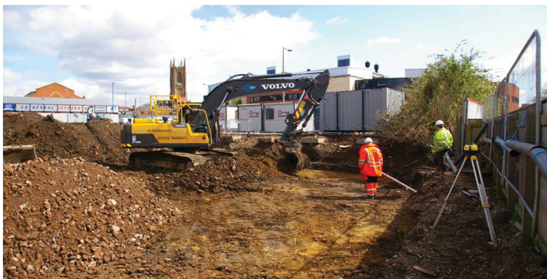
Plate 8: Work in progress on southern side, looking south
