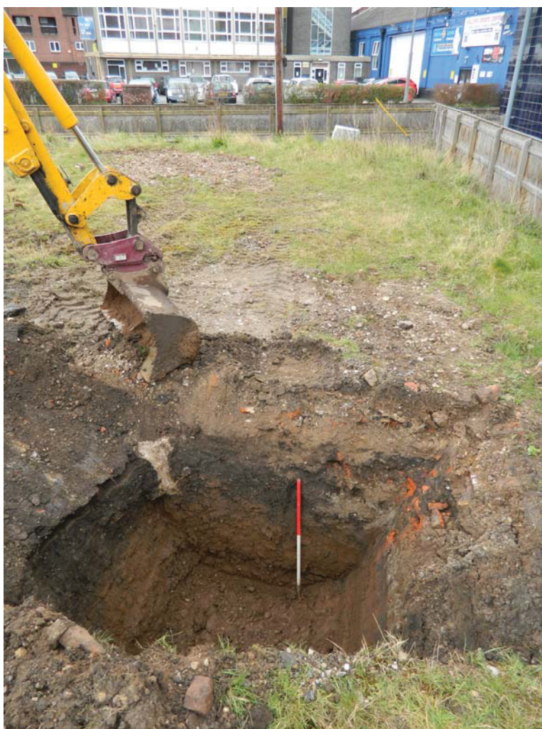
Plate 2: Test pit 1, looking west
