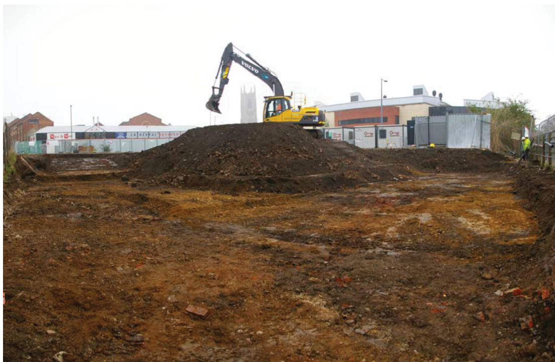
Plate 11: Site mostly complete, looking south-east
