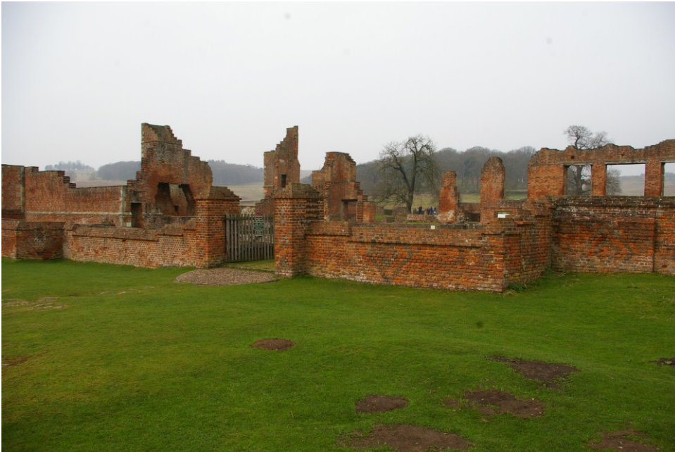
Figure 25: MLE745 Bradgate House ruins Photo 3848 Looking NW
