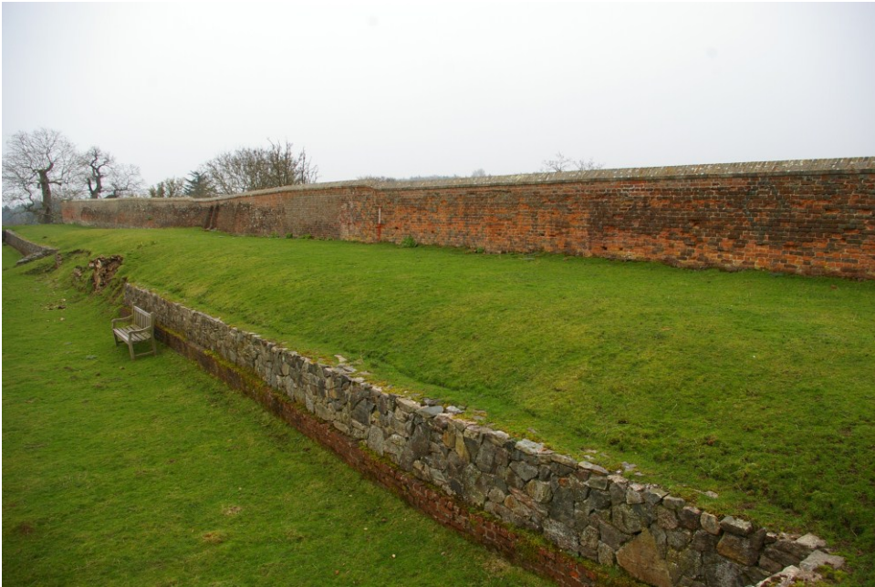
Figure 33: MLE14007 Garden wall Photo 3856 Looking SE
