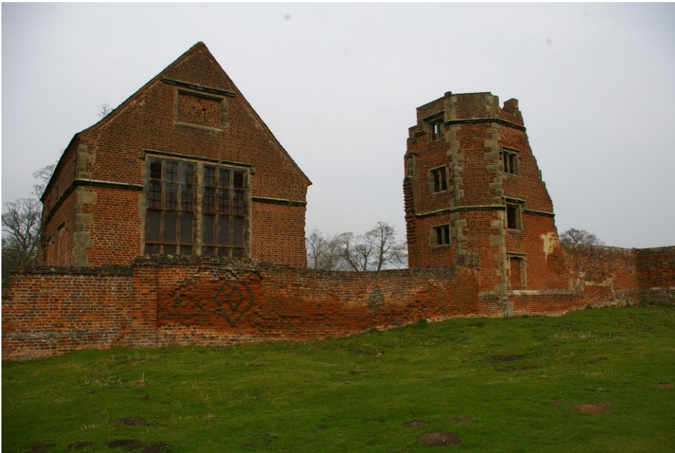
Figure 26: MLE745 ruins plus MLE746 chapel (on left) Photo 3849 Looking NE
