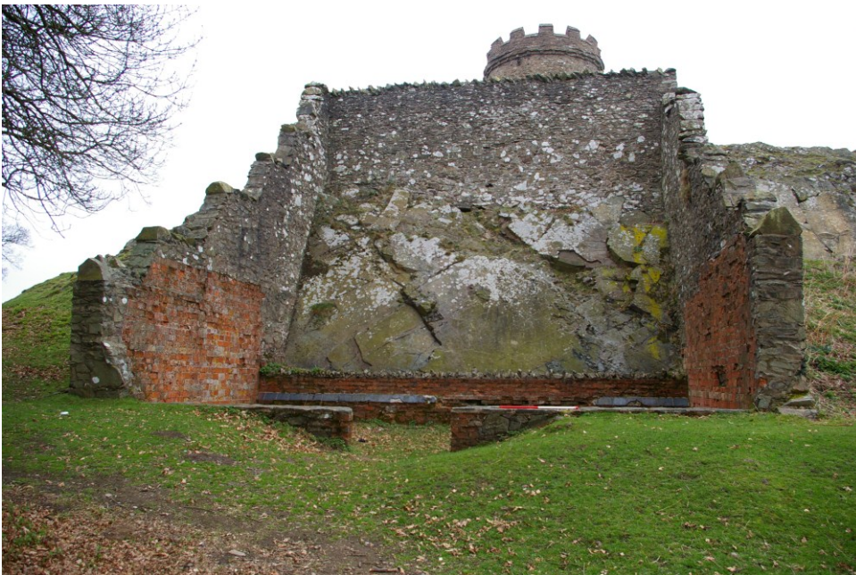
Figure 74: W009 stables Photo 3980 Looking N
