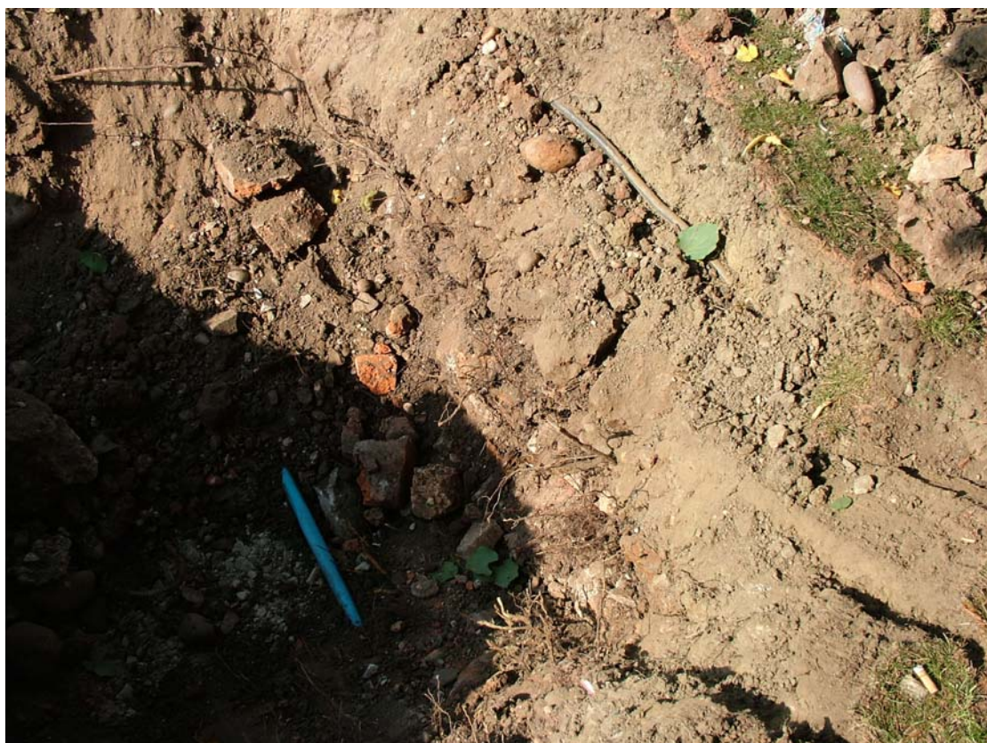
Plate 6: Area 4 trench, showing services encountered, looking west
