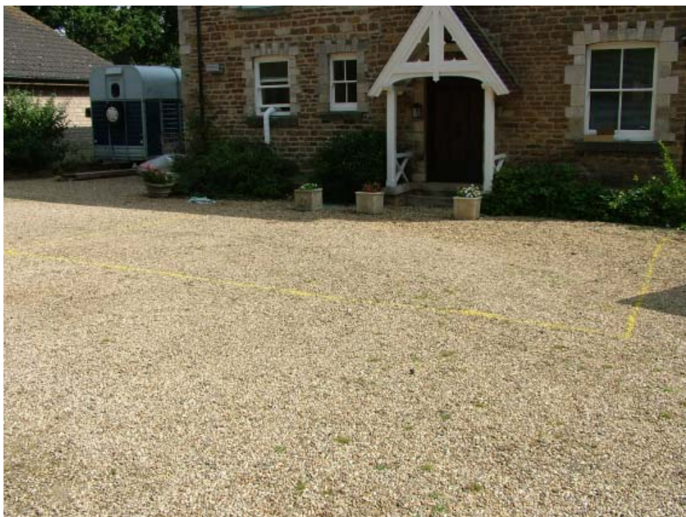
Plate 2: Foundations trenches layout, prior to excavation, looking east
