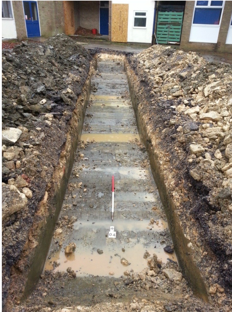
Figure 6: Trench 4; view looking north (1m scale)
