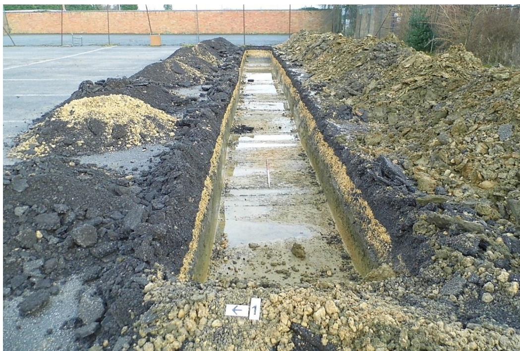
Figure 3: Trench 1; view looking west (1m scale)
