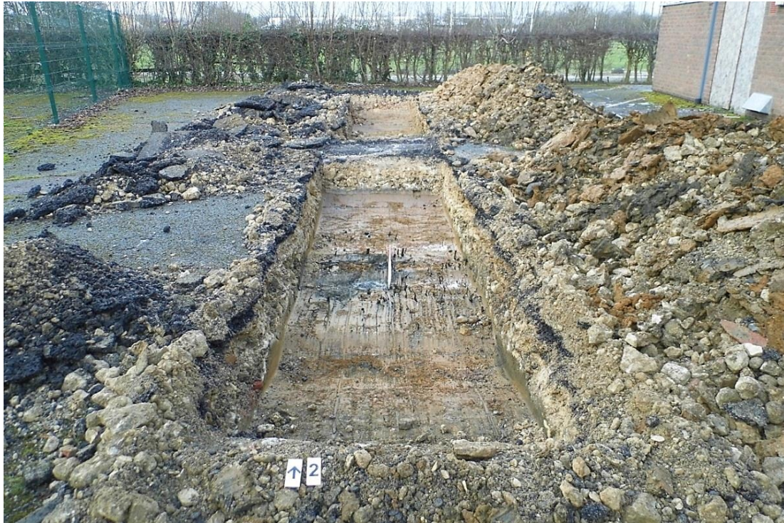
Figure 4: Trench 2; view looking north (1m scale)
