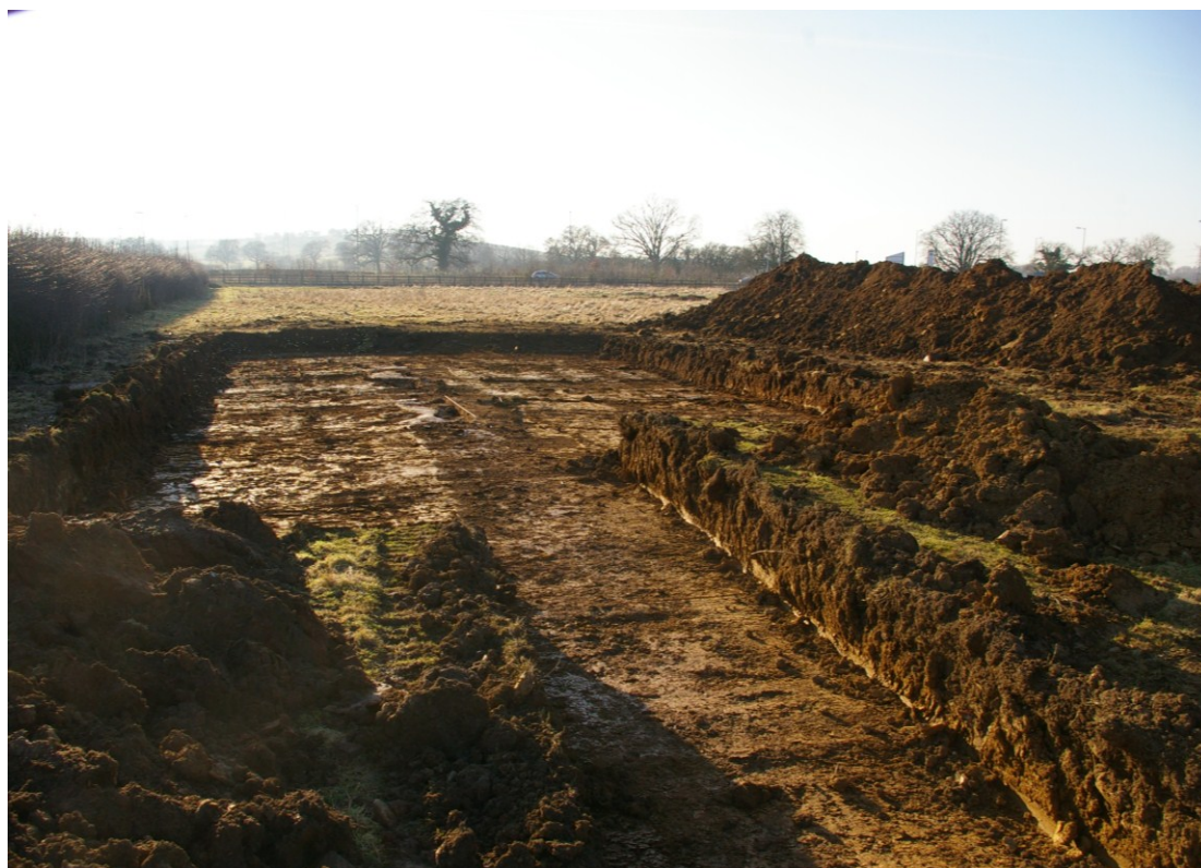
Figure 6 Partially enlarged western end of Trench B Looking west. The trench was later enlarged northwards beneath the spoil heap
