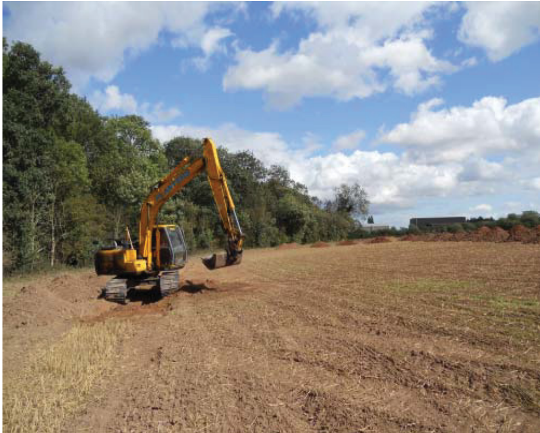
Plate 9 General view of trenches adjacent to northern boundary
