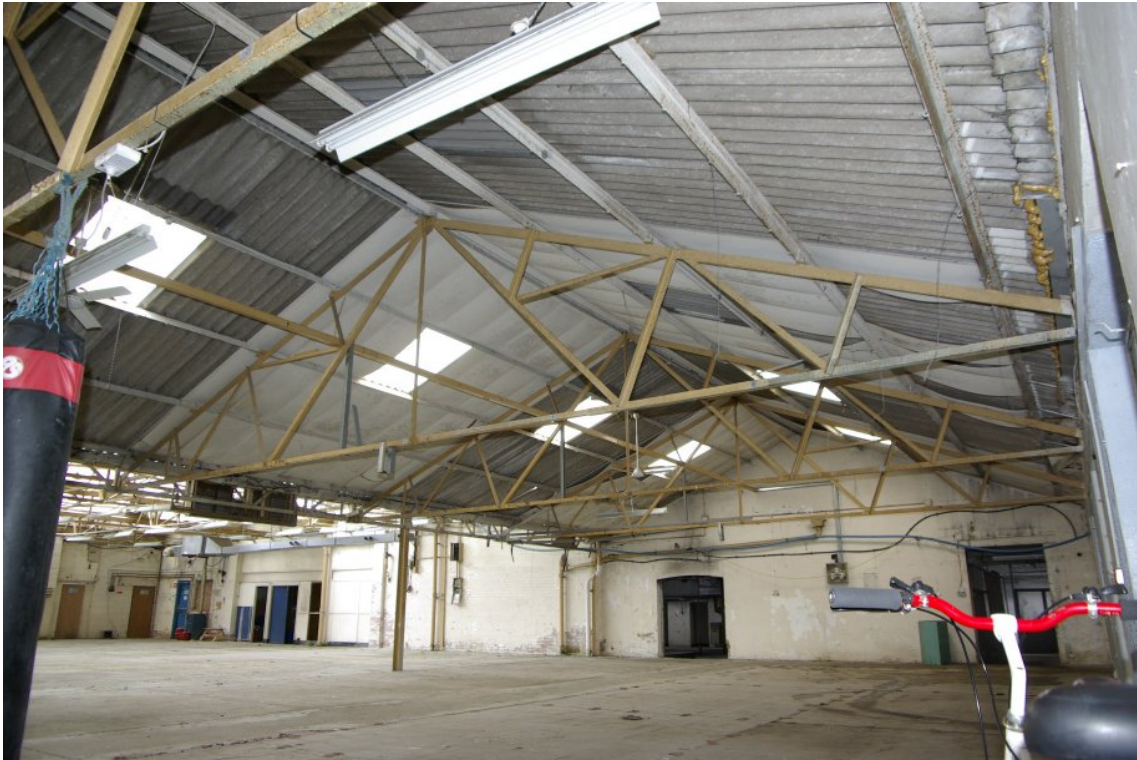
Figure 20 Roof construction within building 3d.
