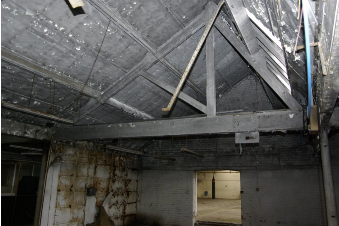
Figure 22 Roof truss within building 4.
