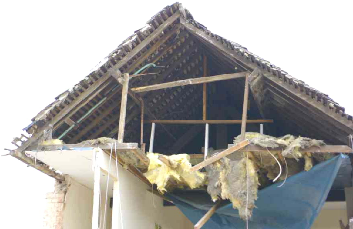
Figure 16 Building 1b, northern end during demolition
