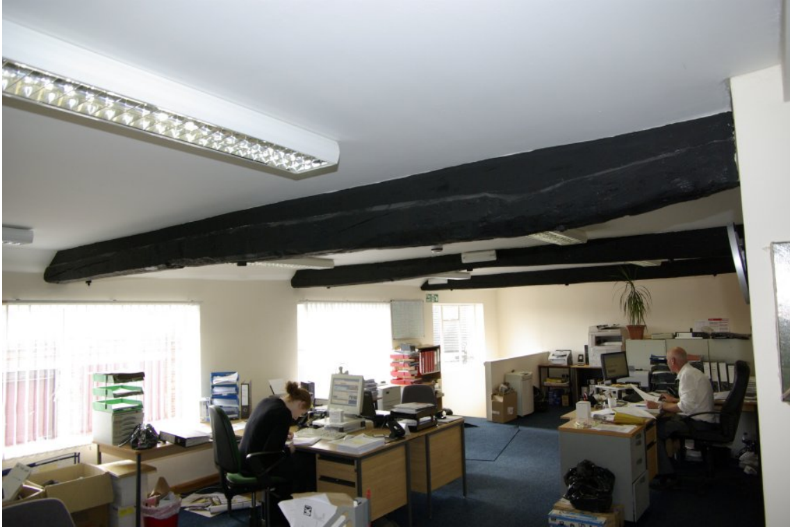
Figure 12 Tie beams visible within building 1b.
