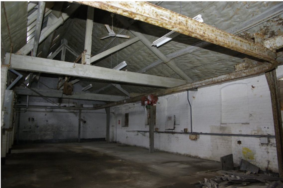
Figure 25 Hoist & tracking mechanism, building 4.
