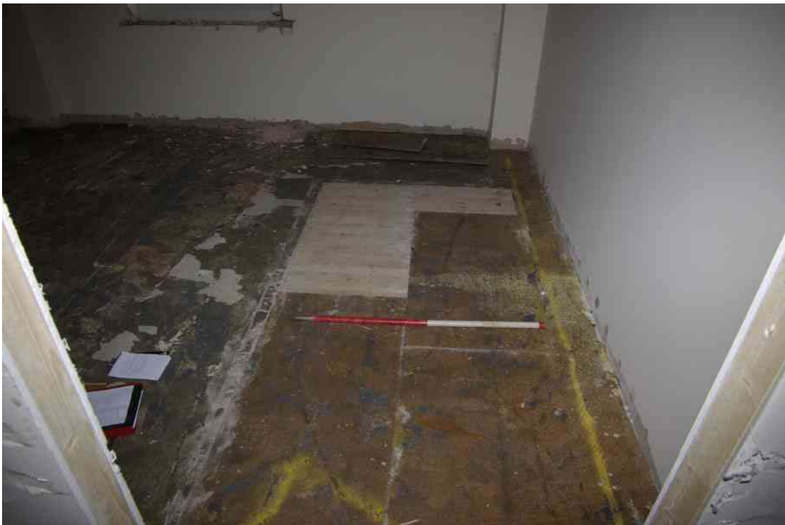
Figure 17 Removed staircase Building 1b, south room northern end
