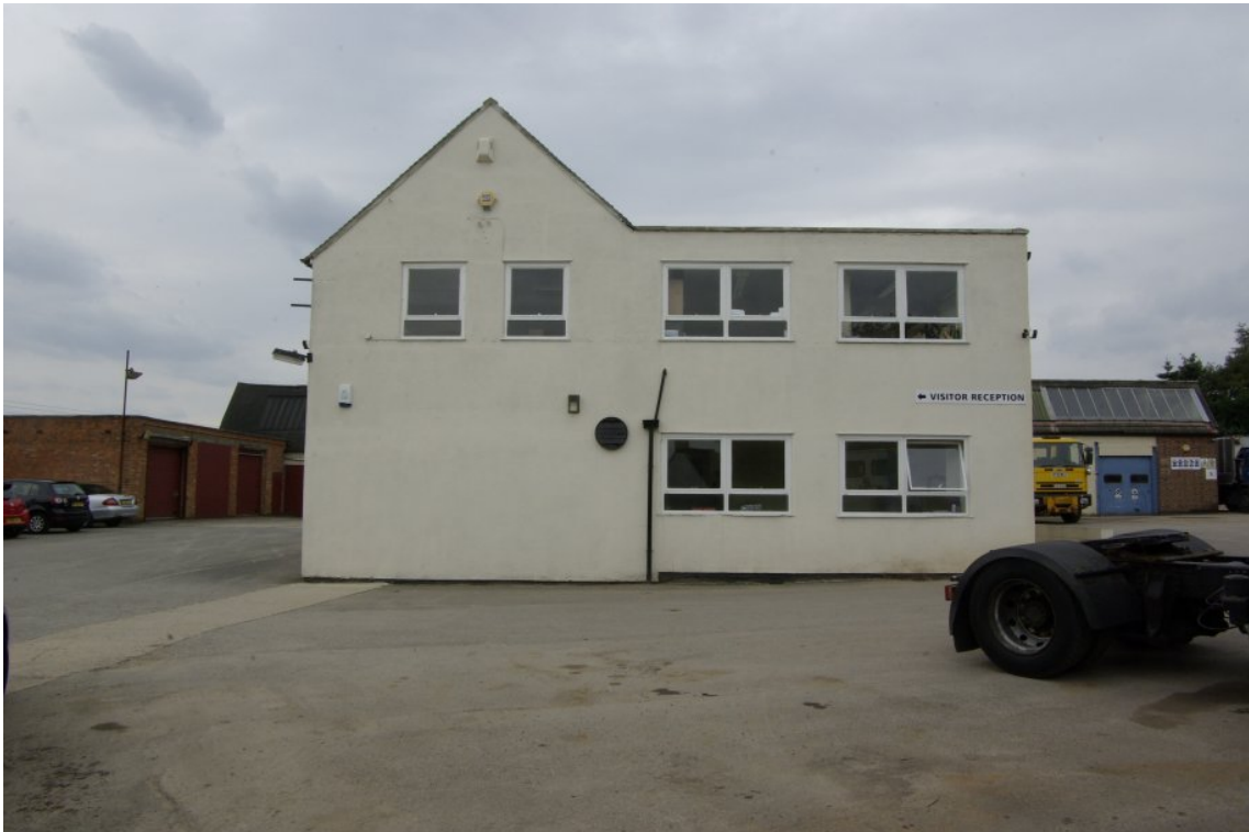
Figure 10 North-facing elevation of building 1.
