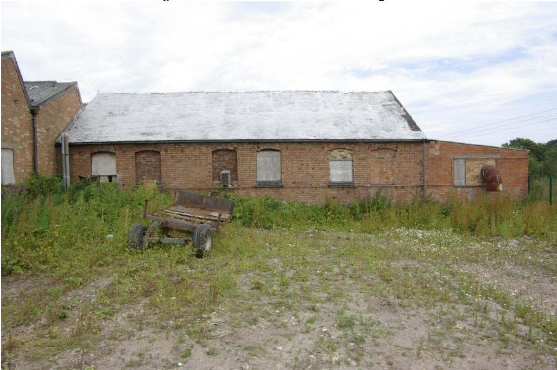
Figure 21 South facing elevation of building 4.
