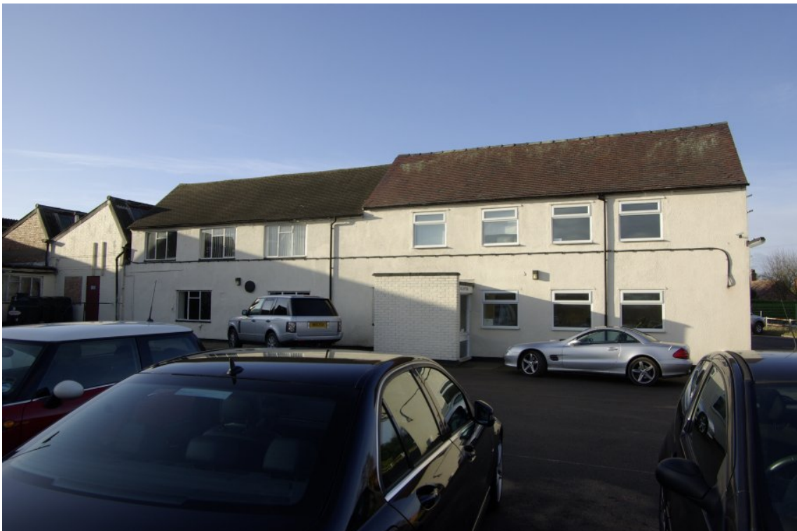
Figure 11 East facing elevation of building 1b, showing change in roof line.
