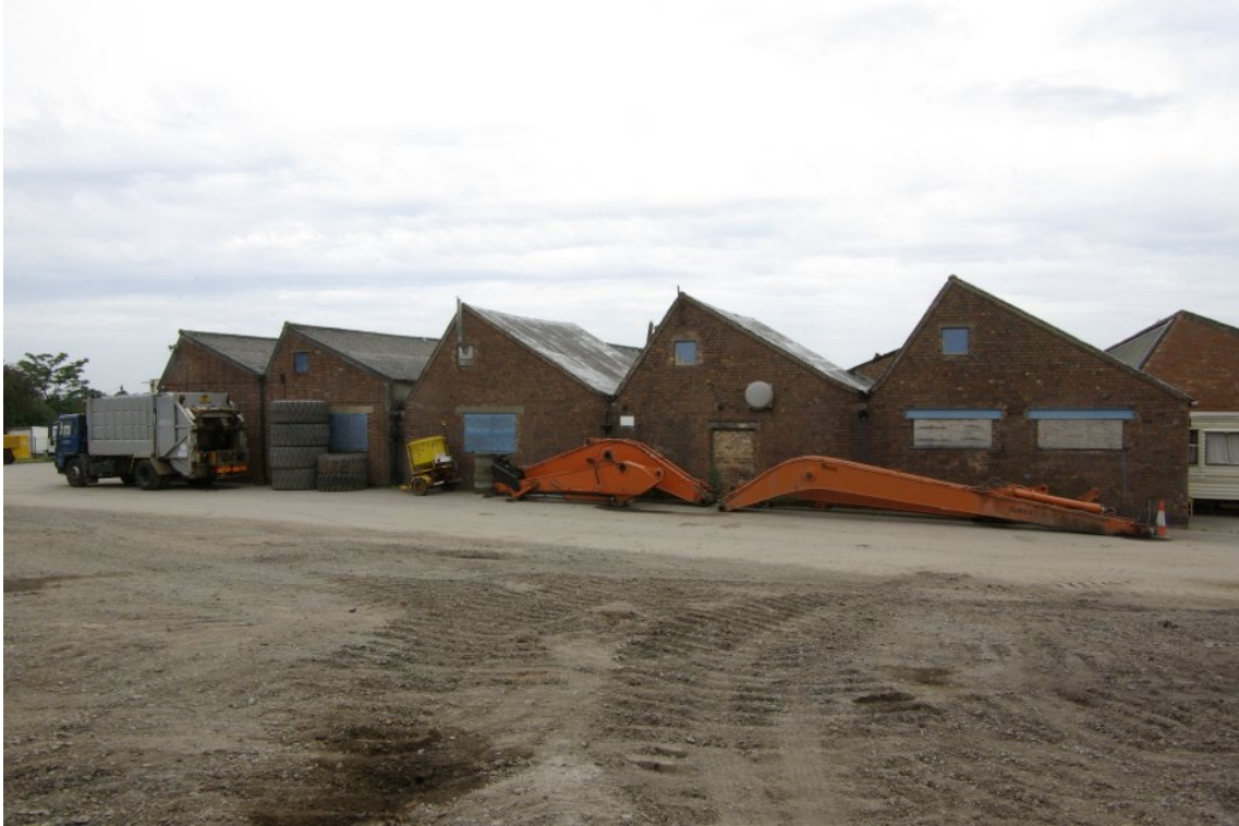
Figure 18 Building 3b, west facing elevation.
