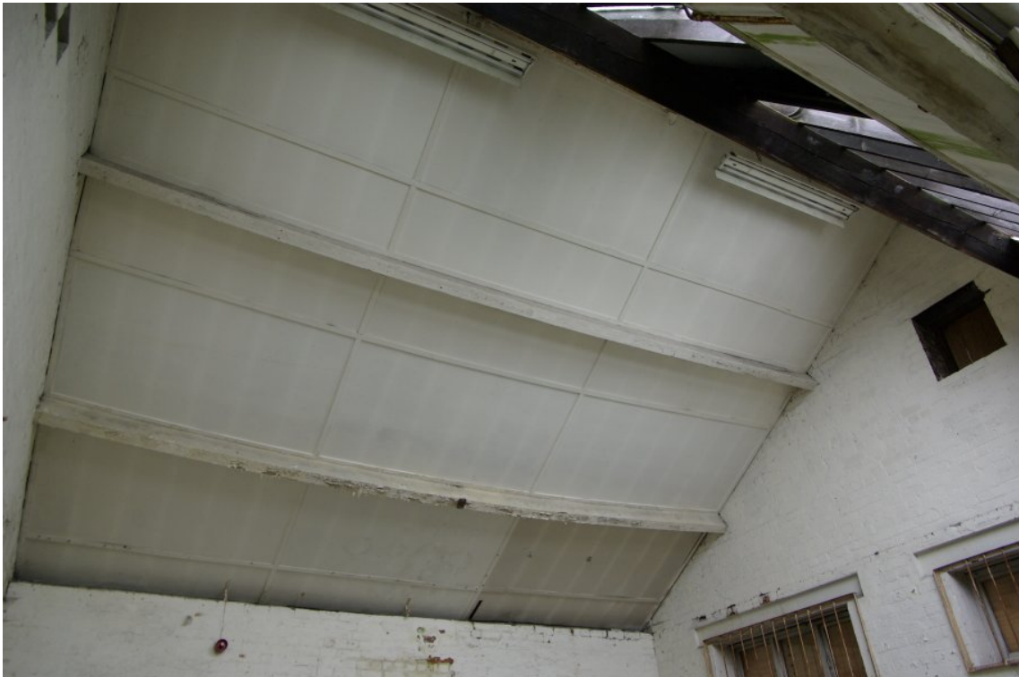
Figure 19 Roof construction within building 3b.
