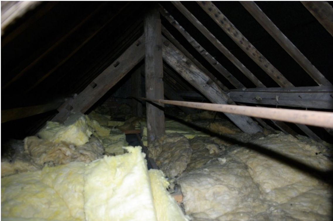
Figure 15 Roof truss within building 1b.
