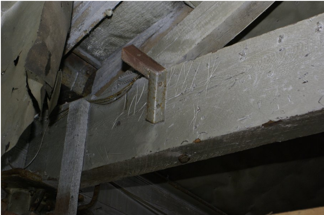
Figure 23 Rase marks on tie beam, building 4.
