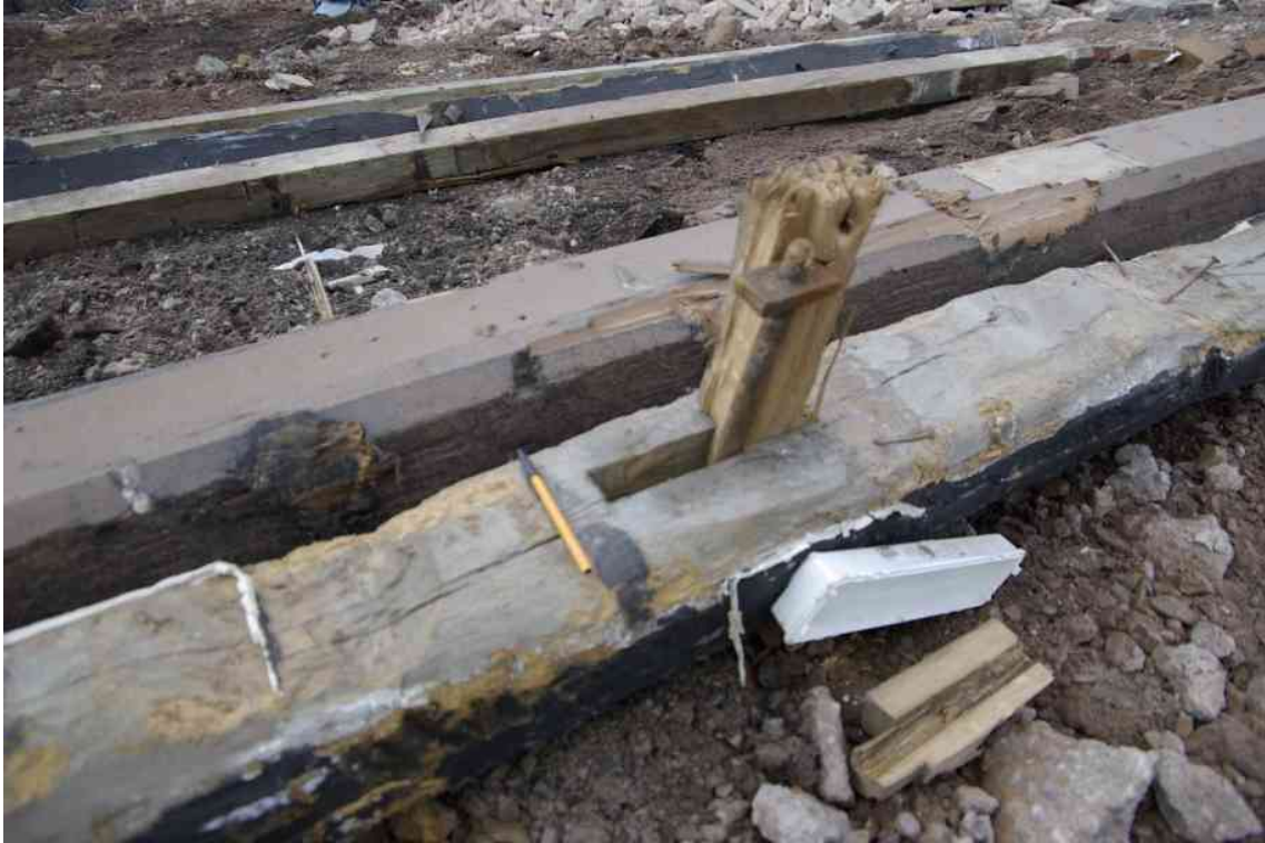
Figure 14 Tie beams from Building 1b after removal
