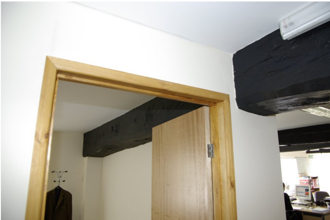
Figure 13 Tie beams visible within building 1b.
