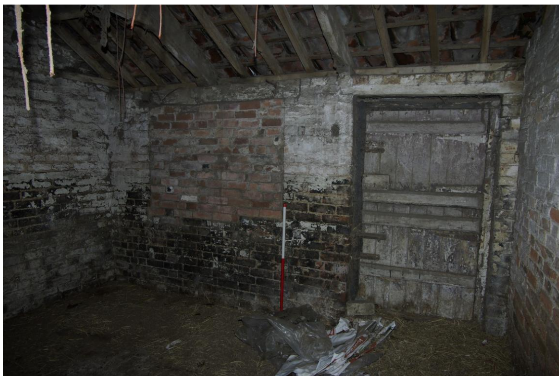
Figure 15. West building, north wall Looking north-west. 1m scale
