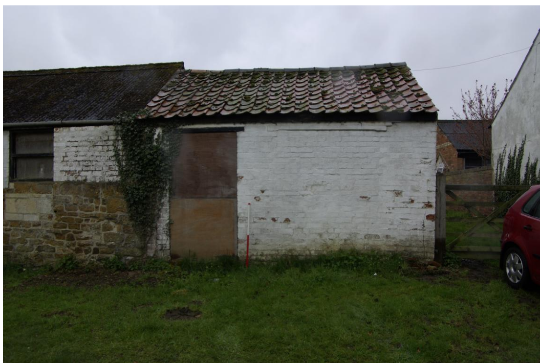
Figure 12. West building, north facing elevation Looking south. 1m scale
