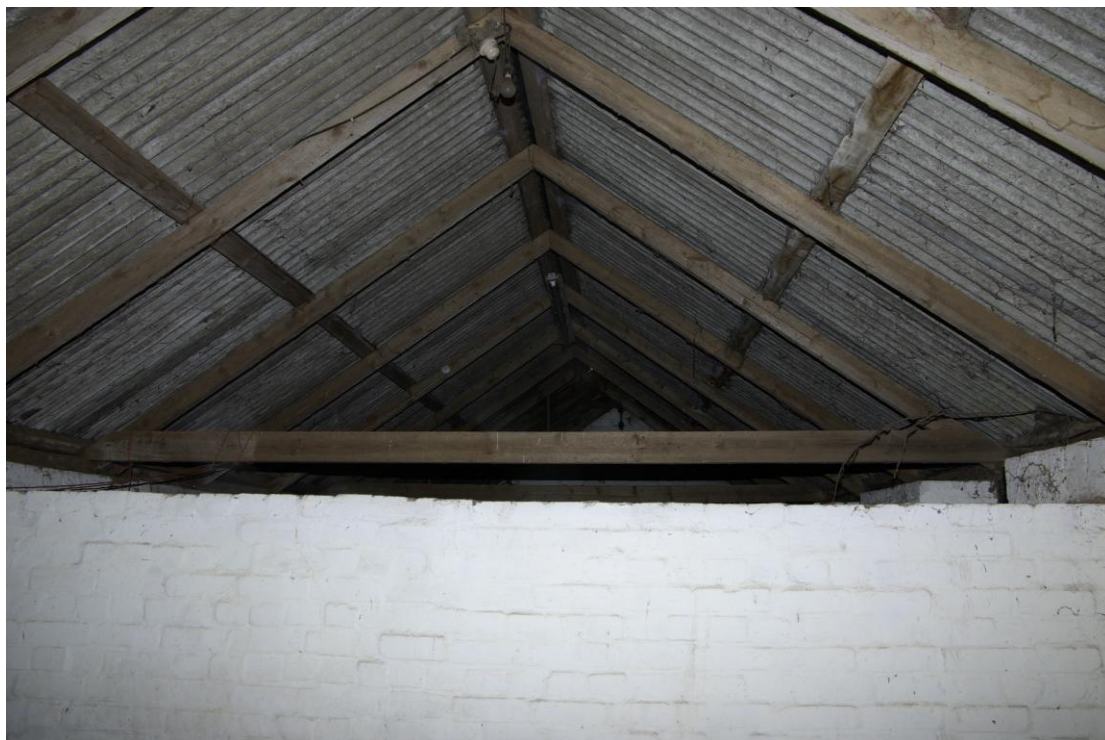
Figure 8. East building, roof and partition detail Looking west from eastern room
