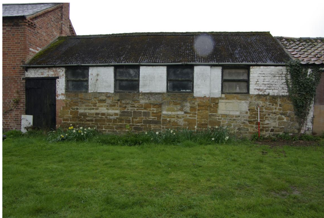
Figure 6. East building, north facing elevation Looking south. 1m scale
