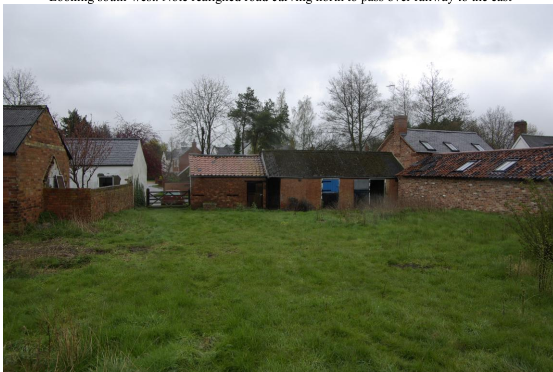
Figure 5. General view of site from rear of paddock Looking north
