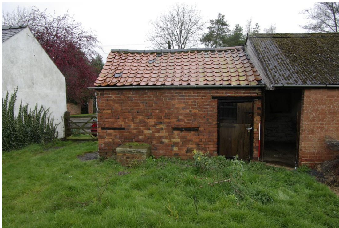
Figure 14. West building, south facing elevation Looking south. 1m scale
