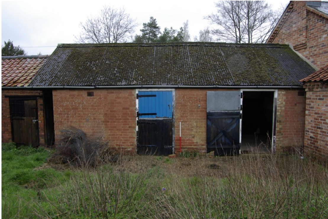
Figure 7. East building, south facing elevation Looking north. 1m scale
