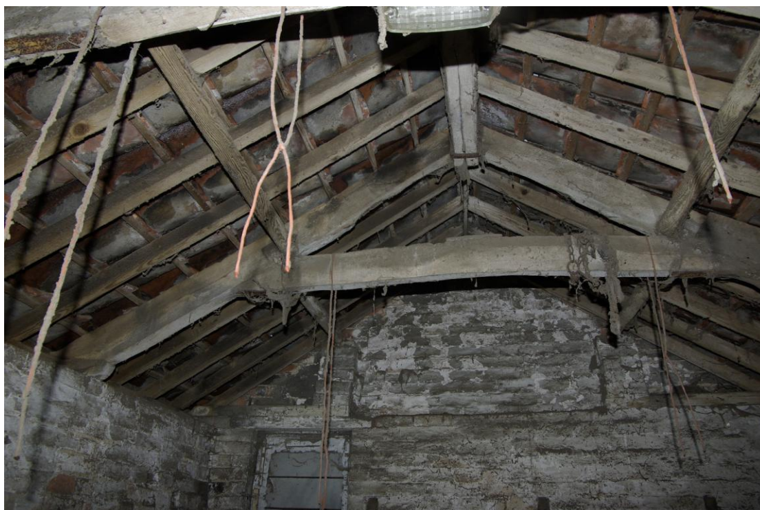
Figure 17. West building roof detail Looking west
