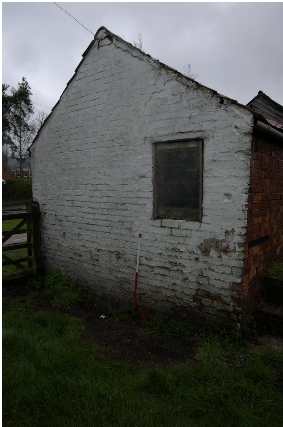
Figure 13. West gable end Looking north-east. 1m scale
