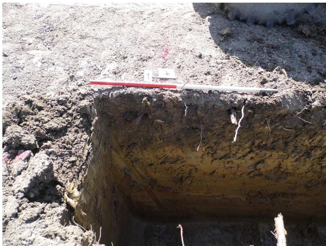
Figure 19. South-east section of garage foundation looking south
