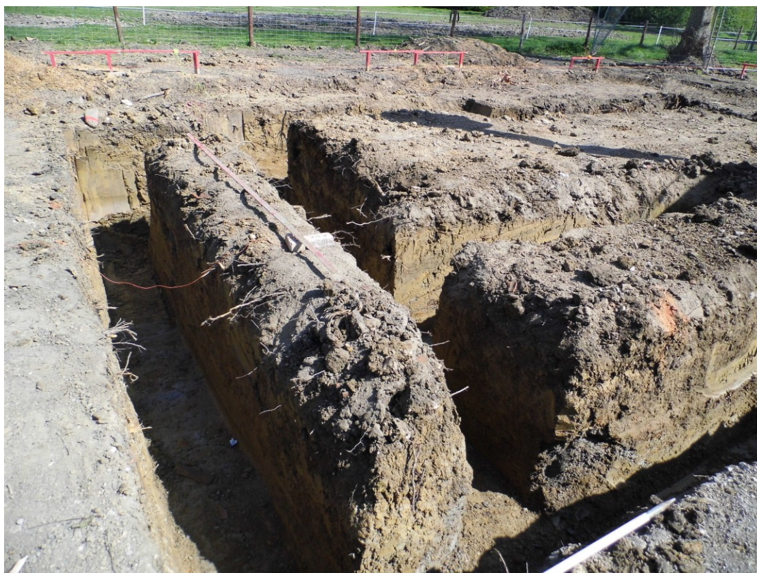
Figure 20. Foundations for the Workmans Cottage looking north-west
