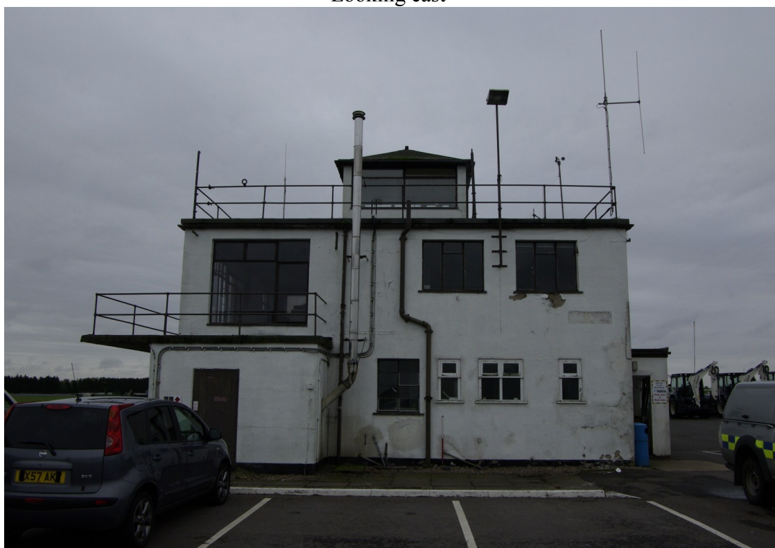
Figure 9. North-facing elevation Looking south. 1m scale
