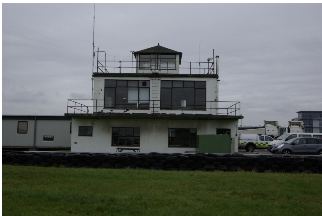
Figure 6. East facing elevation Looking west
