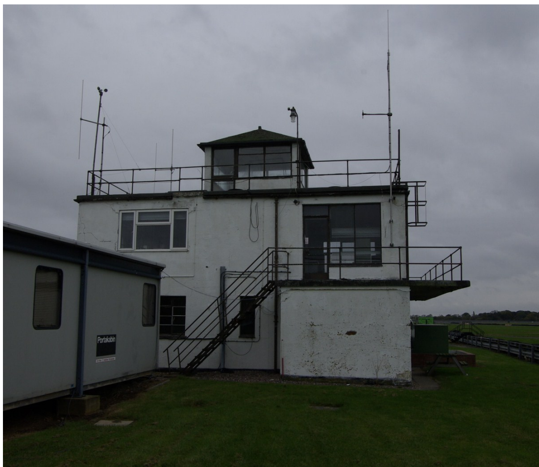
Figure 7. South facing elevation Looking north. 1m scale
