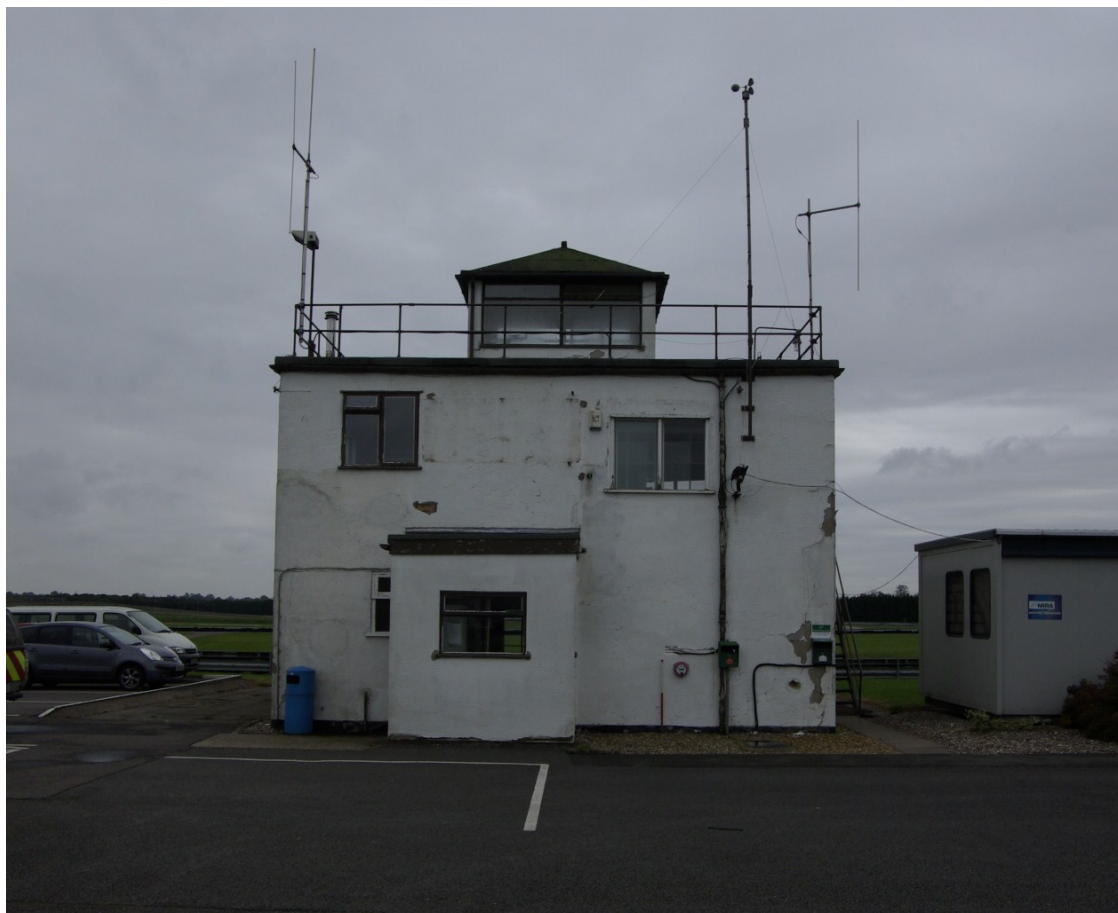
Figure 8. West facing elevation Looking east
