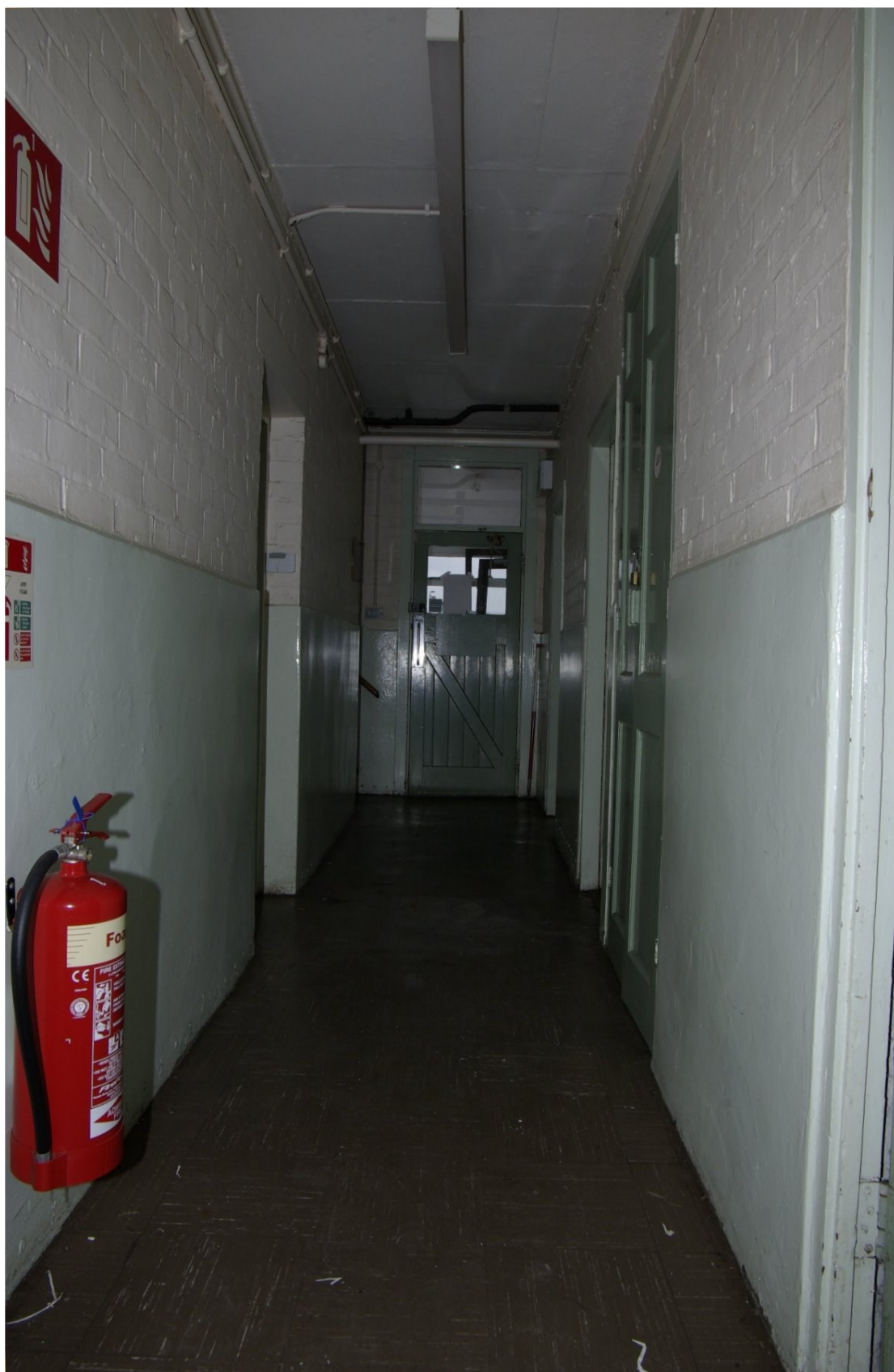
Figure 10. Ground floor corridor Looking west. 1m scale
