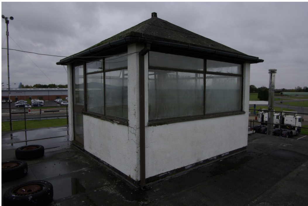
Figure 17. Visual control room. Looking north-east
