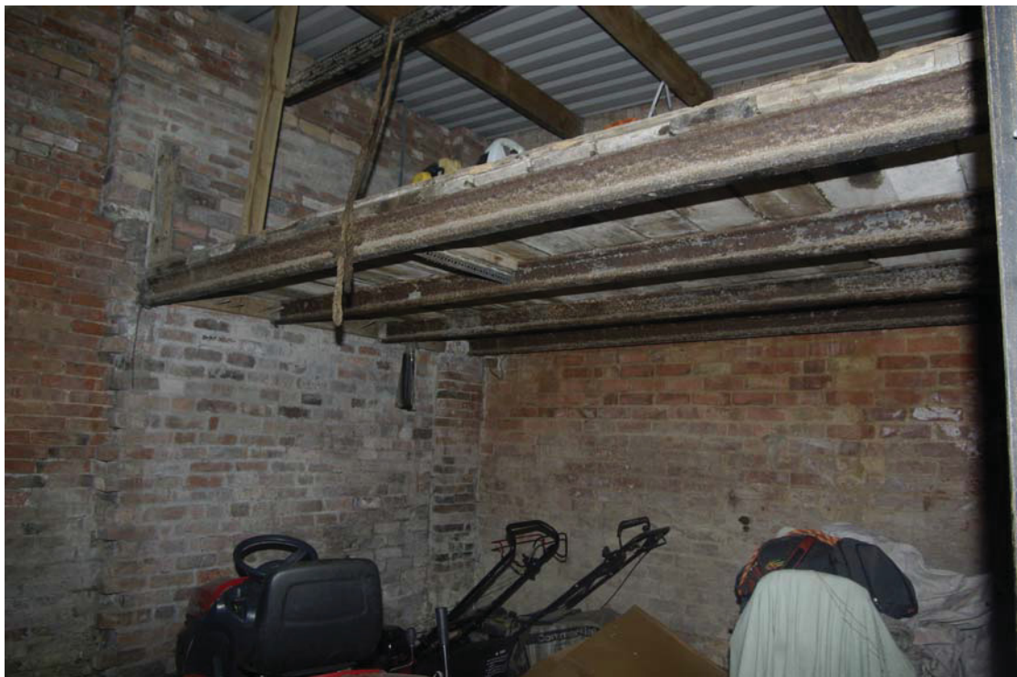
Figure 31. Building E interior, with inserted mezzanine floor, looking north-east.
