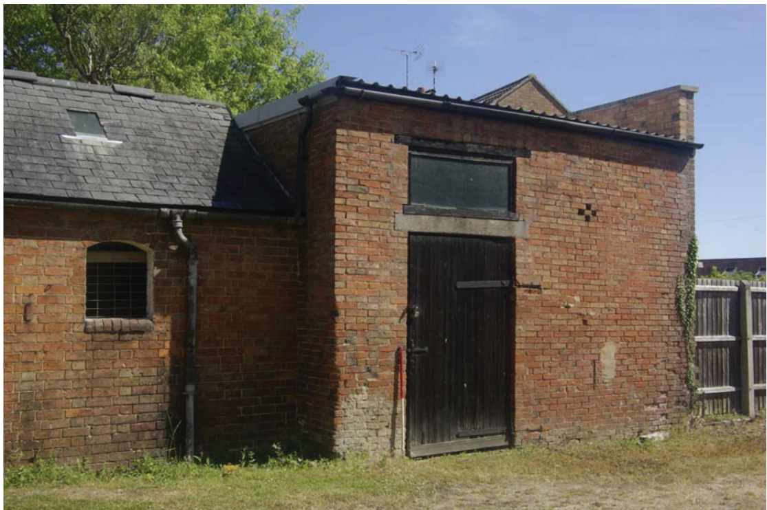
Figure 29. Building E, looking north-east.
