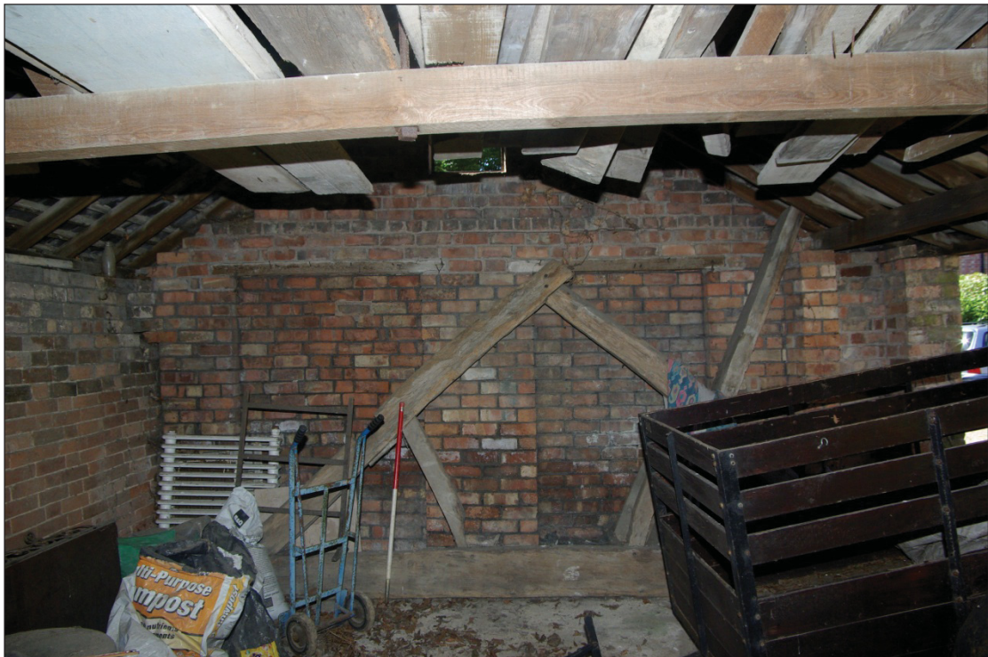
Figure 14. Building A, looking south (with roof truss removed from Building E).
