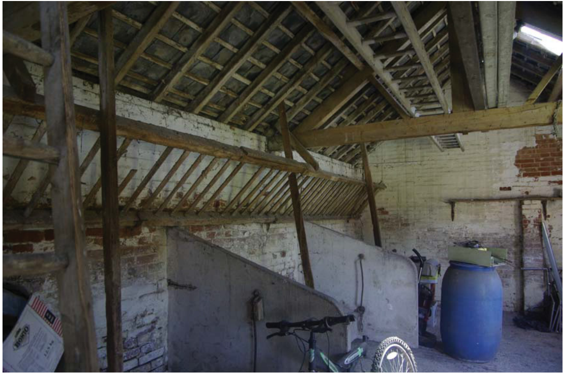
Figure 28. Building D interior, looking north-east.
