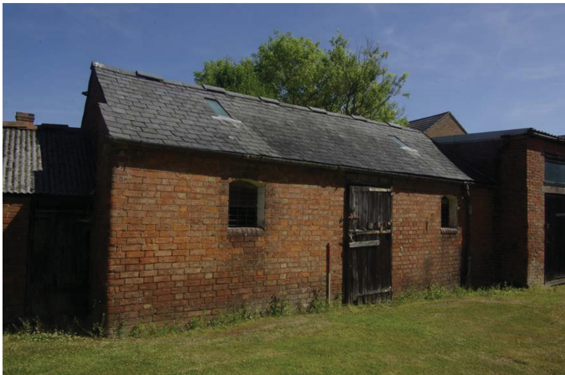
Figure 25. Building D, looking north-east.
