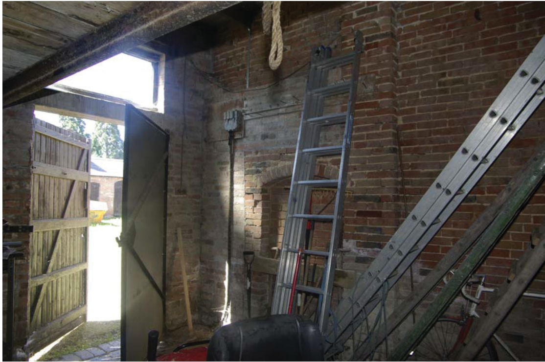
Figure 30. Building E, interior looking south-west.
