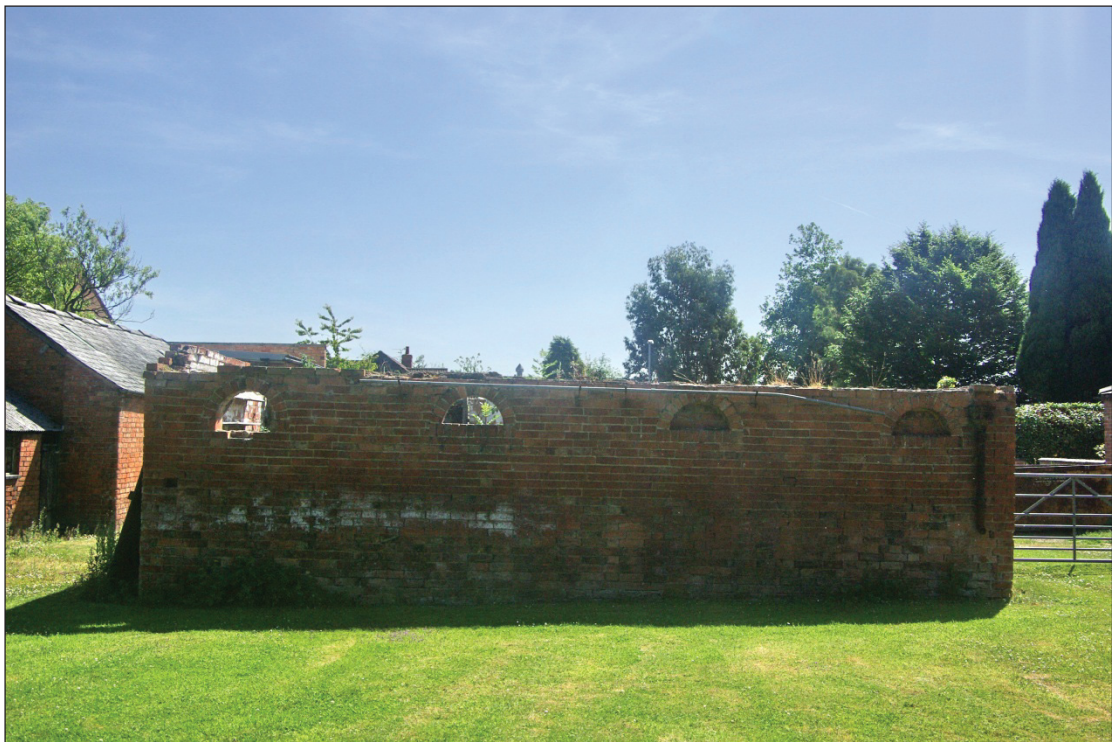
Figure 19. Rear elevation of Building B, looking east.
