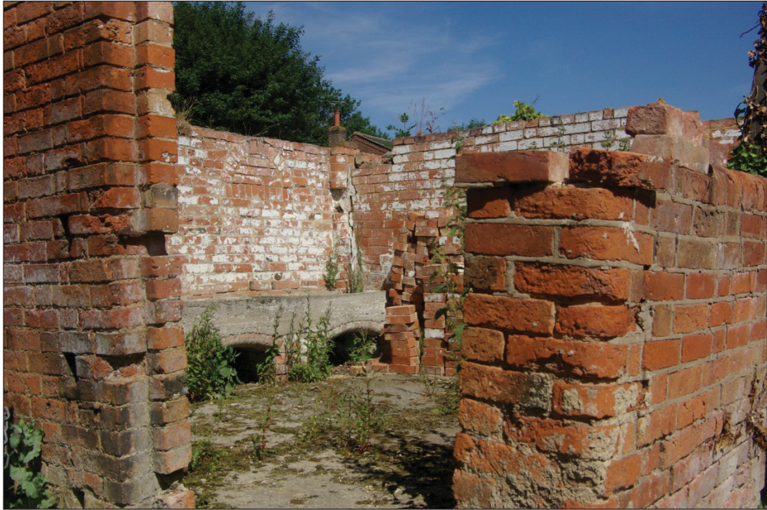
Figure 18. Building B interior, looking north-west.
