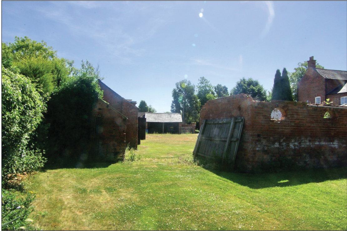
Figure 8. Looking east towards Building A.
