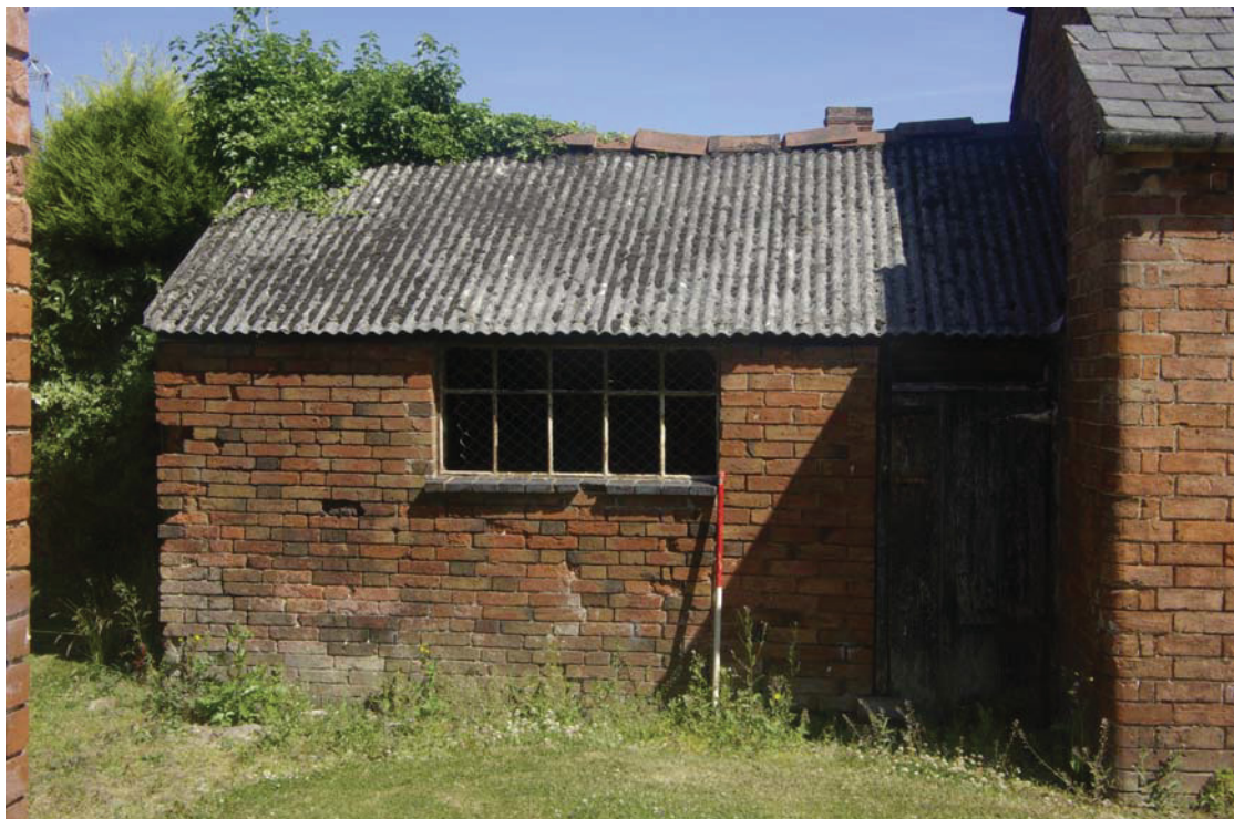
Figure 23. Building C, looking north.
