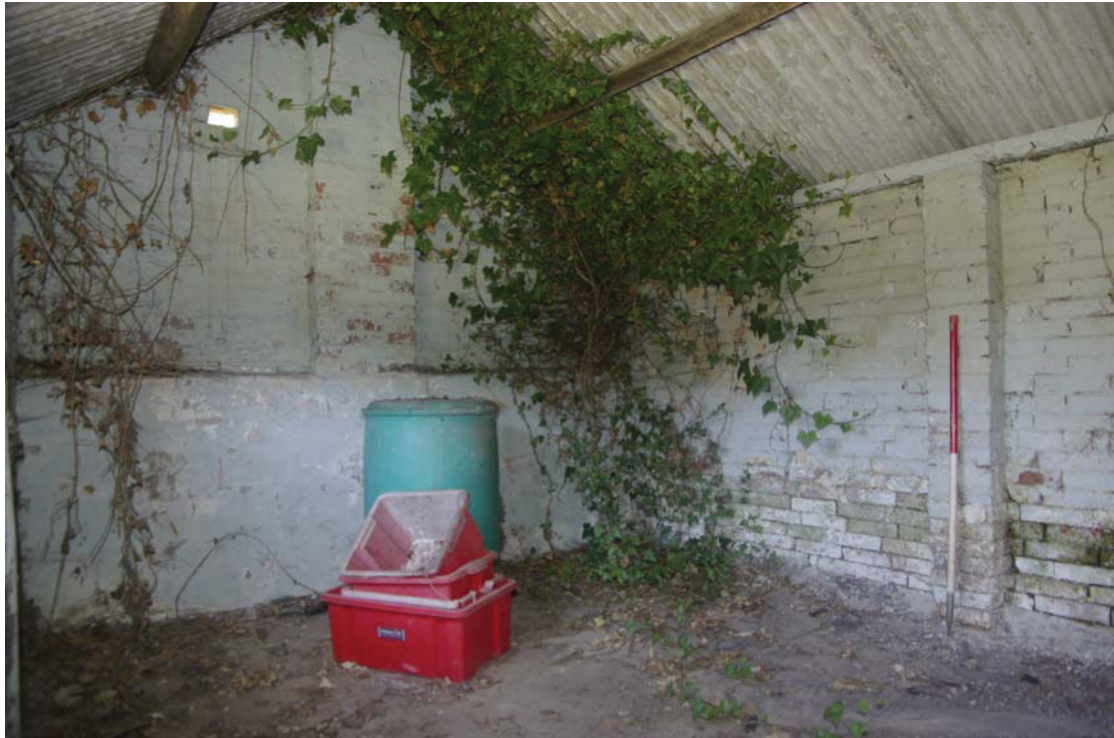
Figure 24. Building C, interior, looking north-west.
