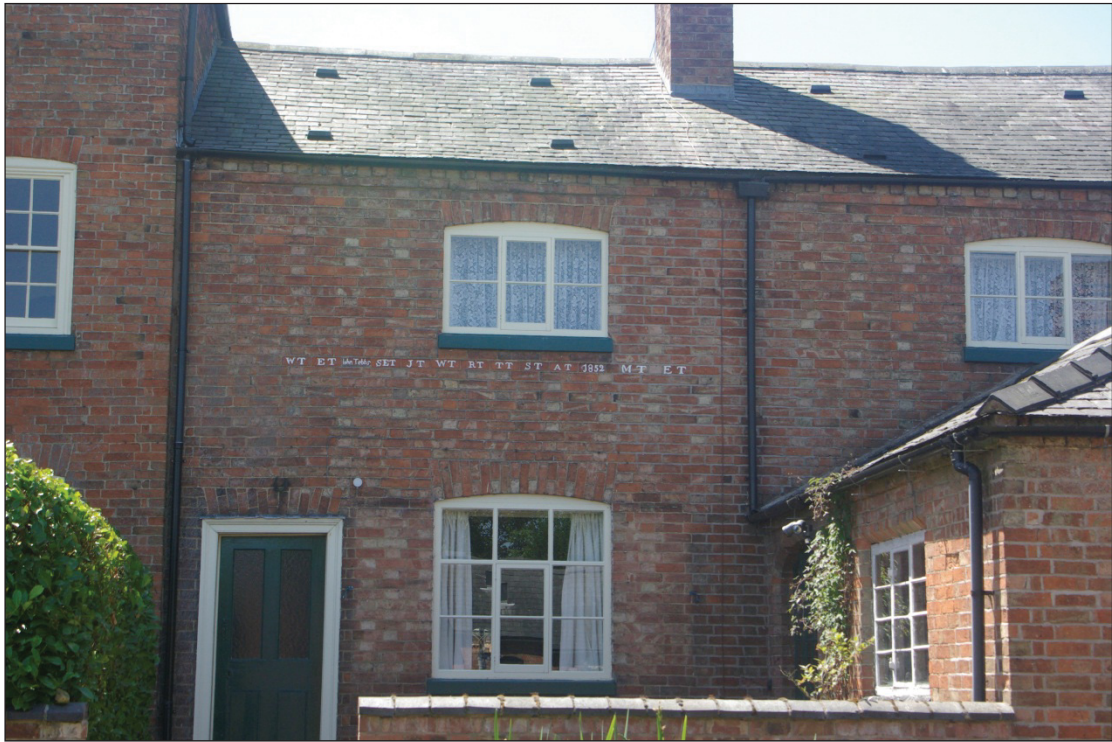
Figure 4. Dated initials on 19th century rear wing of farmhouse, looking south.
