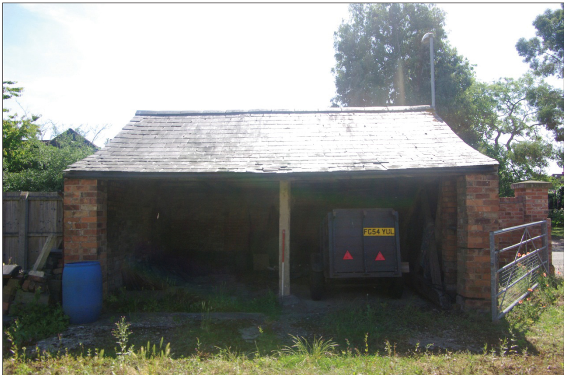
Figure 12. Building A, looking east.
