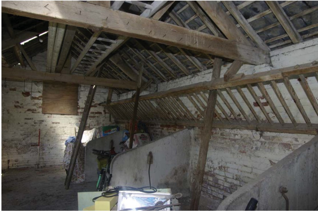
Figure 26. Building D, interior, with timber hayracks. Looking north-west.
