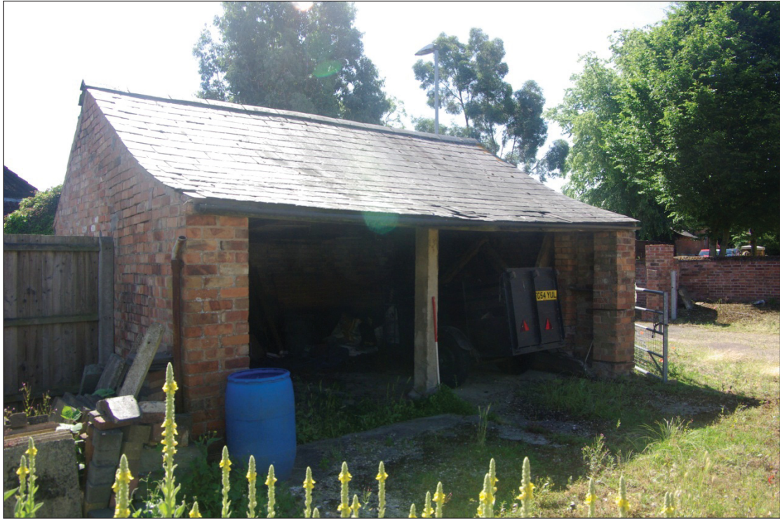
Figure 13. Building A, looking south-east.
