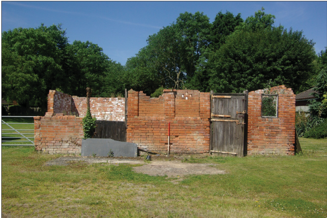
Figure 17. Building B, looking west.
