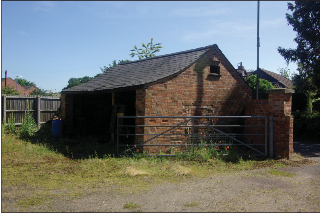
Figure 11. Building A, looking north-east.
