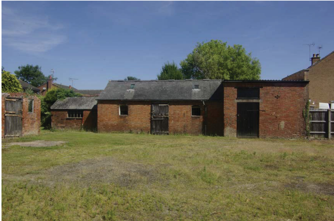
Figure 22. Building range C-E, looking north.
