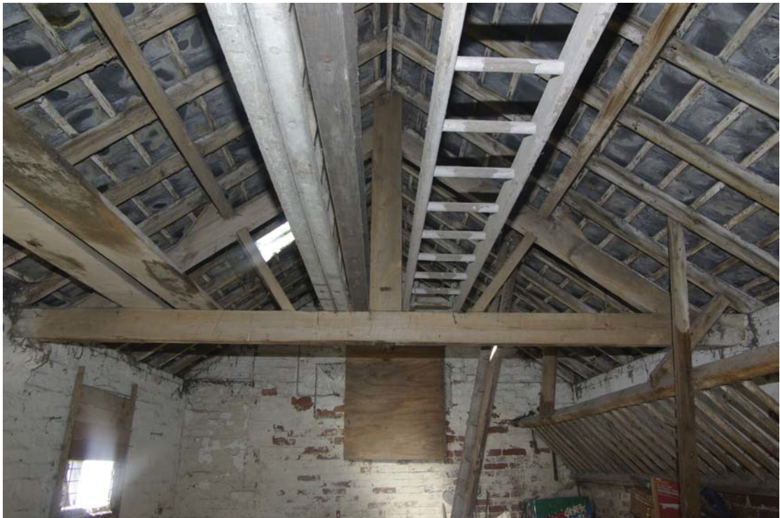
Figure 27. Building D, timber king-post roof truss, looking west.
