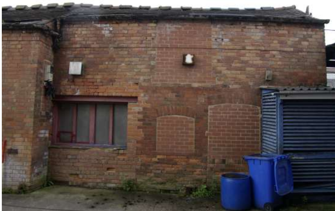
Figure 14. Blocked window and doorway openings in east-facing façade of slaughterhouse. Looking west.
