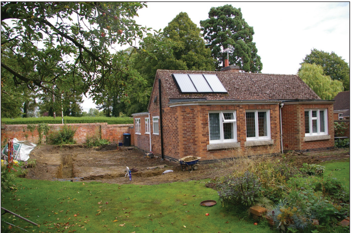
Figure 8. Stripped area, looking north.
