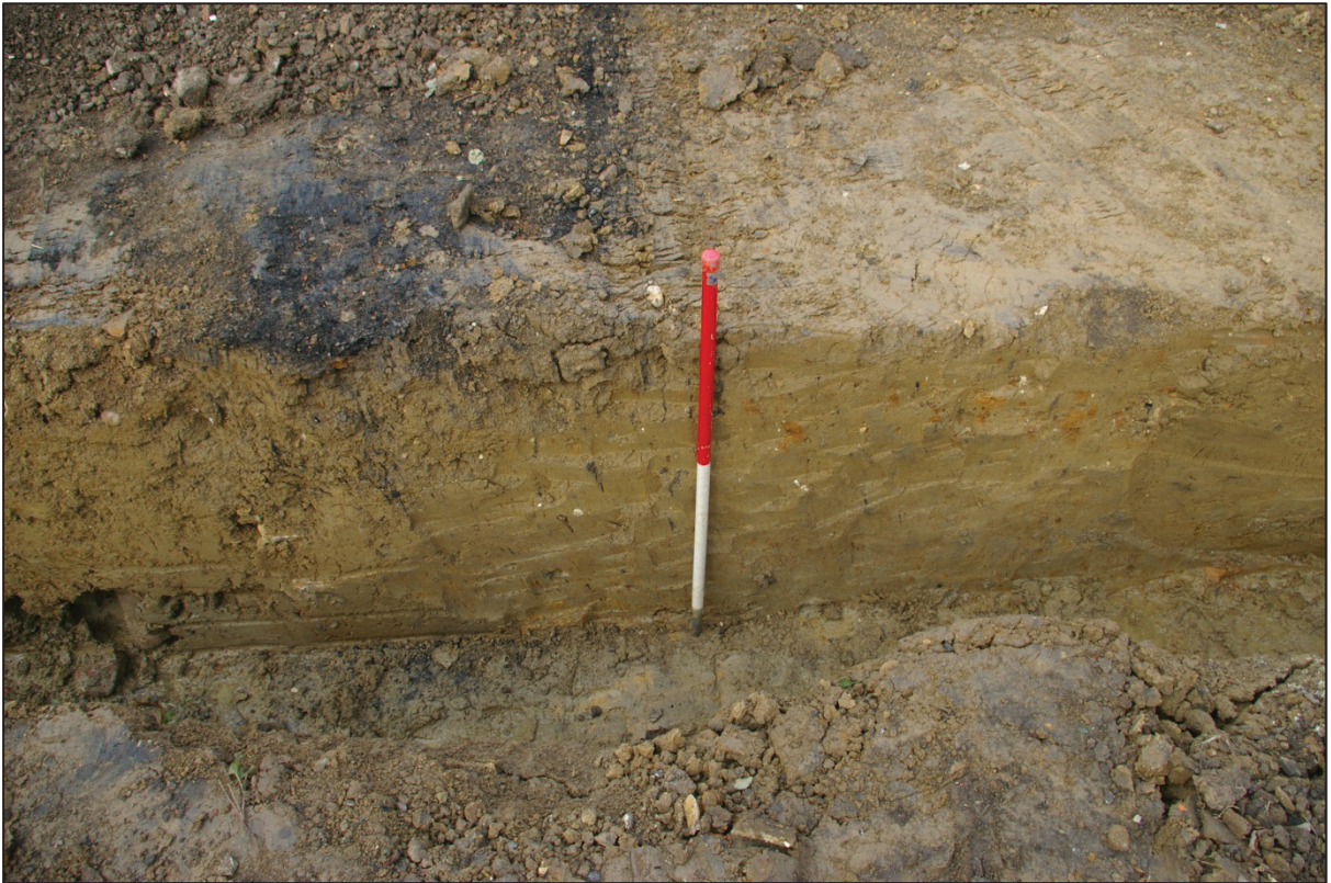
Figure 7. Example of foundation trench section, looking west.
