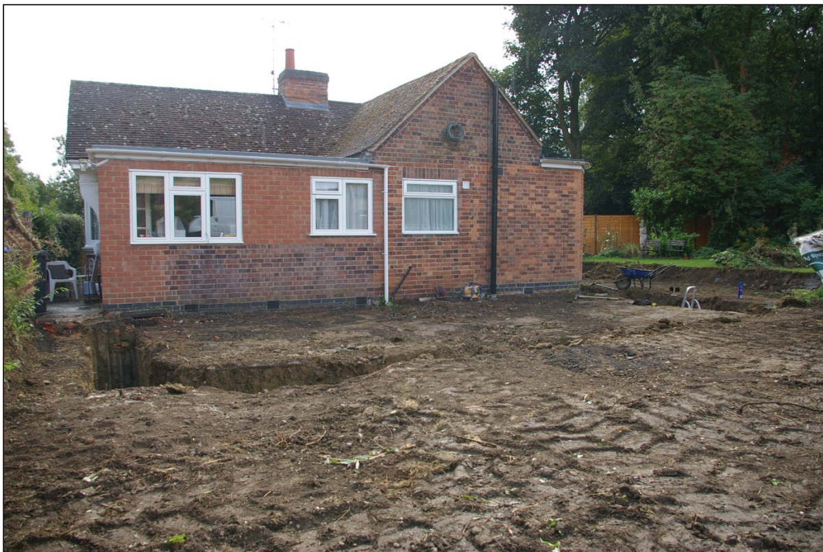
Figure 5. Stripped area, looking east.
