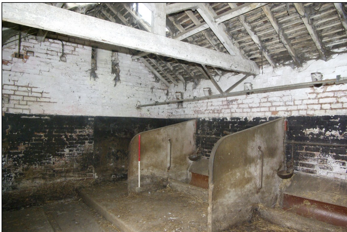
Figure 18. 20 th century concrete stall partitions with ceramic feeding troughs, looking south-west.
