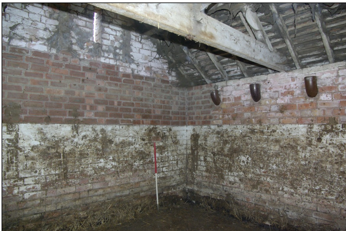
Figure 23. 1930s loose-box interior, with ceramic pipe ventilators, looking south-east.
