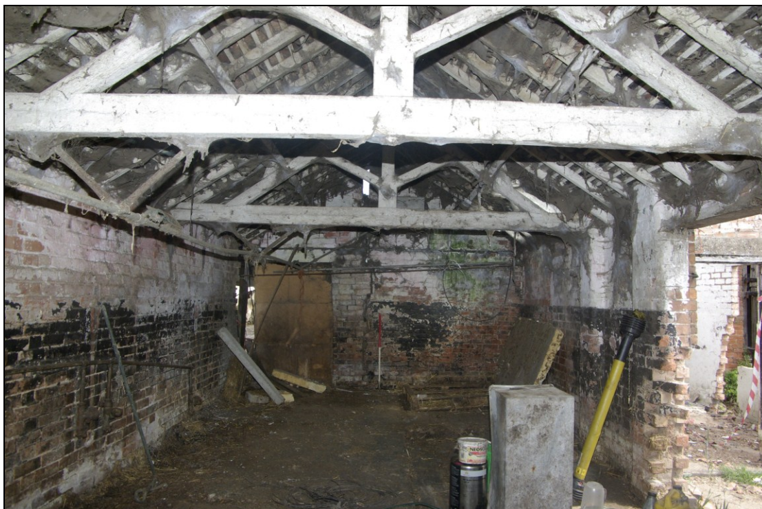
Figure 16. Cow-shed interior, looking north.
