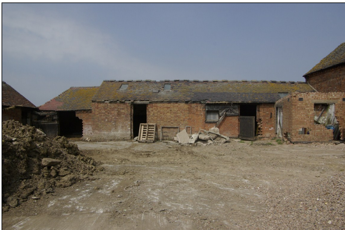
Figure 15. Cow-shed, with rebuilt east-facing wall. Looking west.
