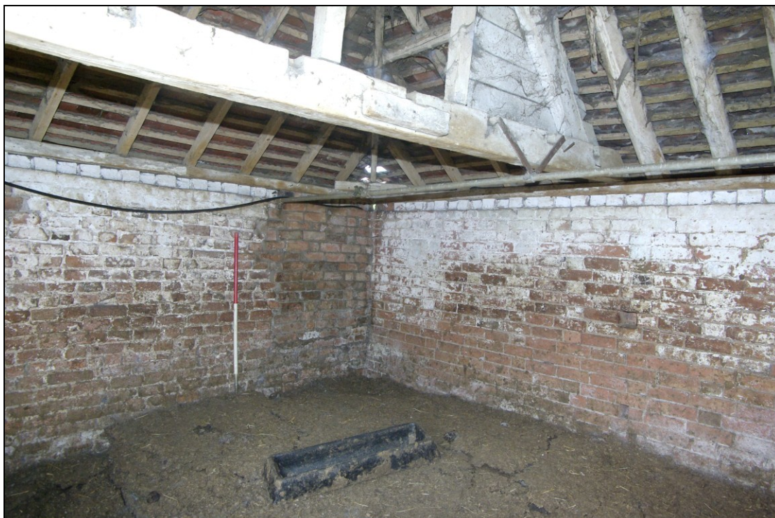
Figure 20. Loose-box interior, looking west.
