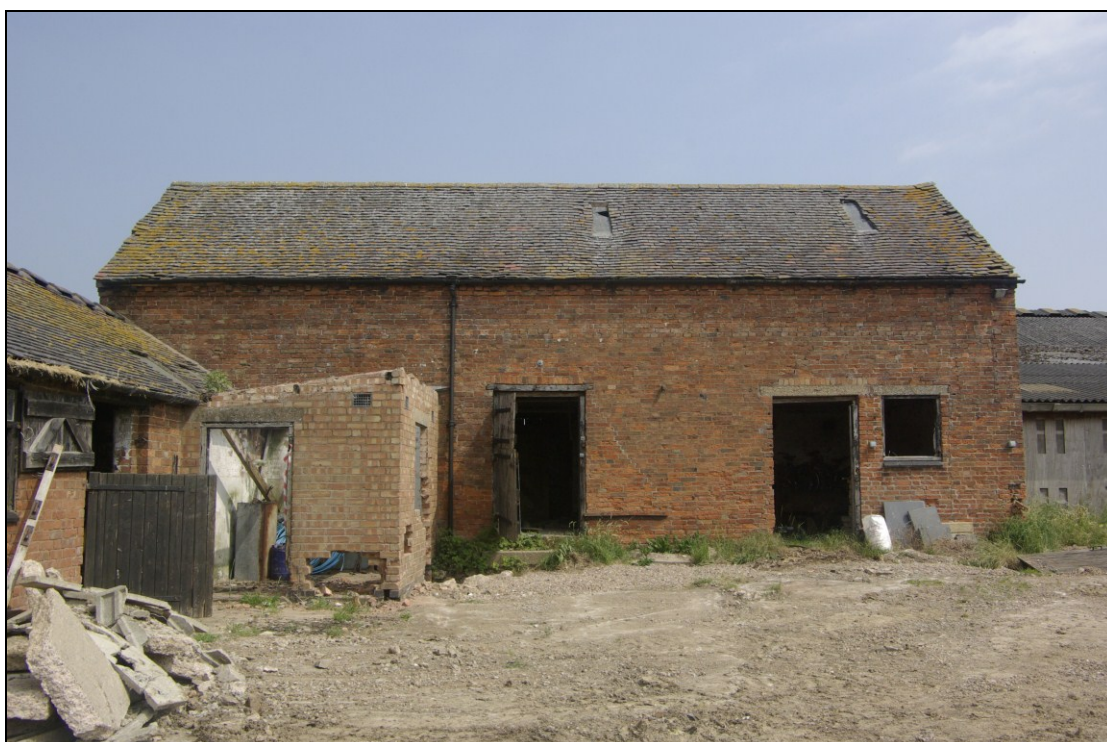
Figure 9. Barn, looking north.
