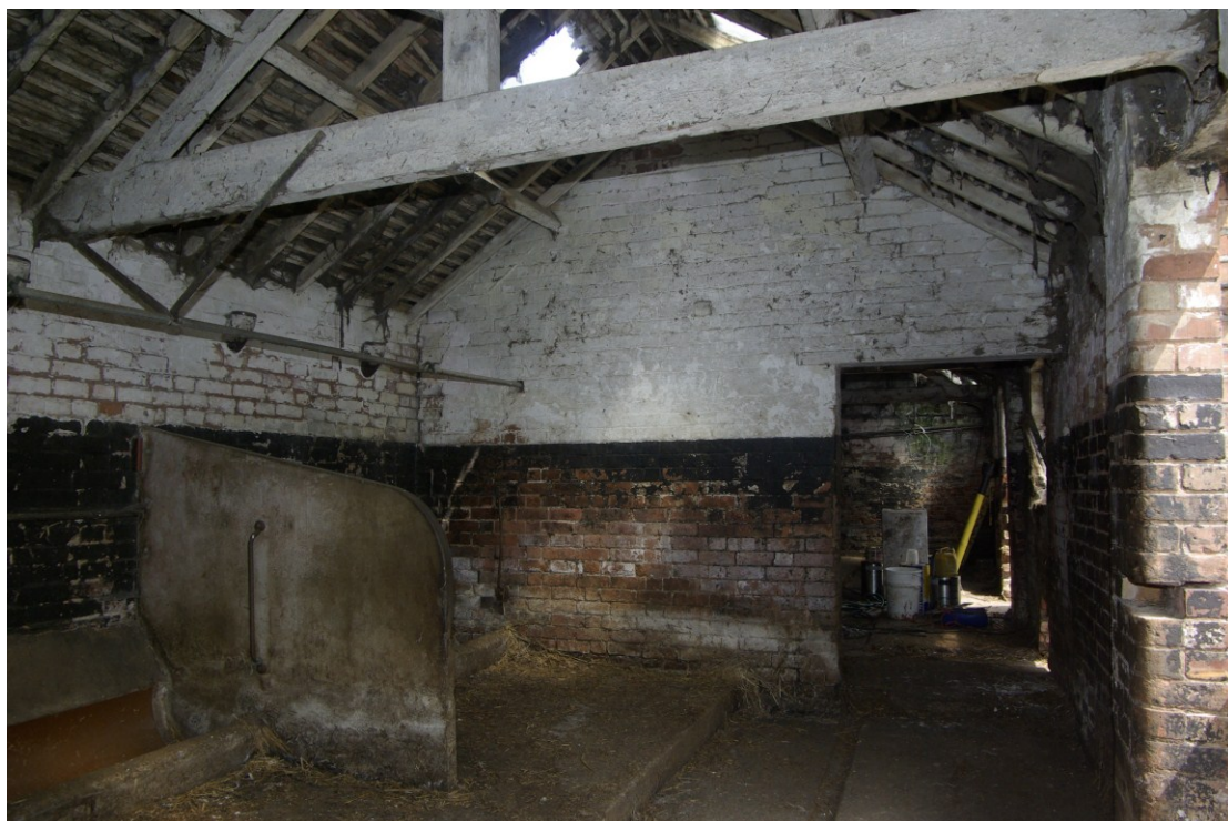
Figure 17. Cow-shed interior, looking north.
