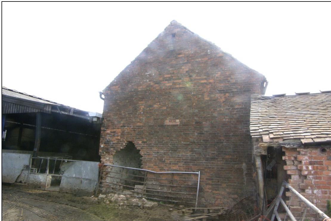
Figure 14. Western gable-end wall of Barn, looking east.
