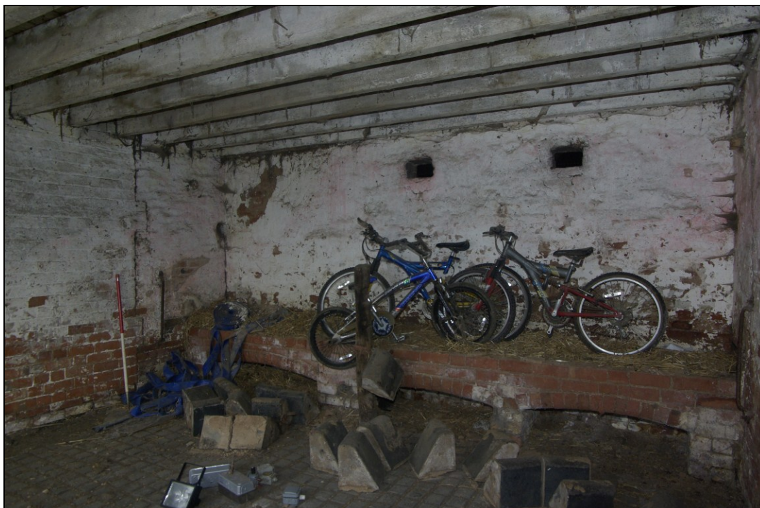
Figure 10. Eastern end bay of Barn, with brick-arch troughs. Looking north.
