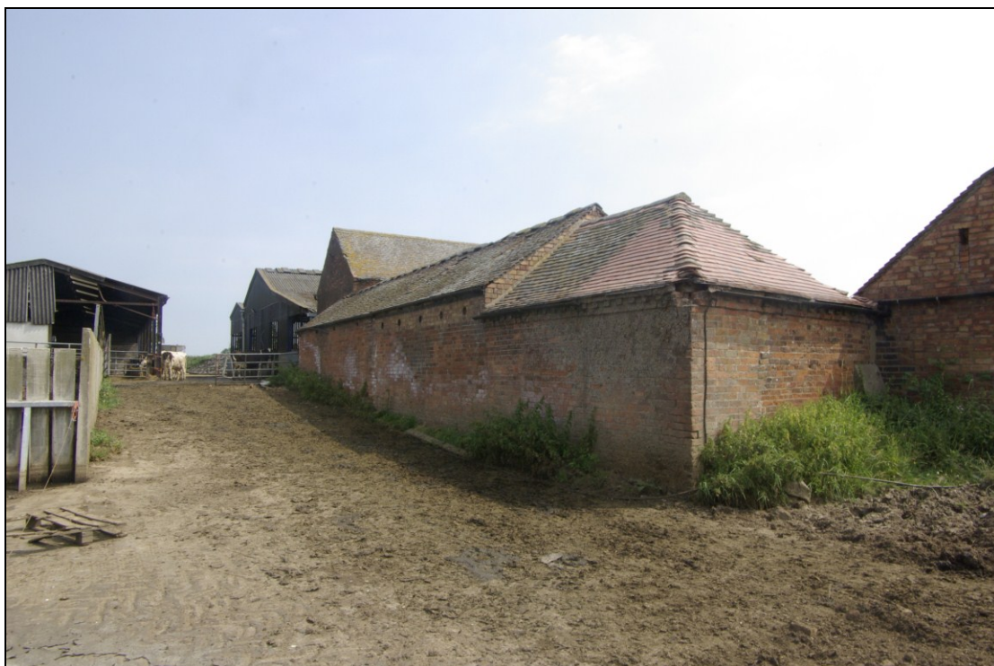
Figure 21. Rear elevation of cow-shed, showing raised line of eaves. Looking north-east.
