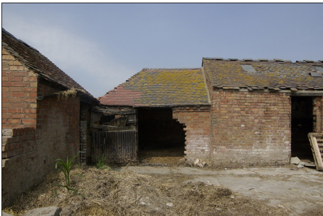
Figure 19. Loose-box at southern end of cow-shed. Looking west.
