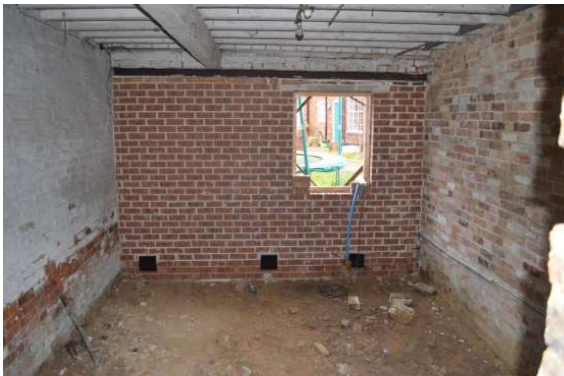
Figure 23 Ground floor, east room Looking south
