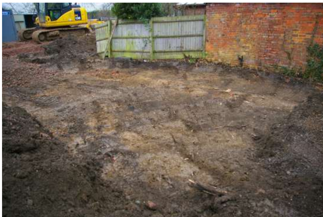
Figure 7 Stripped drive Looking south west
