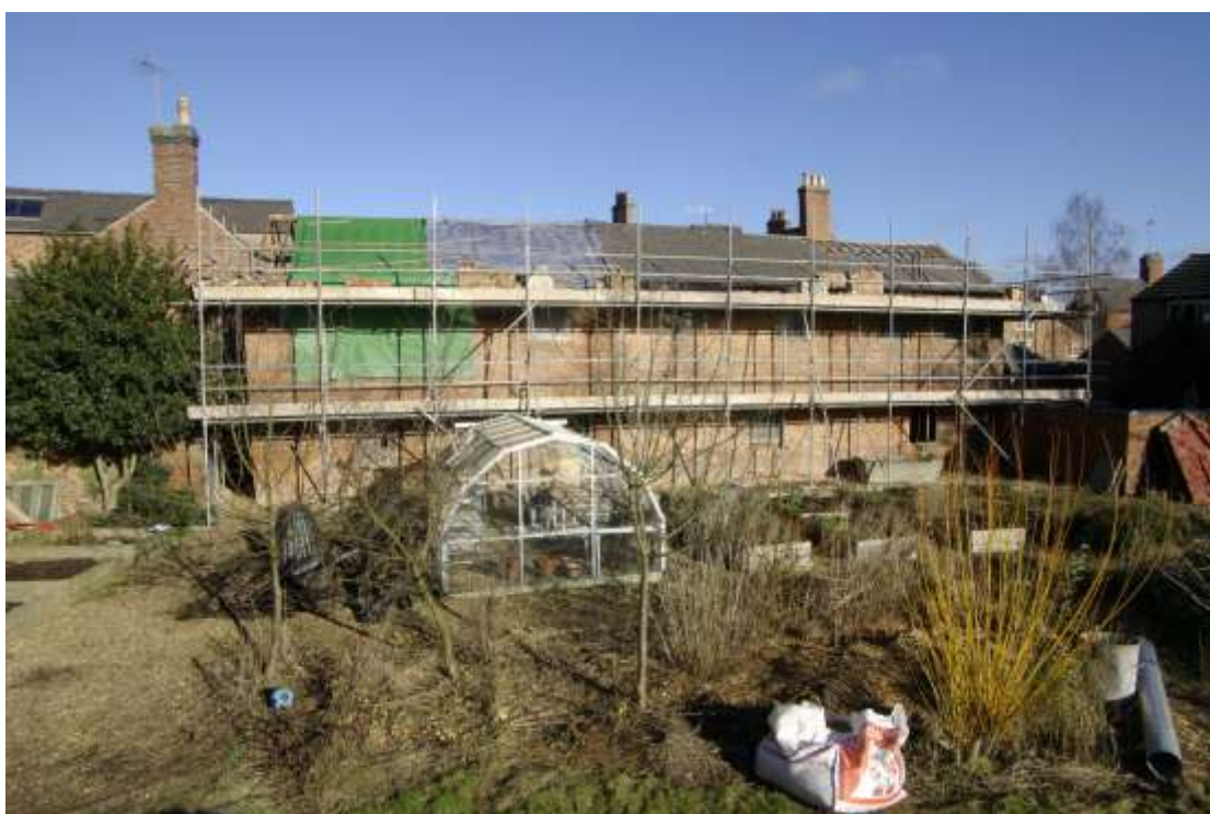
Figure 14 South facing elevation Looking north east
