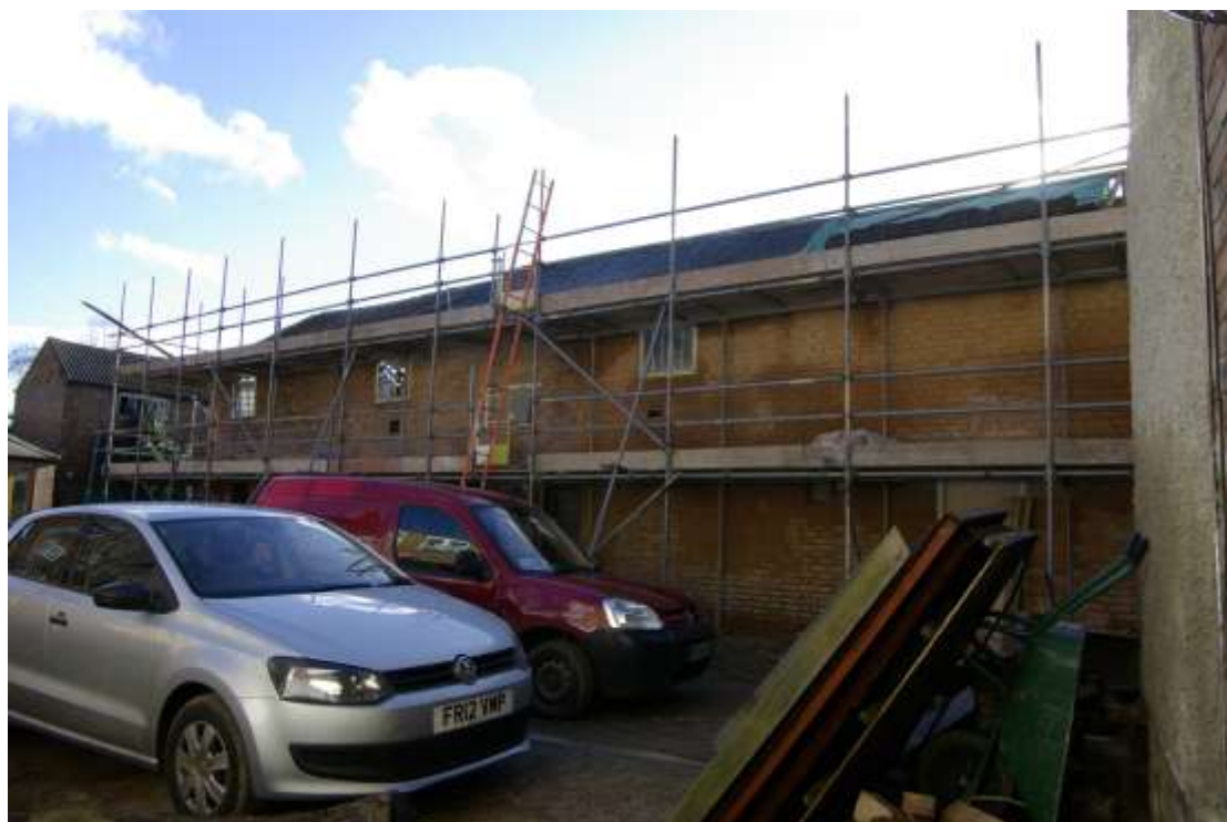
Figure 8 North facing elevation Looking south east
