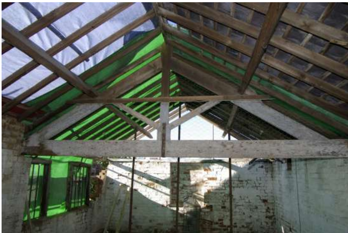
Figure 27 First-floor roof truss Looking west
