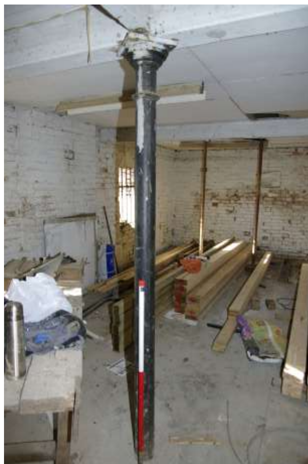
Figure 19 Ground floor, west room, post detail Looking south west, 1m scale
