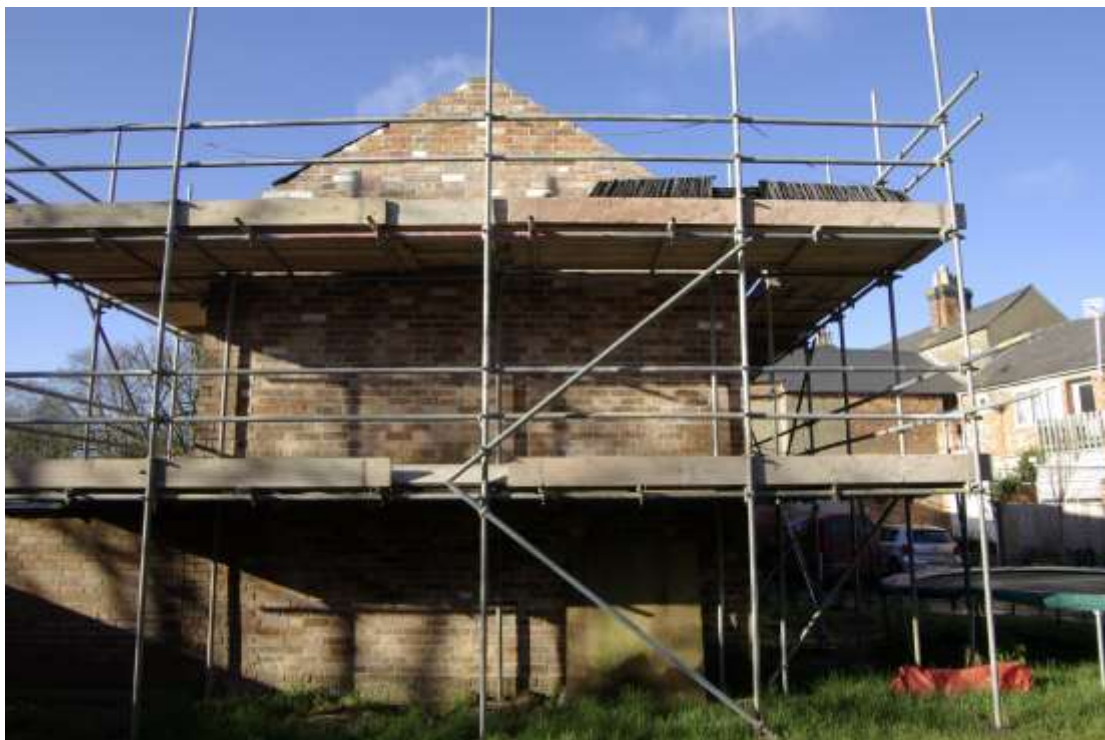
Figure 13 East-facing elevation Looking west
