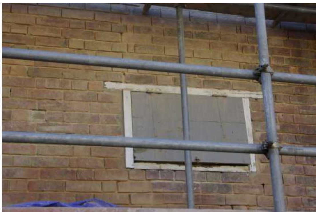
Figure 12 Modified window on north facing elevation Looking south west
