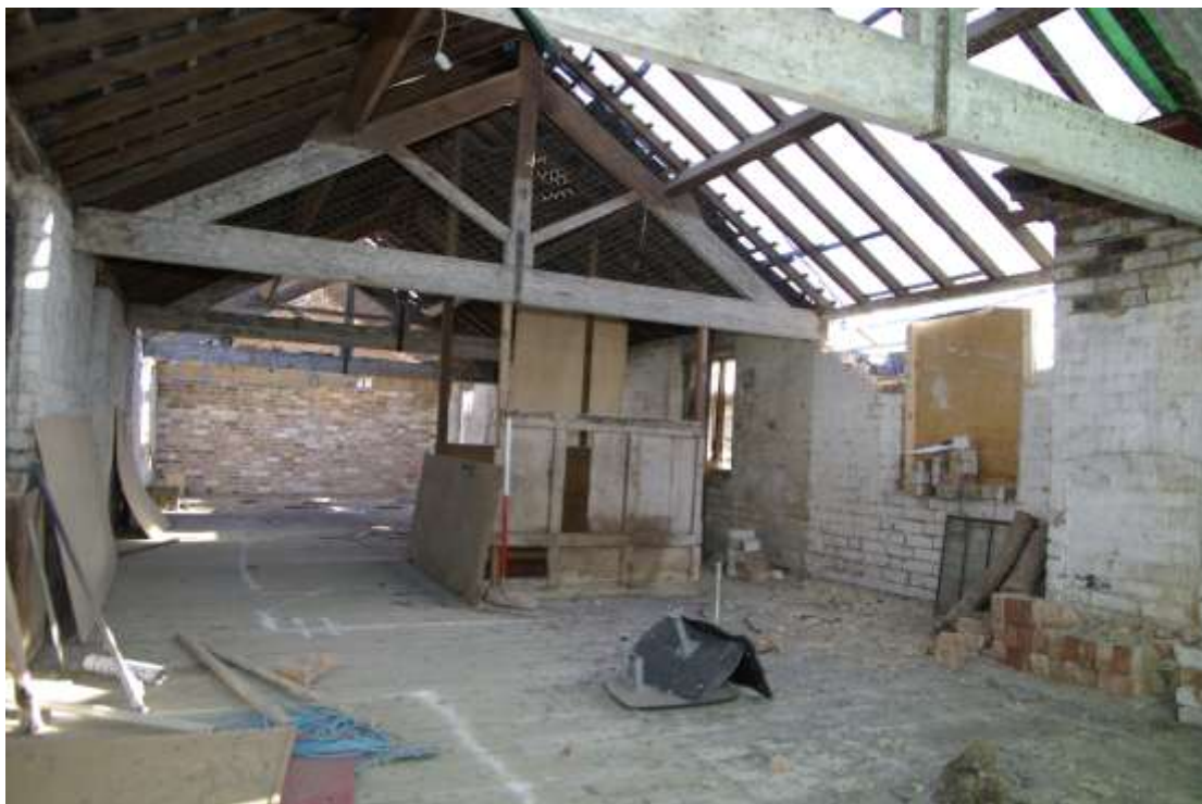
Figure 25 First floor Looking south east, 1m scale
