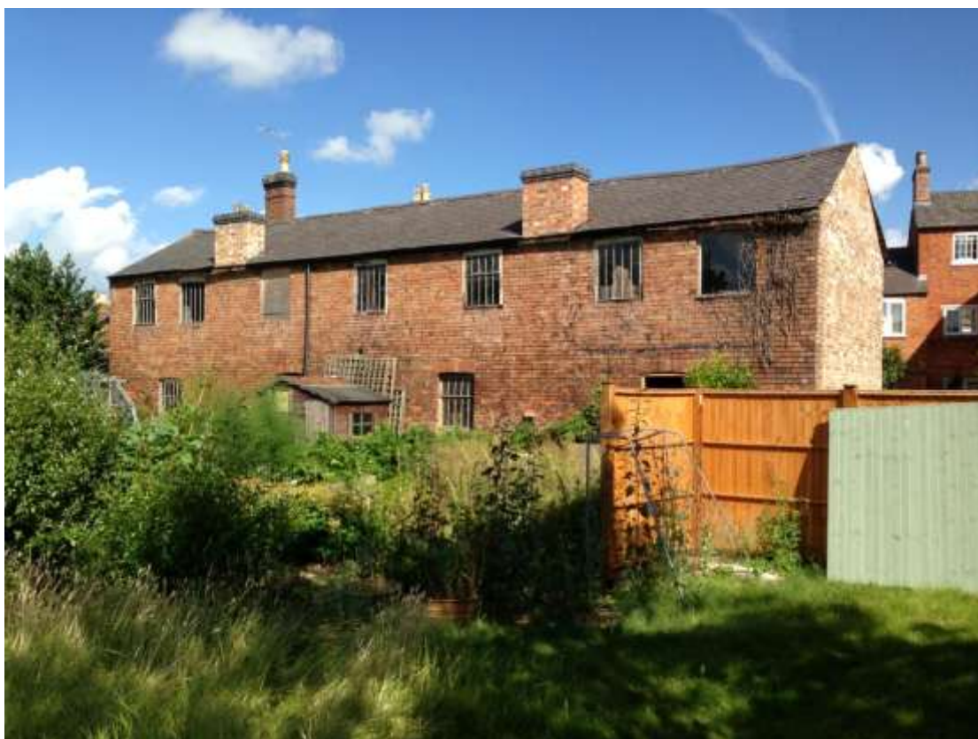
Figure 16 South-facing elevation Photograph taken by Mr R Gamble prior to remedial works.
