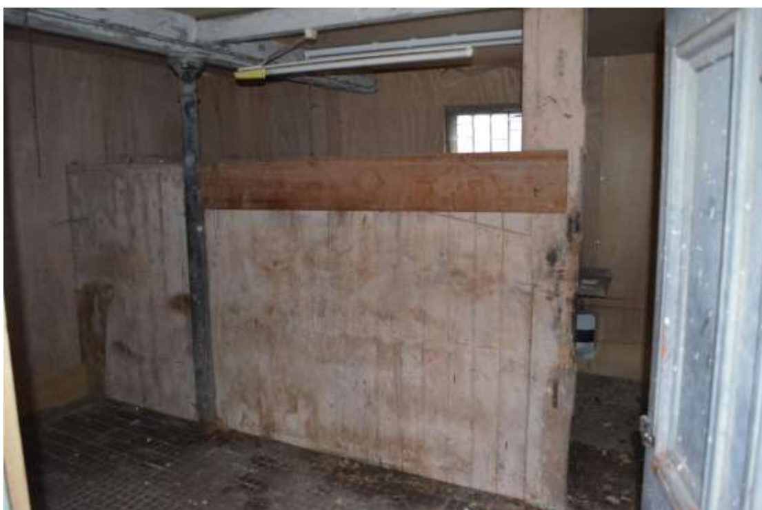
Figure 21 Ground floor, middle room Looking south east
