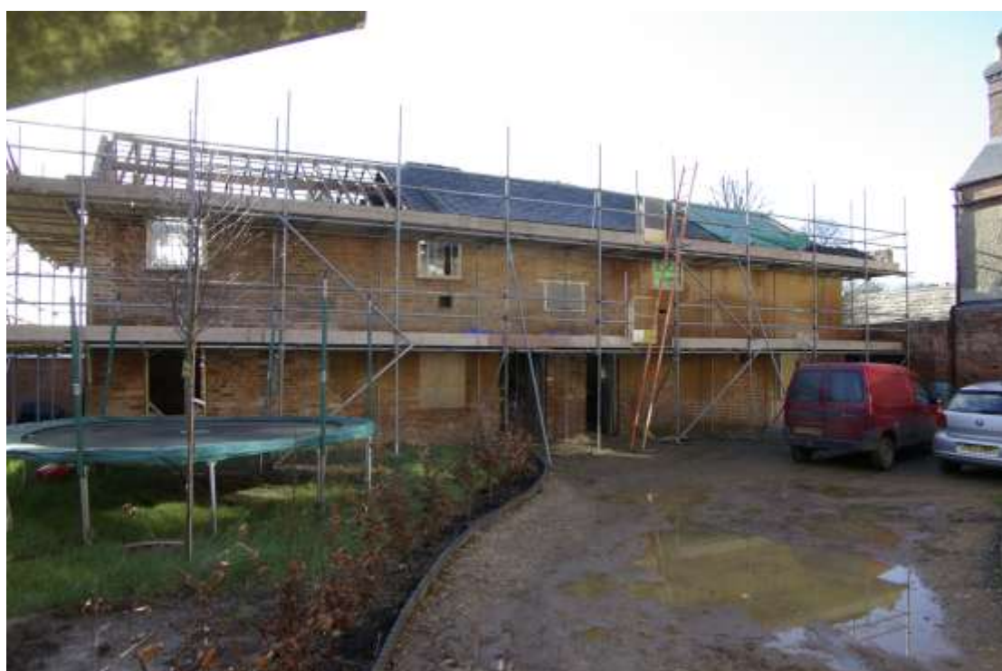
Figure 9 North facing elevation Facing south west
