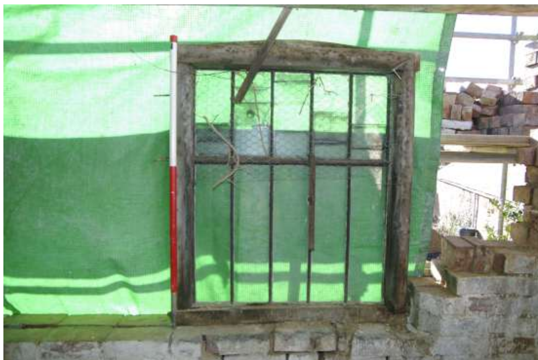
Figure 17 South-facing elevation first floor window Looking south, 1 m scale
