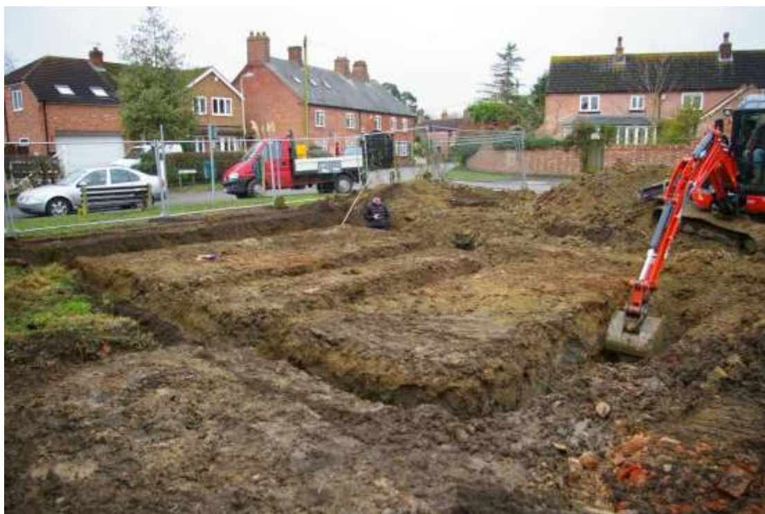
Figure 5 Foundation trenches Looking south west
