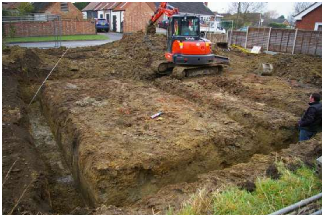
Figure 4 Partially excavated foundation trenches Looking north west
