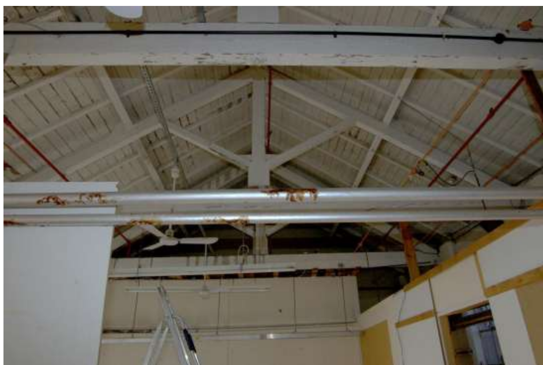
Figure 19. Building A, first floor, with modern office partitions and king-post roof structure. Looking west.
