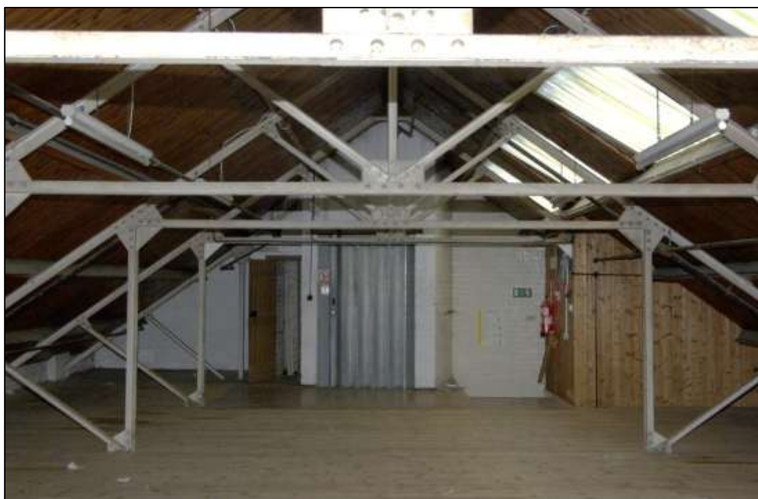
Figure 25. Building D, loft storage, with steel roof trusses. Looking north towards lift shaft.
