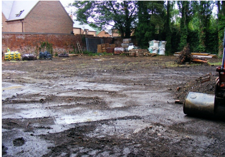
Figure 4: Looking northeast over the ground surface after the site strip
