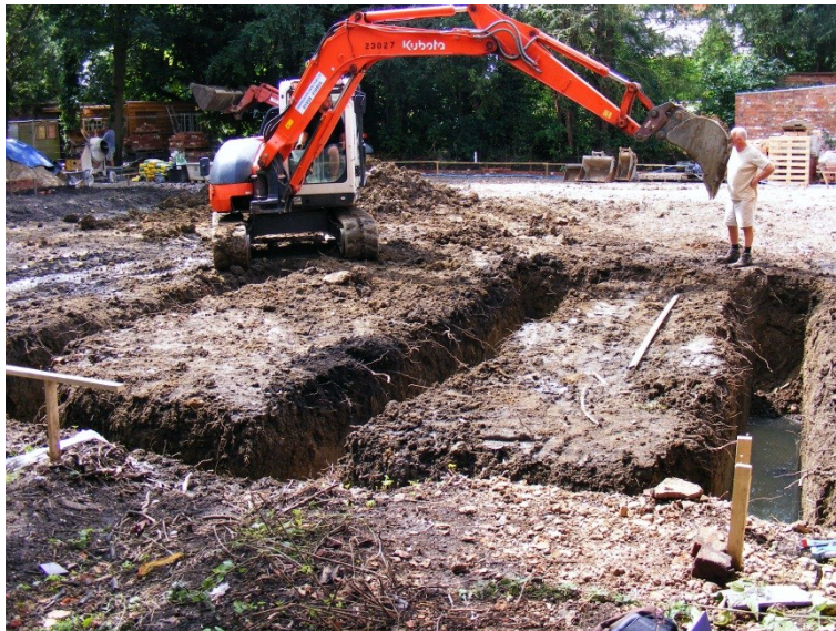
Figure 5: Looking west during the excavation of the foundation trenches
