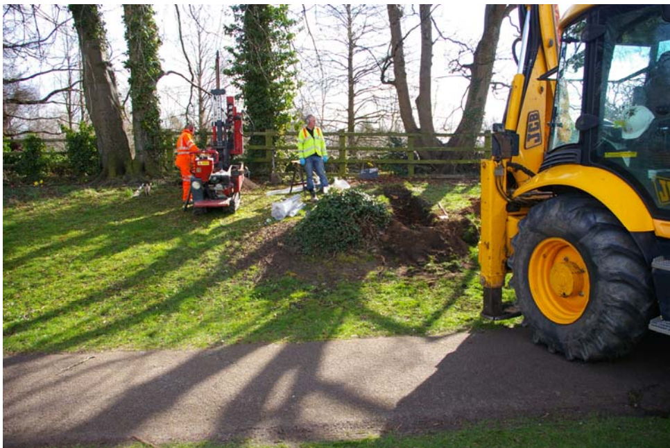
Figure 6 Location of trench Trench partially excavated. Looking east
