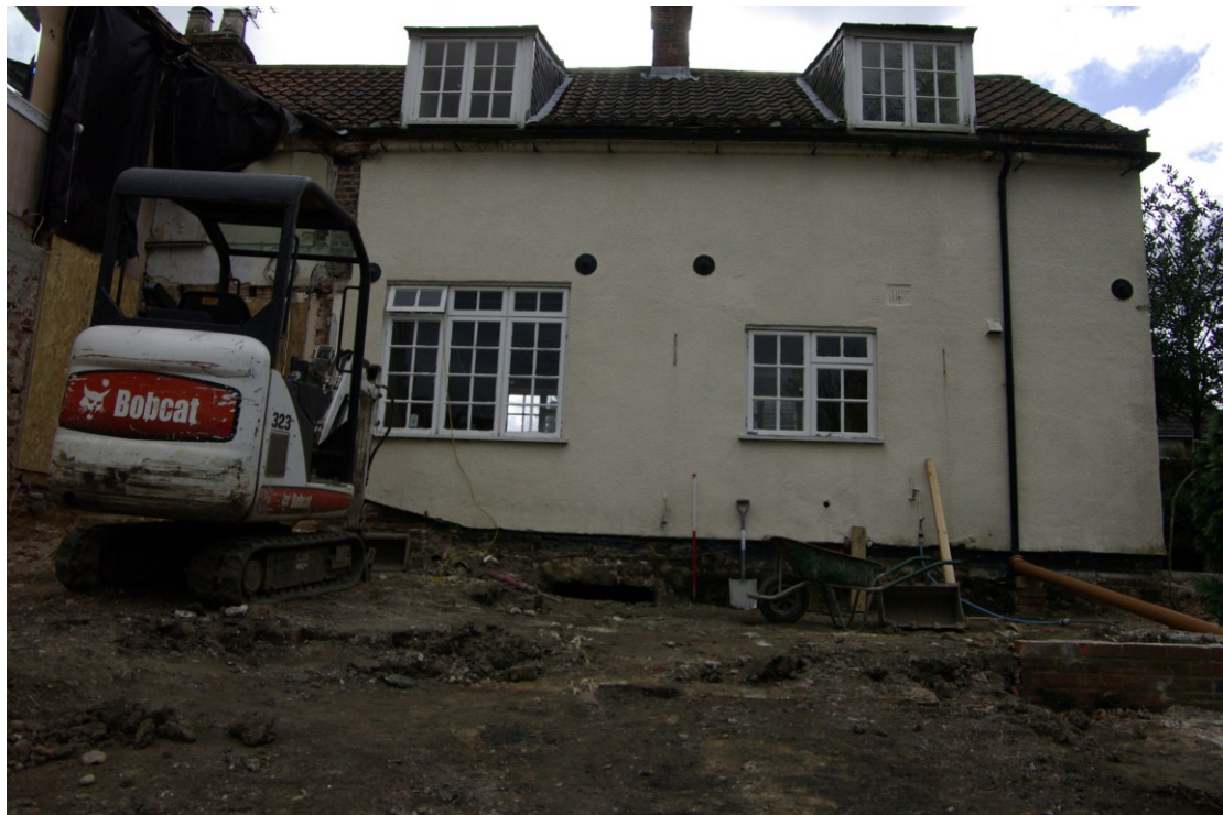
Figure 12 Underpinning of north-west facing elevation Looking south-east. 1m scale
