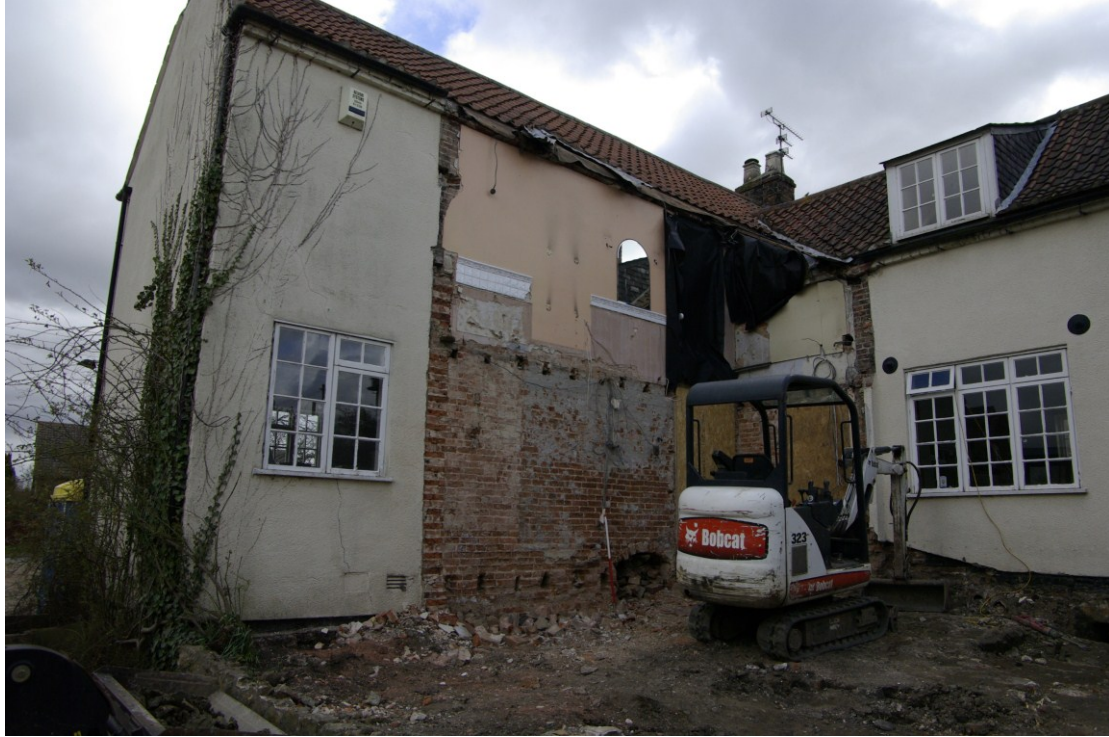
Figure 8 Demolished extension Looking north-east.
