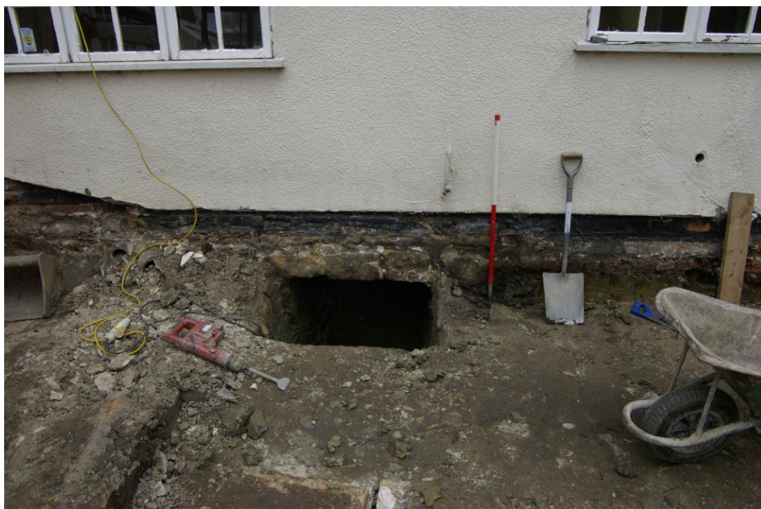
Figure 13 Underpinning close-up Looking south-east. 1m scale
