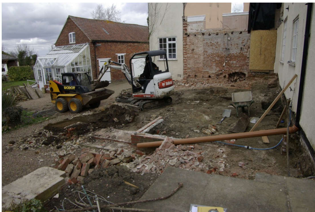
Figure 14 Yard, patio area Looking north
