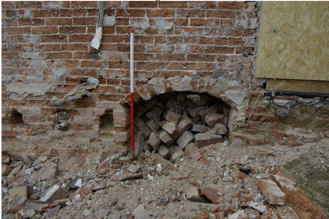
Figure 9 Head of archway leading into cellar Looking north-east
