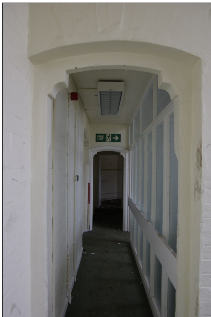
Figure 34. Pair of shouldered- arch doorway openings. Looking west along first floor passage.
