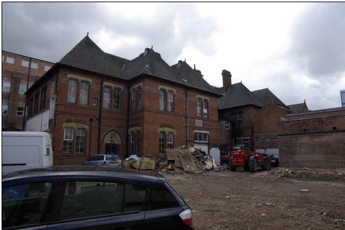
Figure 15. North-facing elevation, looking south-west.
