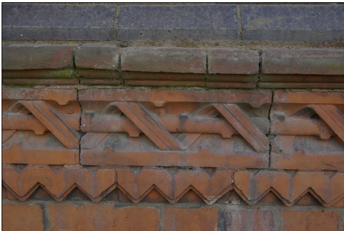
Figure 23. Detail of decorative brickwork string-course.
