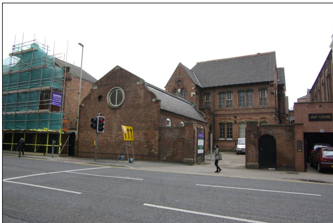
Figure 16. West facing elevation, with former art room fronting onto Oxford Street. Original boys' entrance is located on the left hand side. Looking east.
