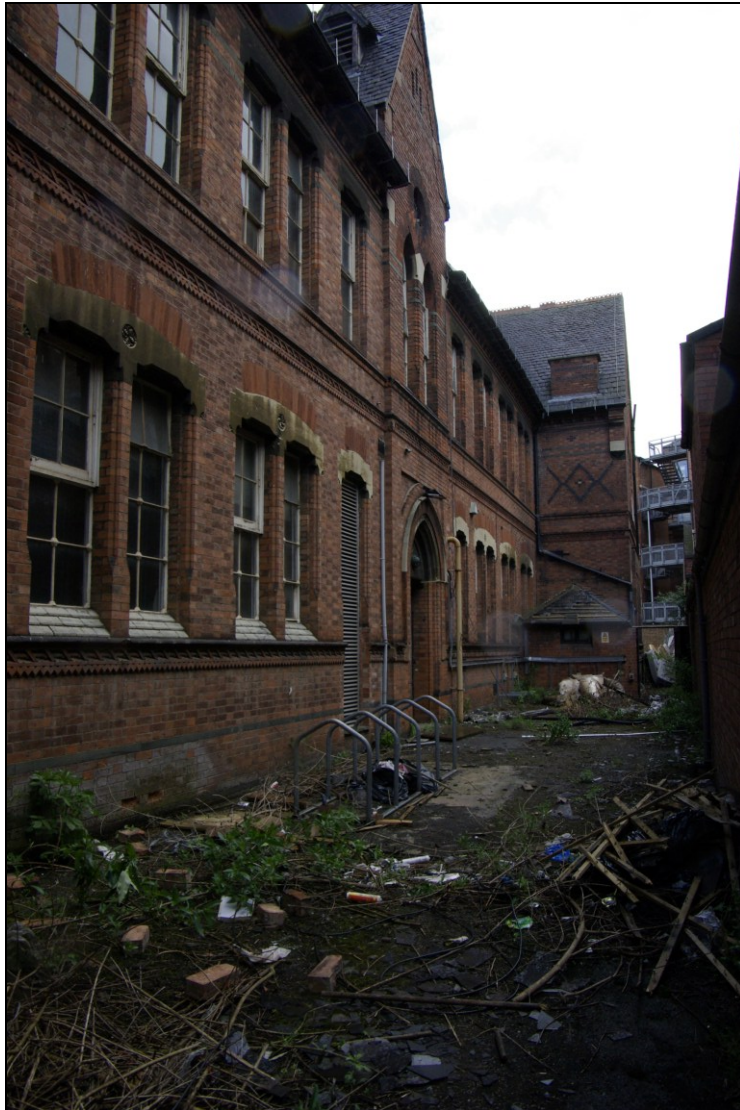
Figure 18. South-facing elevation, looking east.
