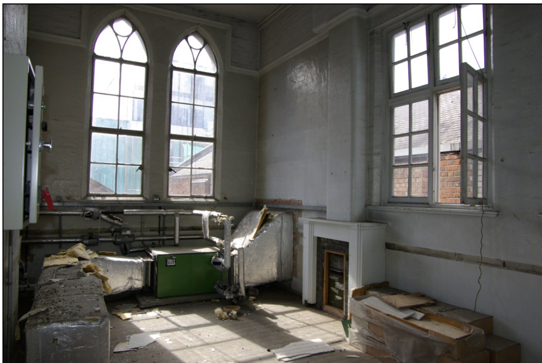
Figure 41. Former heated class-room, looking west.
