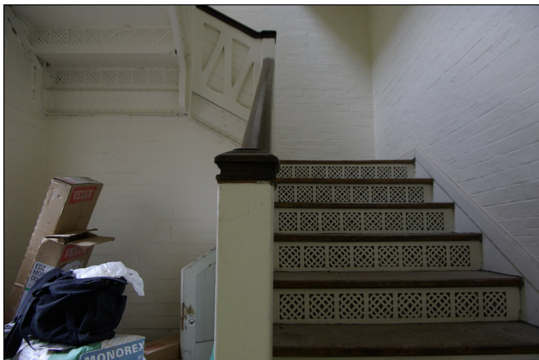
Figure 27. Boys' staircase, with cast-iron open-fretwork risers and oak treads. Looking east.
