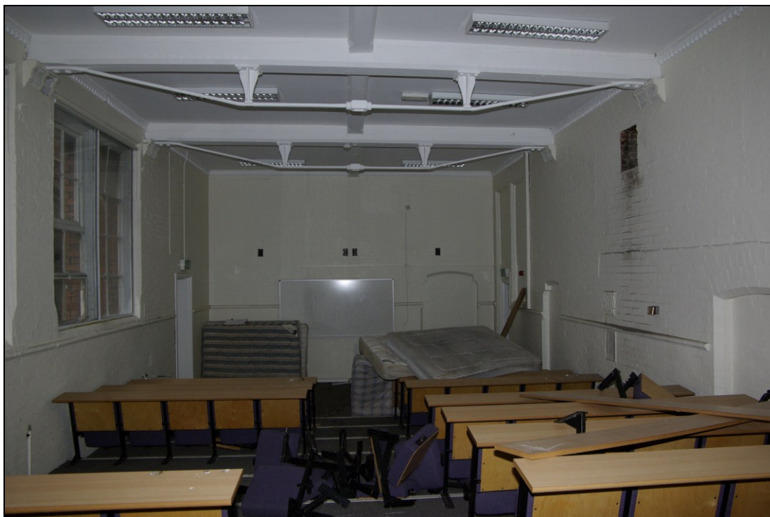
Figure 33. Former infants' school room, looking west, towards blocked doorway into nursery.
