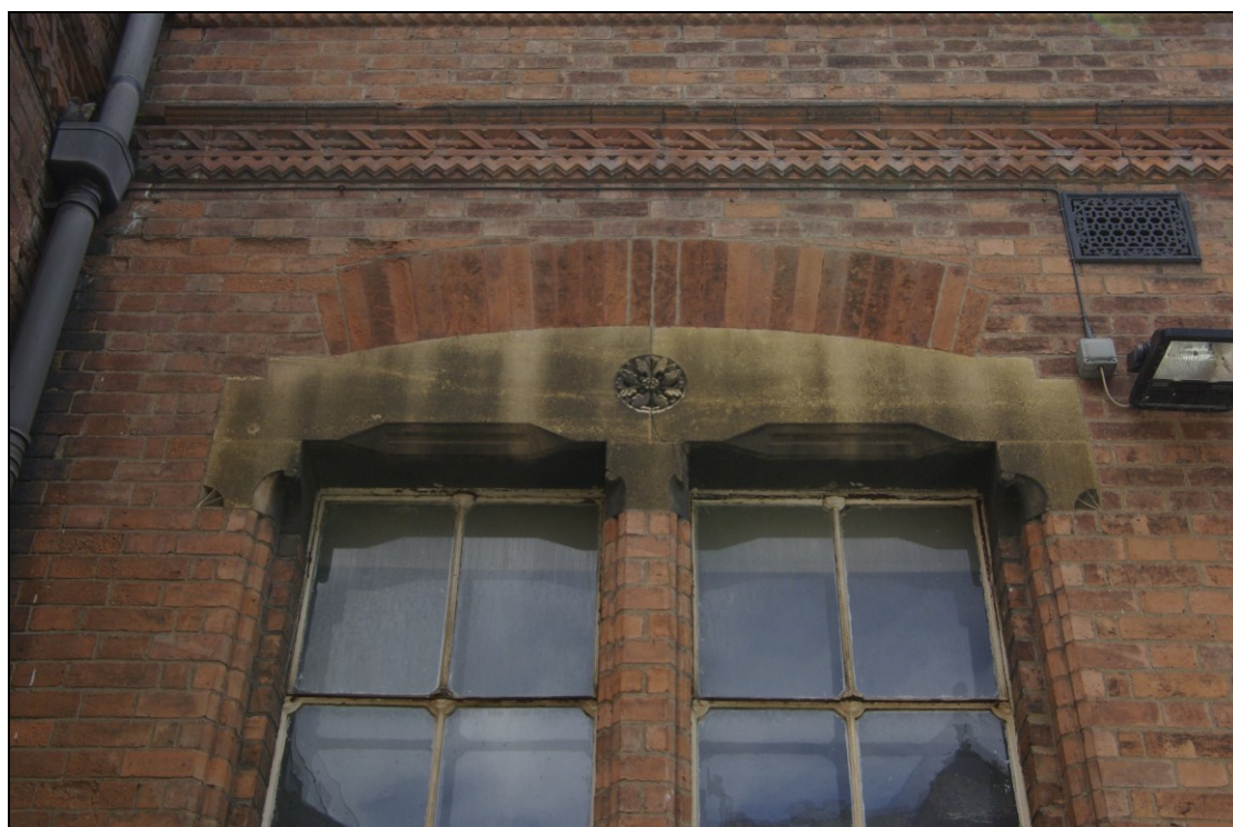
Figure 22. Decorative window head detail, looking east.
