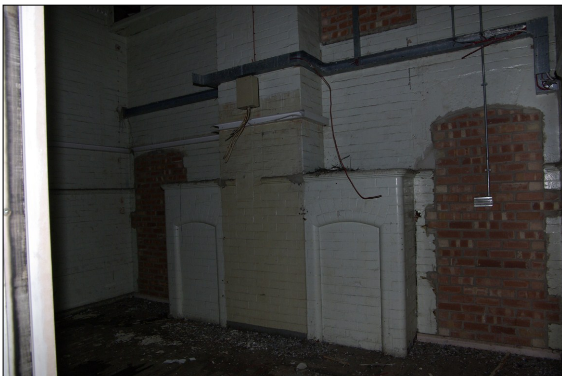
Figure 32. Blocked doorway and chimney openings within former class room. Looking south-east.
