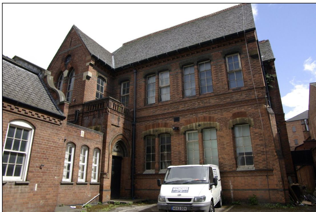
Figure 17. Detail of above. Looking east.
