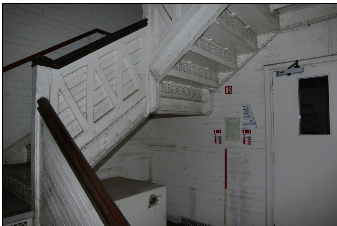
Figure 28. Girls' staircase, looking north.
