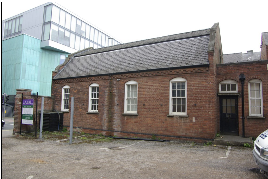
Figure 25. Former art room building of 1927. Looking north.
