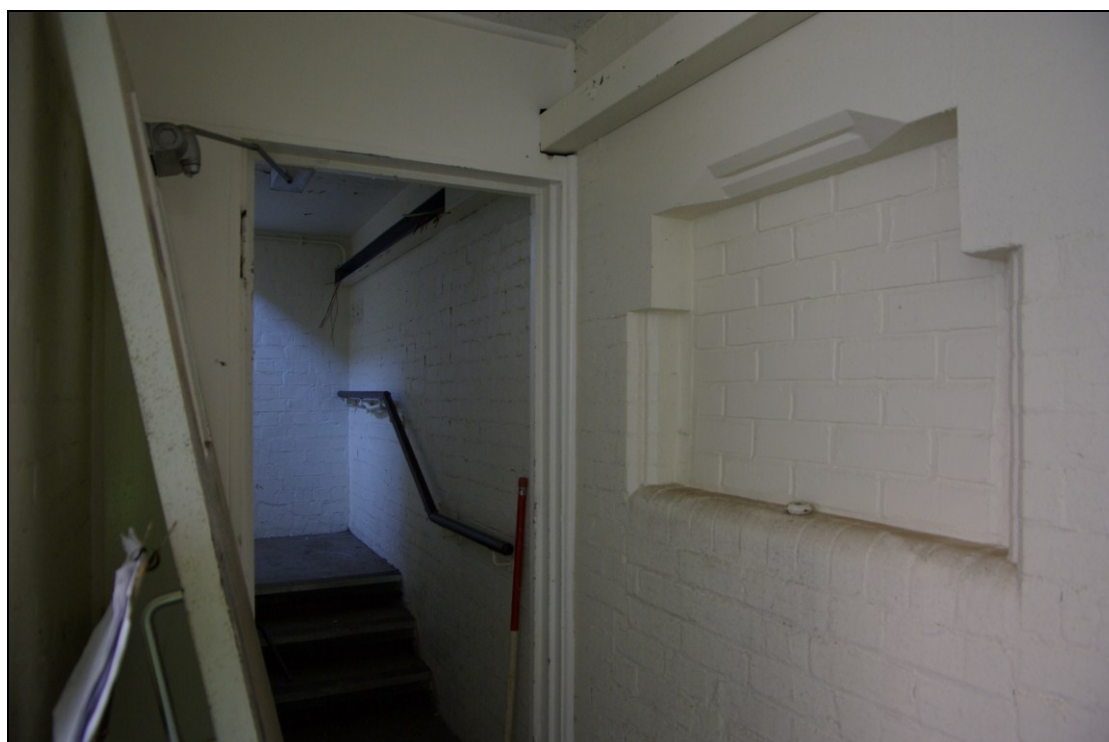
Figure 36. Blocked window opening within inserted stairwell. Looking south-east.
