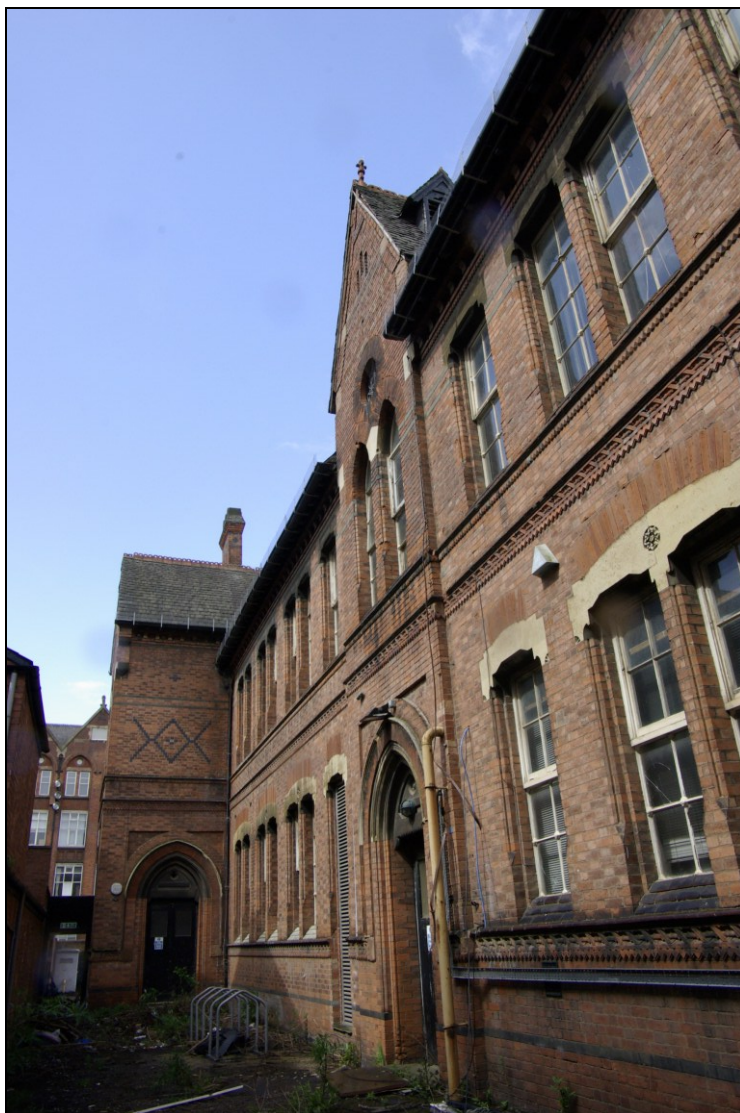
Figure 19. South-facing elevation, looking west towards former girls' entrance.
