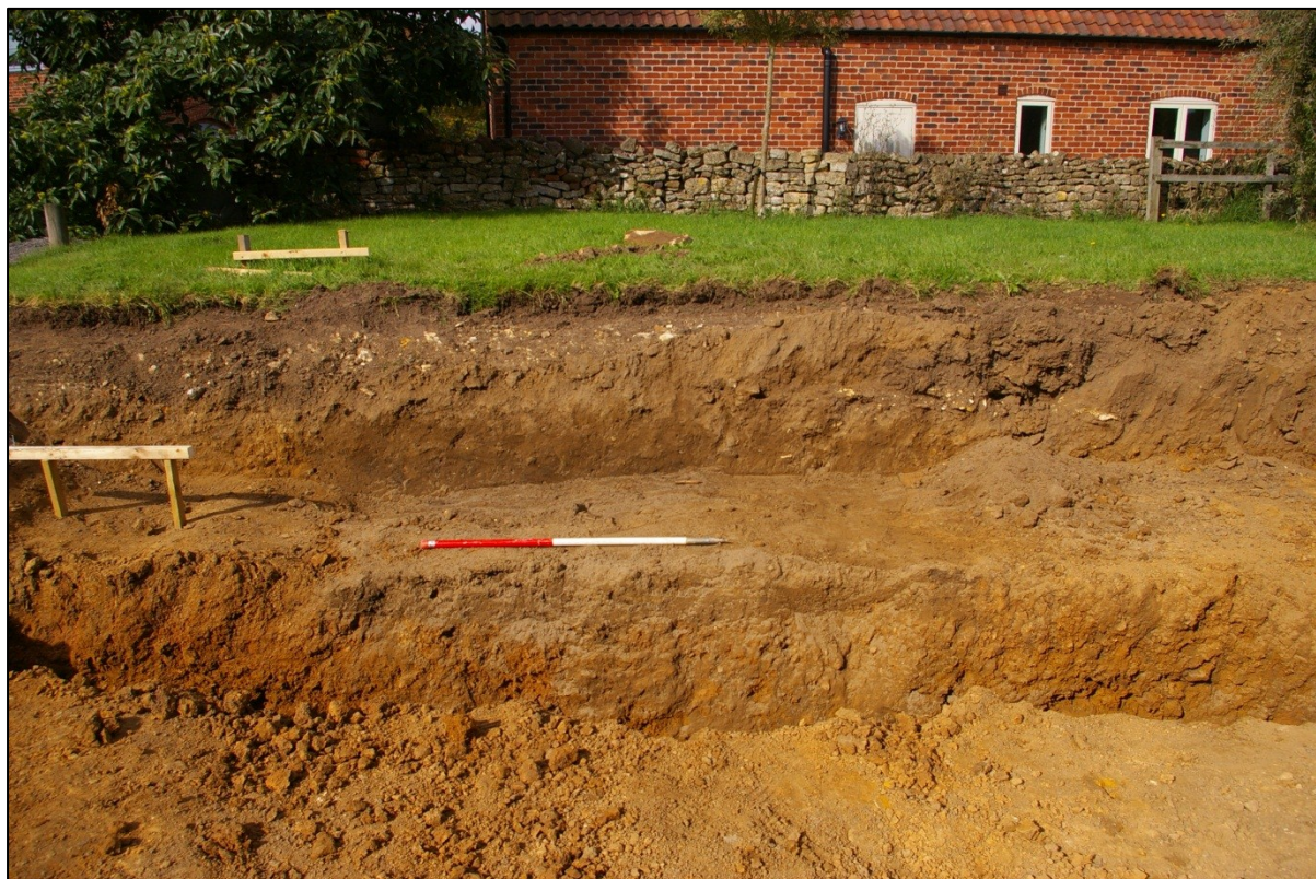
Figure 8. Section 1 of pit [2] and gully [4], following excavation of foundation trench. Looking west.
