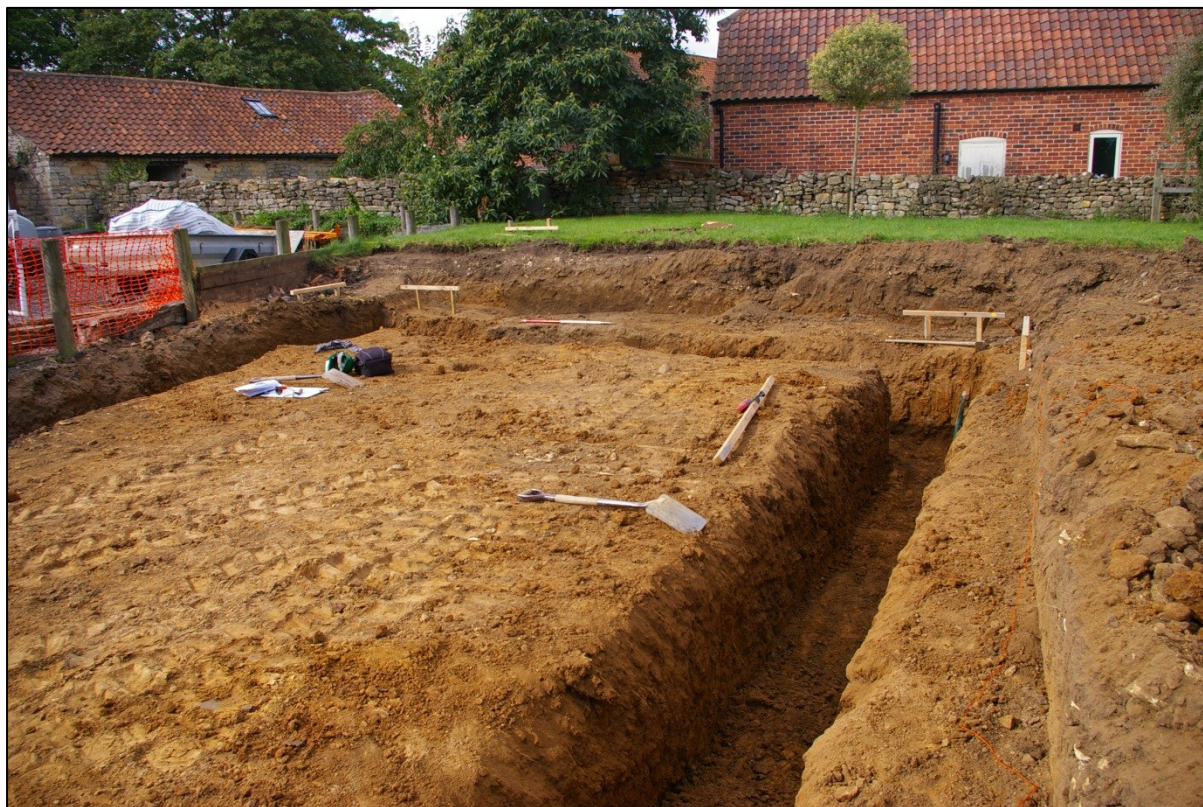
Figure 10. Fully excavated site, looking south west.
