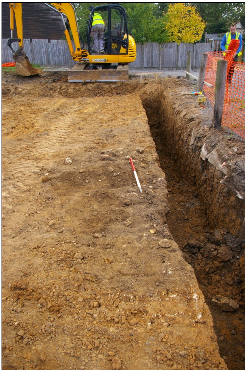
Figure 12. Possible pit (5) [6] looking south-east.
