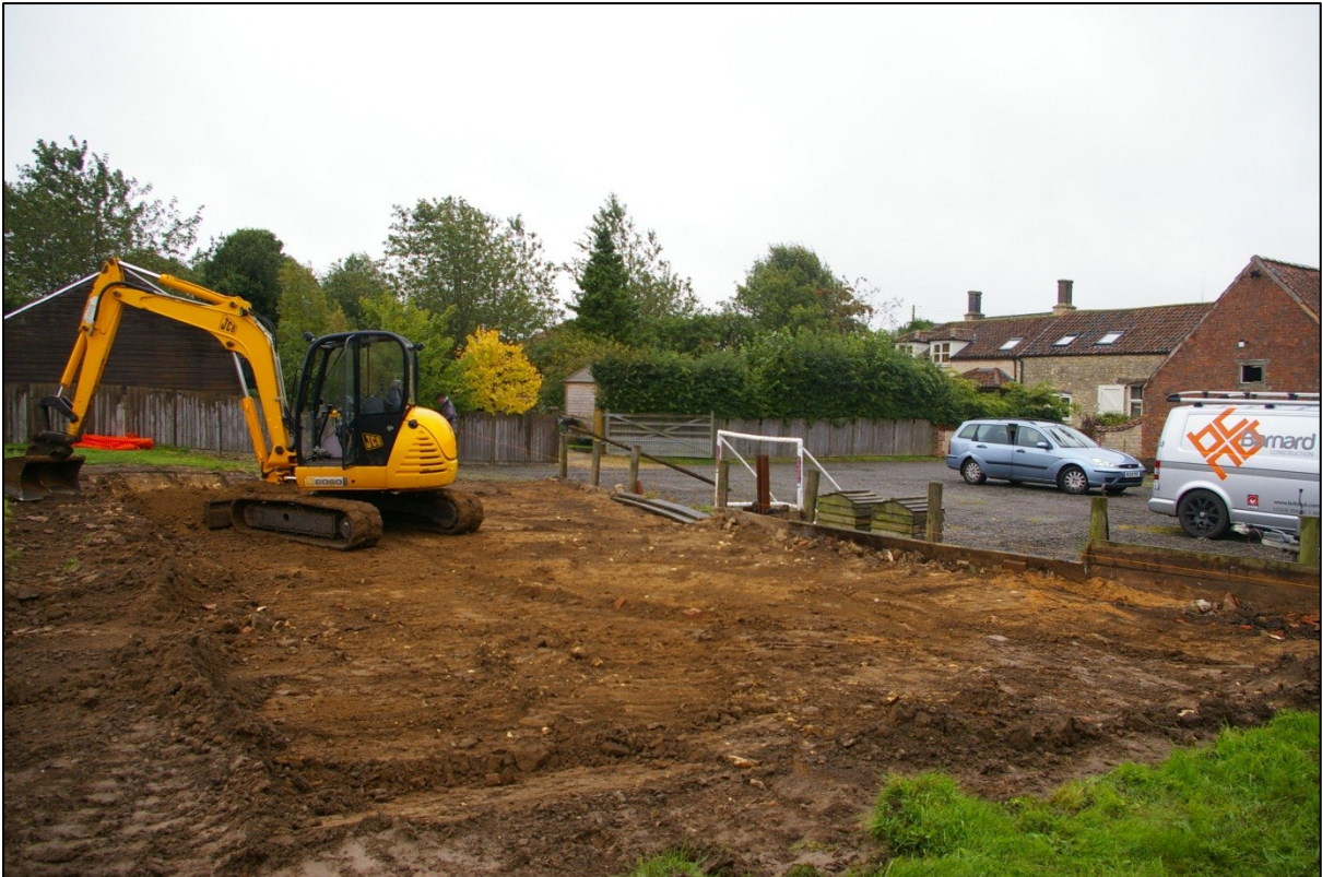
Figure 6. Topsoil stripping over footprint of new car port, looking south-east.
