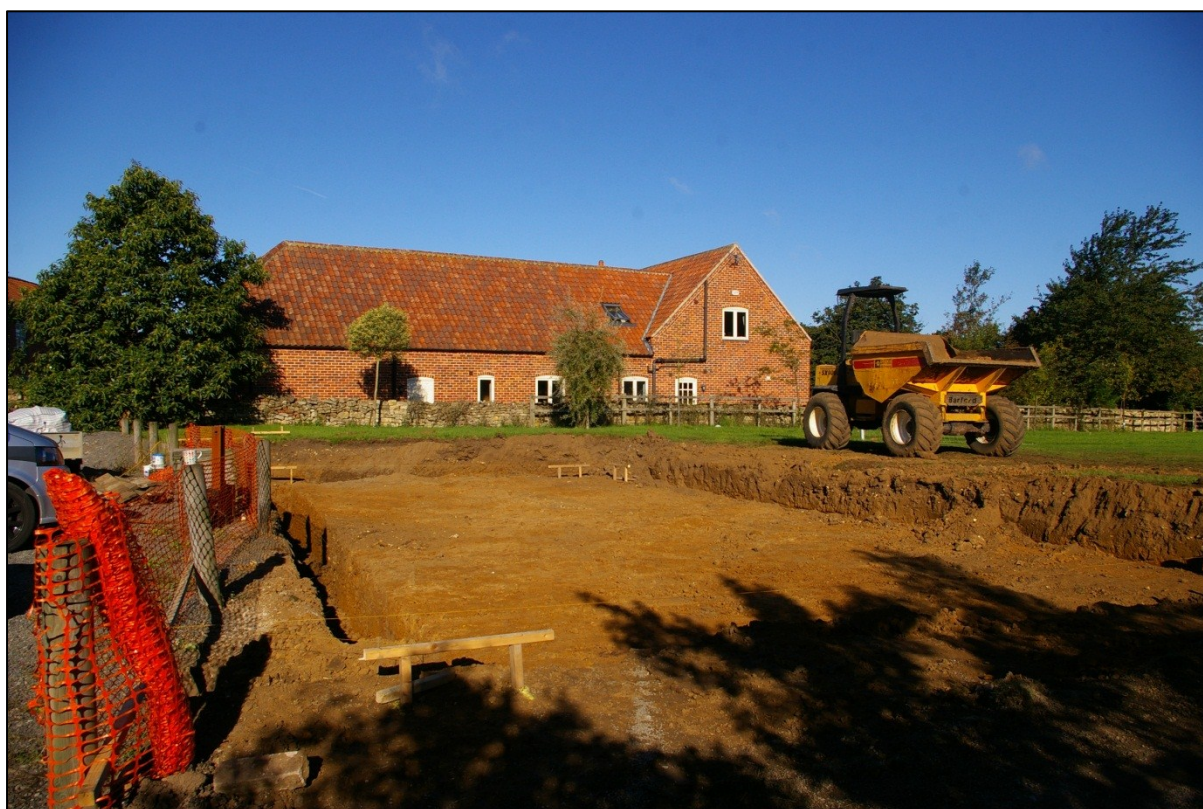
Figure 9. Fully excavated site. Looking north-west.
