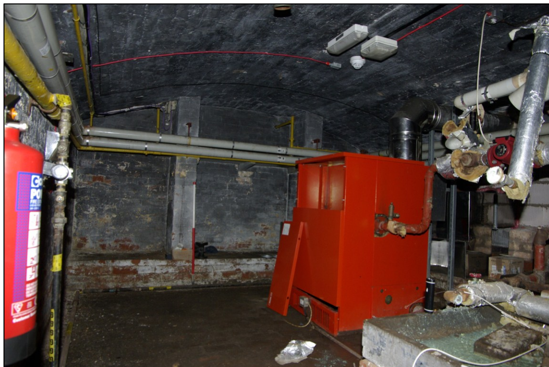
Figure 18. Cellar, main room Looking south-west. 1m scale
