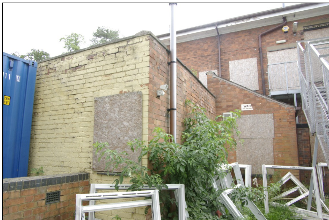
Figure 13. West facing elevation outbuildings Looking north-east
