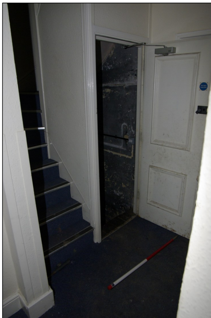
Figure 30. Servant's stairs, up to first floor and down to cellar Looking north-west. 1m scale
