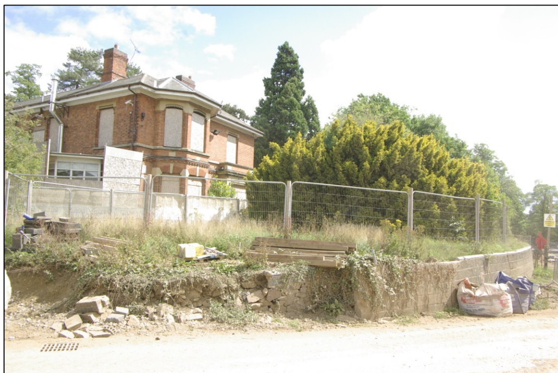
Figure 3. General view of The Woodlands and ha-ha Looking north-east
