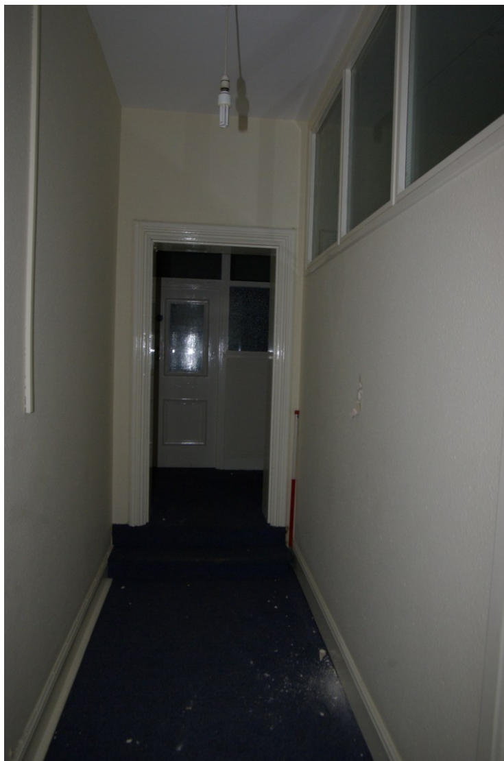
Figure 35. Corridor to Room F5 Looking north. 1m scale. Partition wall of Room F4 on right of picture.
