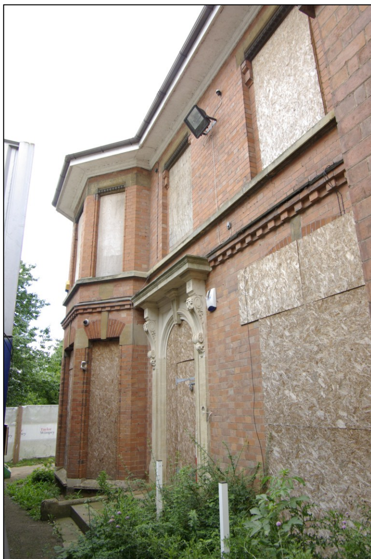
Figure 8. East-facing elevation front door. Looking south-west
