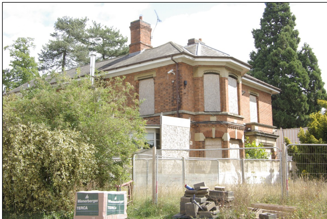
Figure 10. South facing elevation Looking north-east
