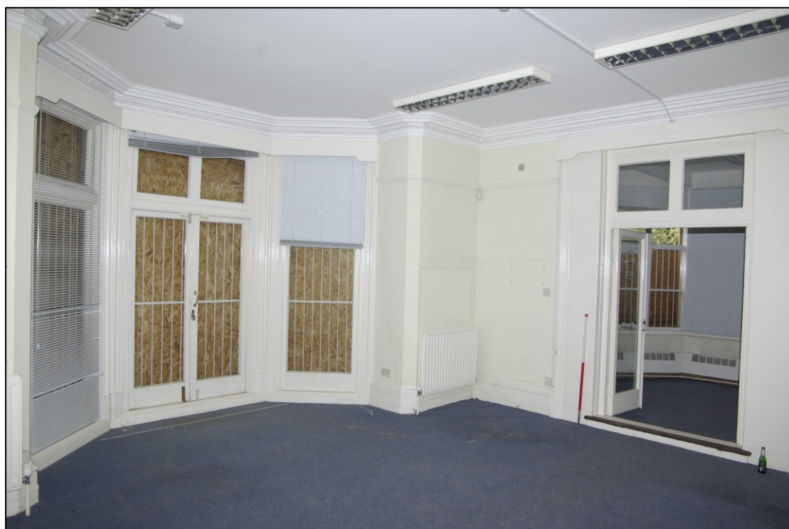
Figure 25. Room G2 Looking south-west. Conservatory on right of picture.
