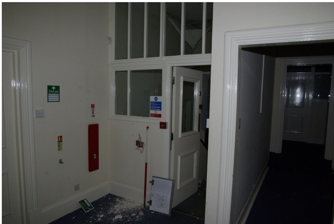
Figure 32. First floor landing Looking north-west. 1m scale. Stairs behind scale
