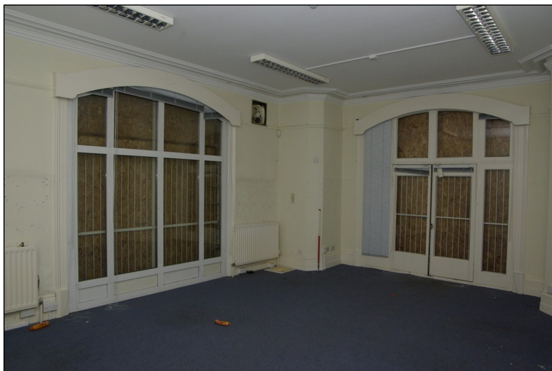
Figure 27. Room G5 Looking north-east. 1m scale
