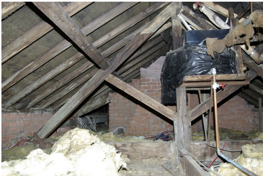
Figure 41. Roof structure Looking south
