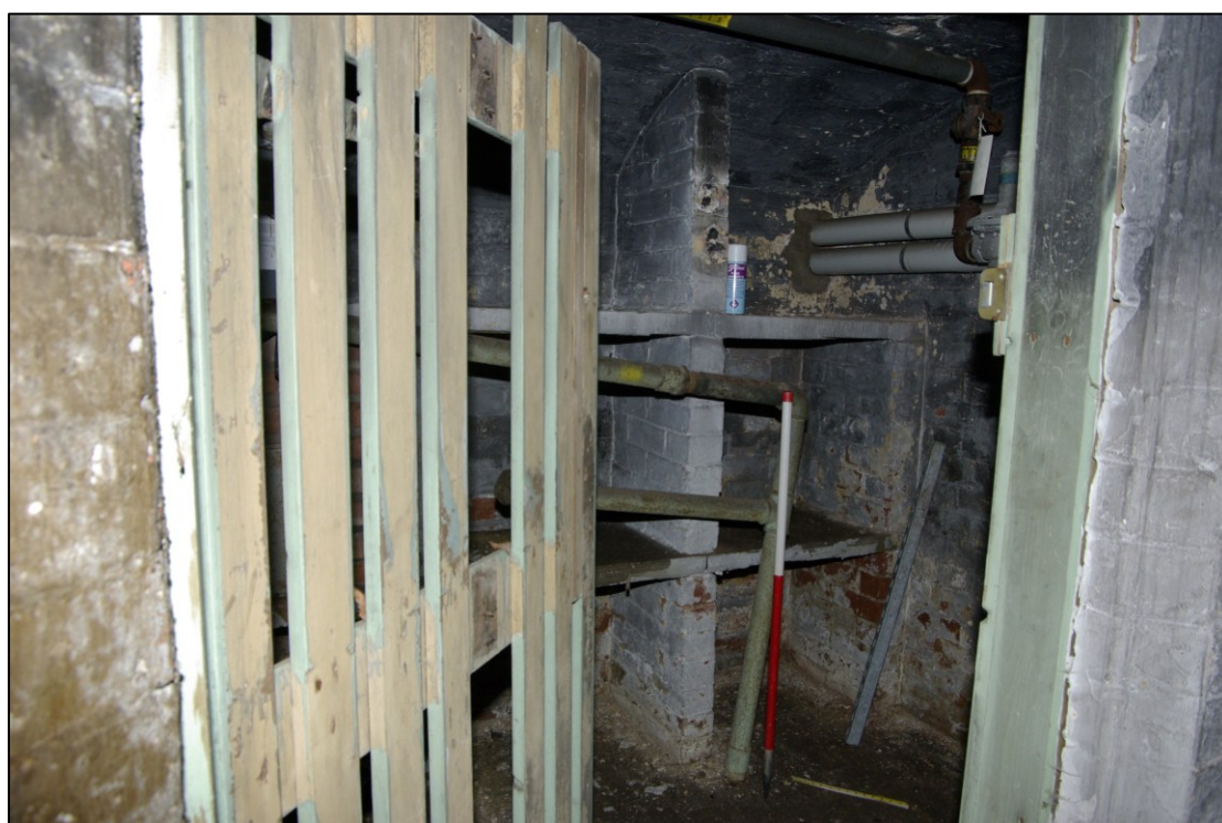
Figure 19. Cellar pantry Looking south-east. 1m scale
