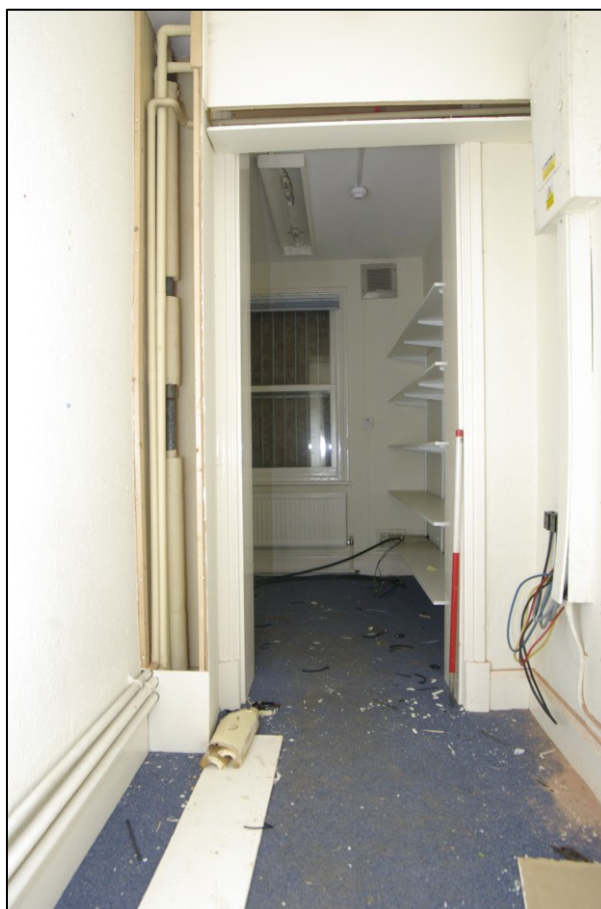
Figure 29. Room G7 Looking west. 1m scale
