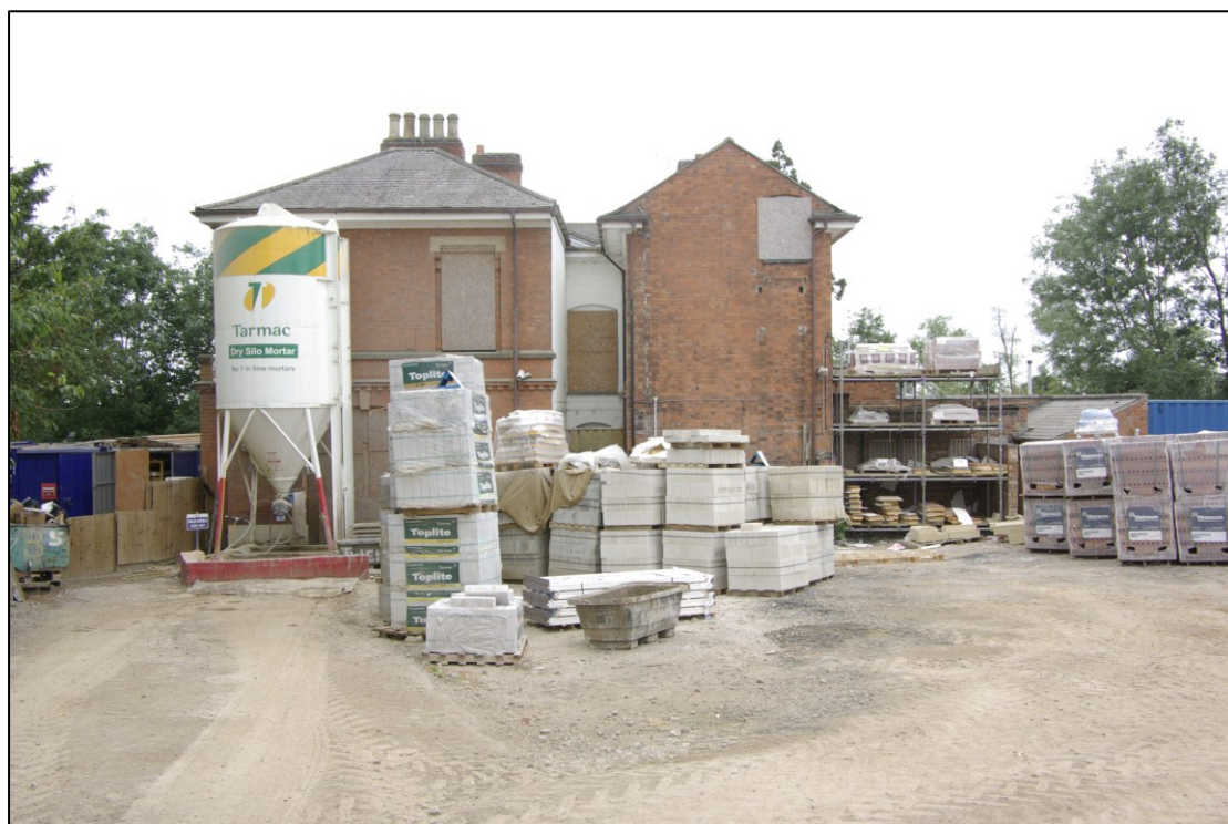
Figure 16. North facing elevation Looking south
