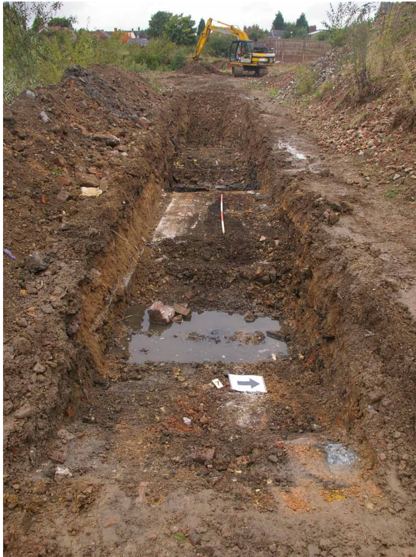
Figure 14. Trench 7 Looking west. 2m scale
