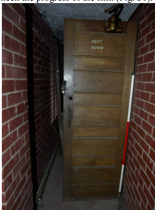
Figure 29. Rest Room door detail Looking south. 1.5m scale
