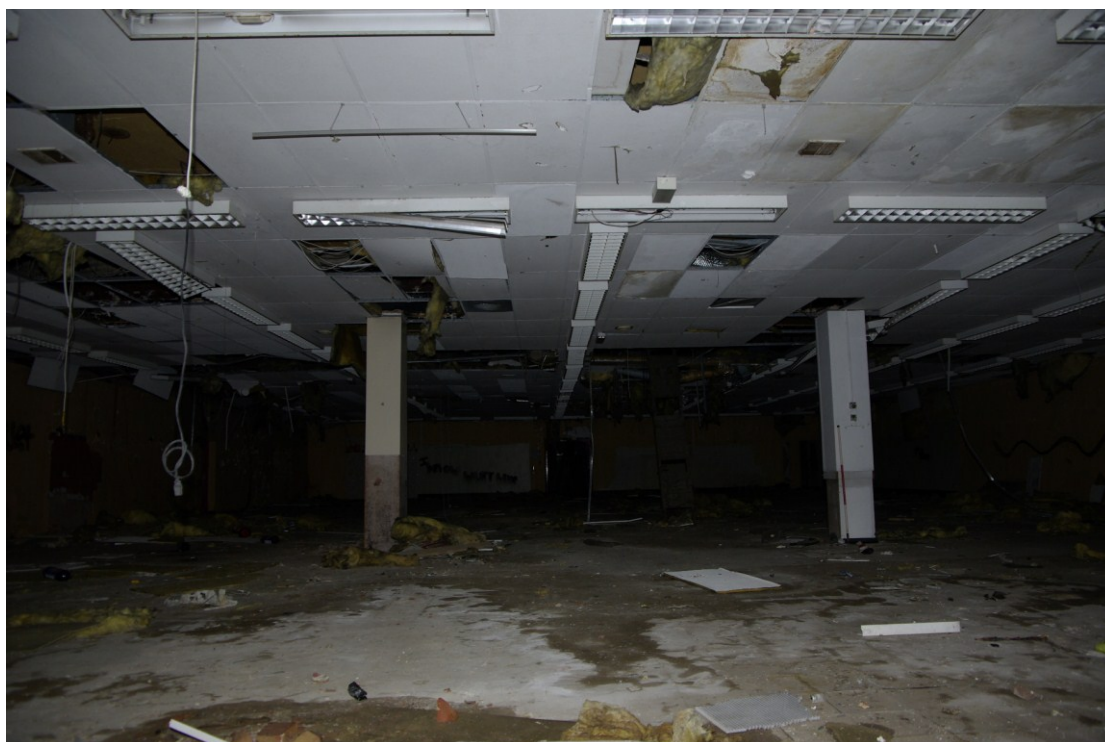
Figure 18. Main auditorium, ground floor Looking west. 1.5m scale
