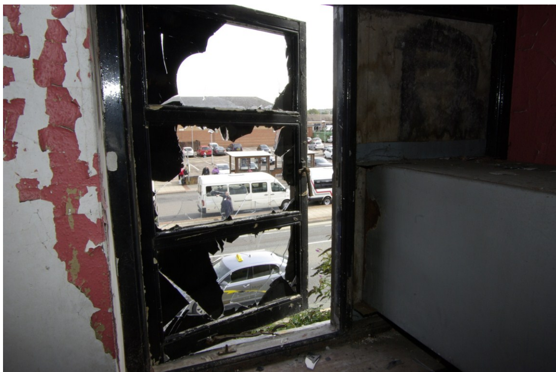
Figure 22. Window detail on first floor landing
