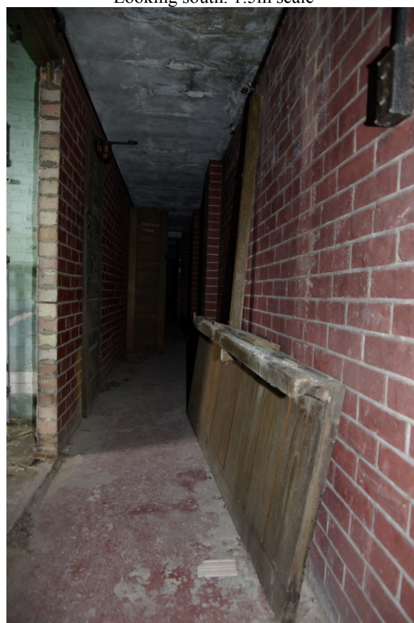
Figure 27. Projection Suite corridor Looking north from southern stairs
