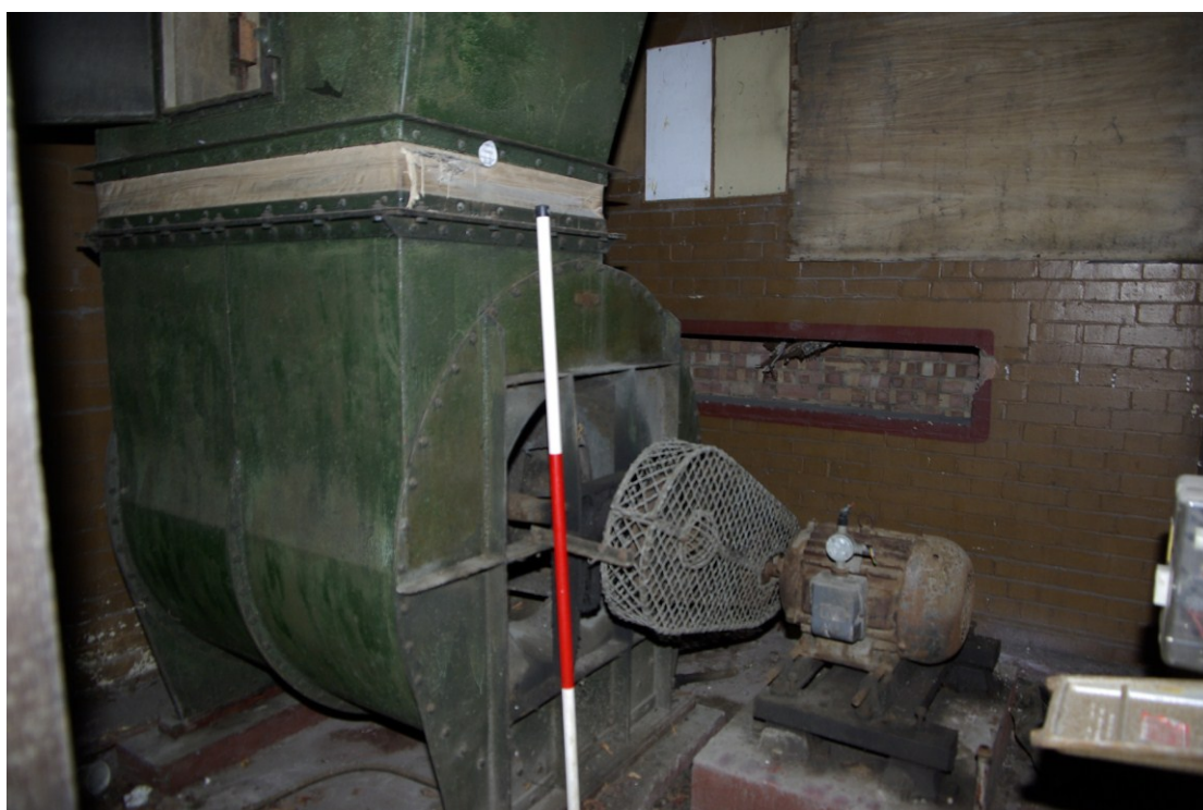
Figure 37. Ventilation/extraction room Looking south-west. 1.5m scale
