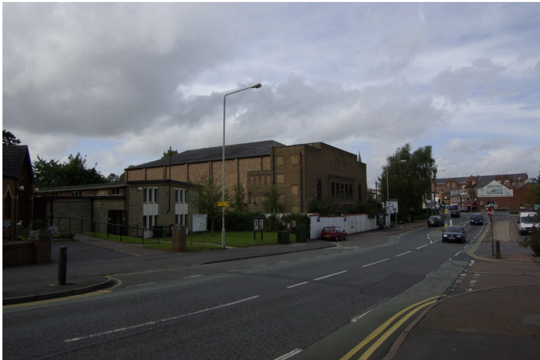
Figure 5. General view of site from Northampton Road Looking north
