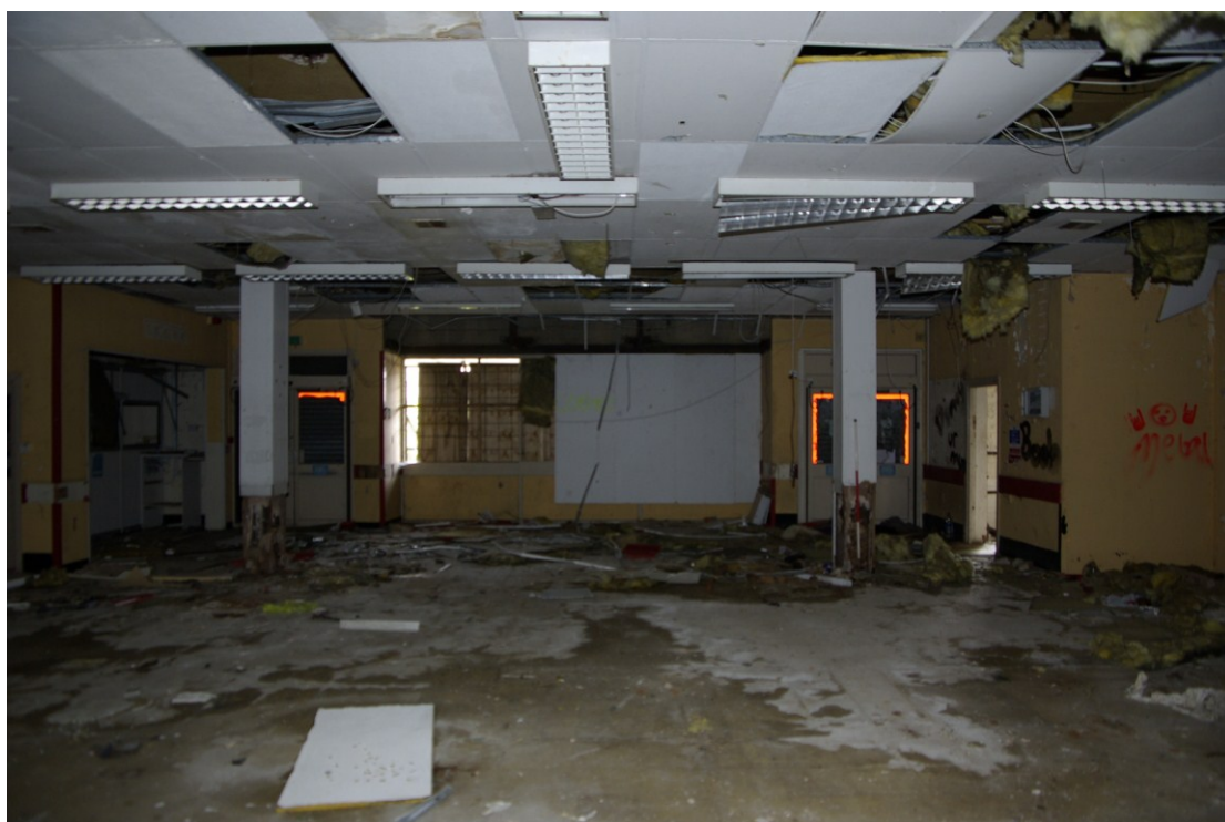
Figure 17. Ground floor entrance Looking east. 1.5m scale
