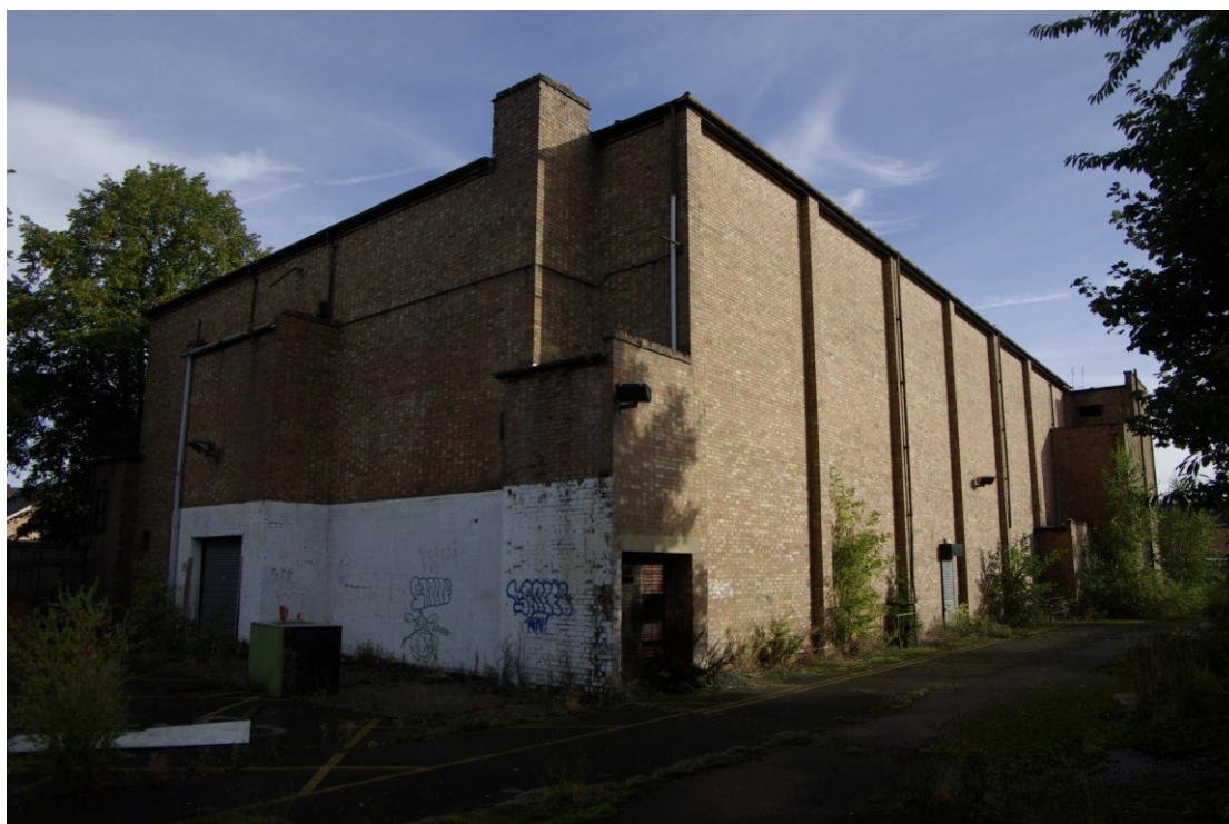
Figure 14. South and west elevations Facing north-east
