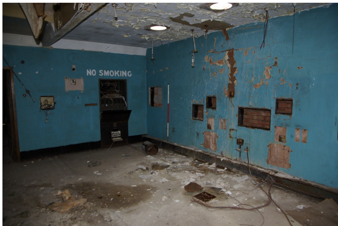
Figure 35. Projection Room Looking south-west
