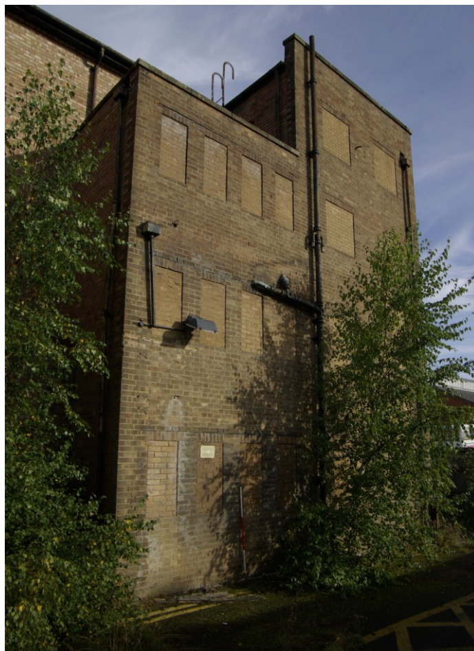
Figure 12. South wing blocked windows Facing north-east. 1.5m scale
