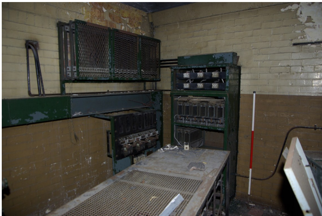
Figure 31. Rectifier Room Looking north-west. 1.5m scale
