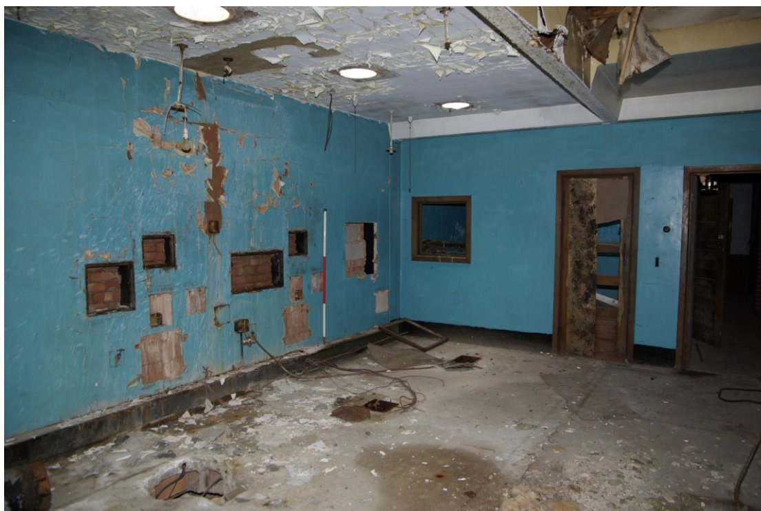
Figure 34. Projection Room Looking north-west. 1.5m scale
