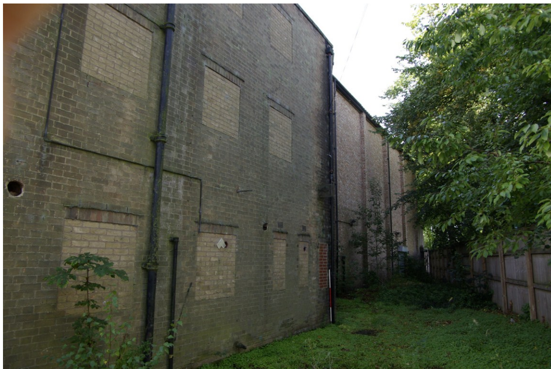
Figure 13. North facing elevation Facing south-west. 1.5m scale. Note different types of brick used in main façade (on left of picture) and those used on the main auditorium
