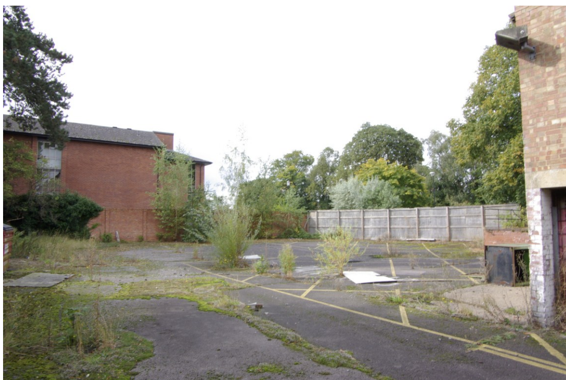
Figure 7. Rear yard to west of building Looking north-west
