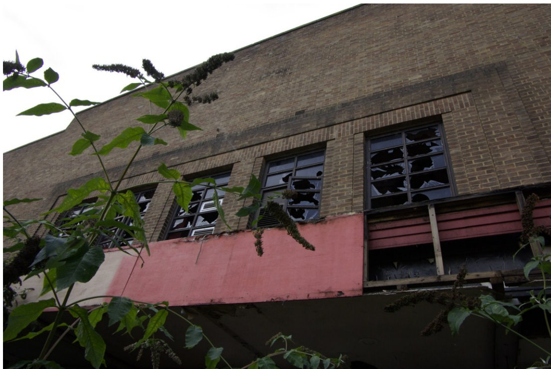
Figure 10. Window detail on east facing elevation
