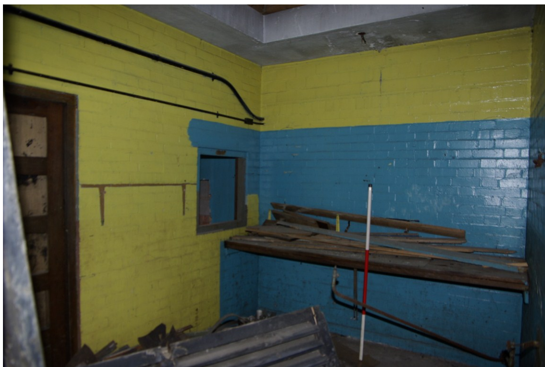
Figure 36. Room to the north of the Projection Room Looking south-west. 1.5m scale
