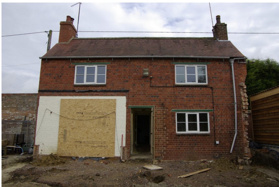
Figure 12. South-west facing elevation Looking north-east. 1m scale
