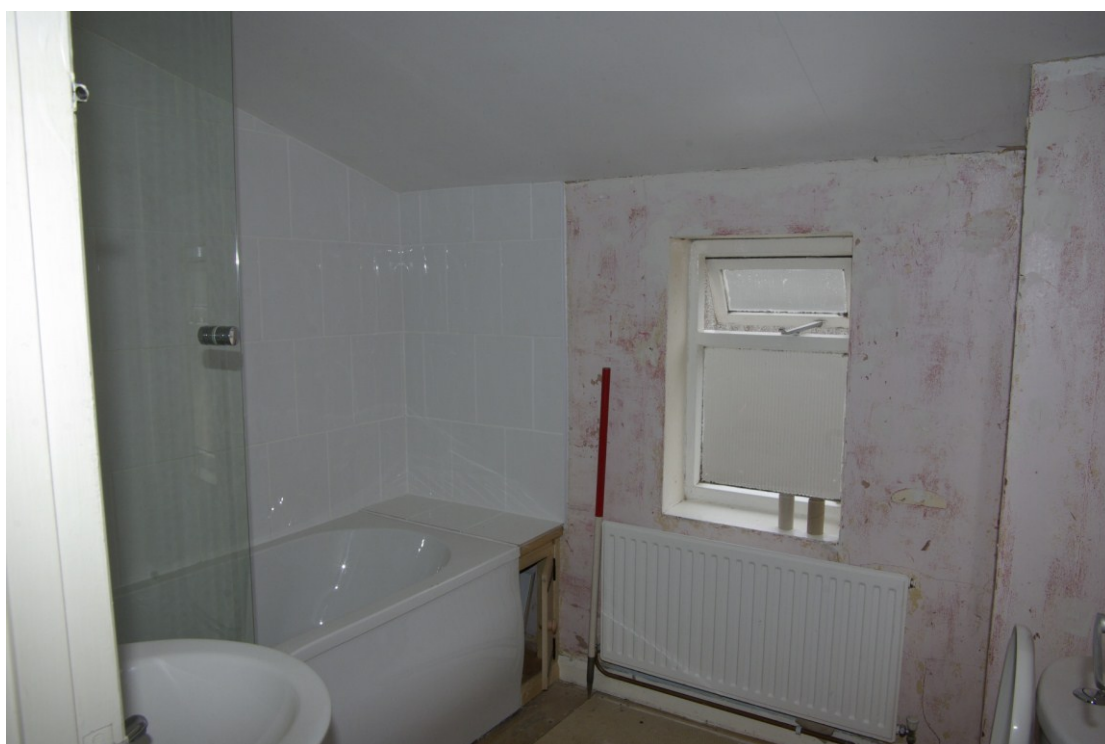
Figure 25. Bathroom Looking north. 1m scale
