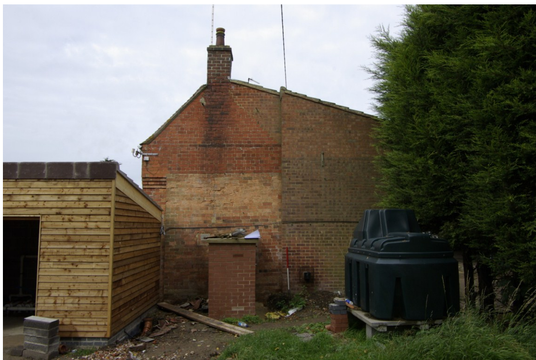
Figure 9. South-east facing elevation Looking north-west. 1m scale
