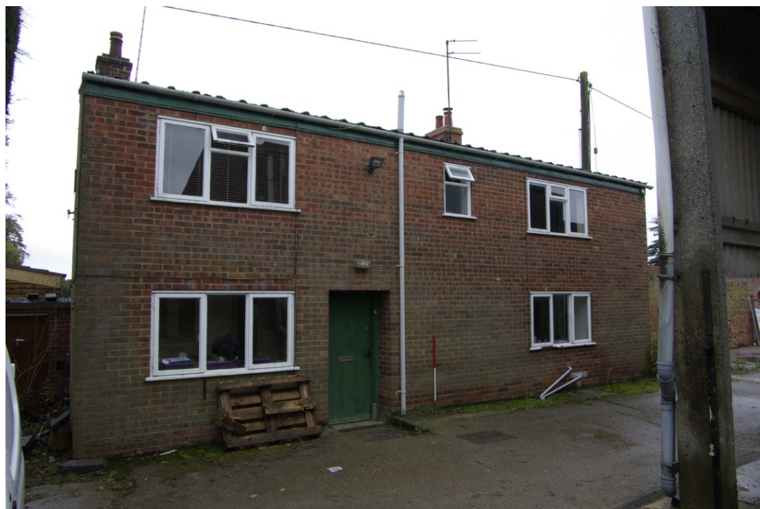
Figure 8. North-east facing elevation Looking south-west. 1m scale
