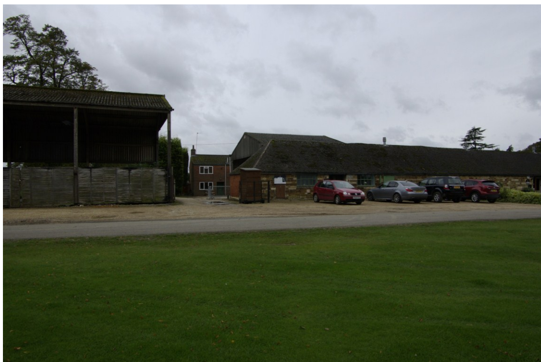
Figure 5. Gardens Cottage seen from the east Looking south-west
