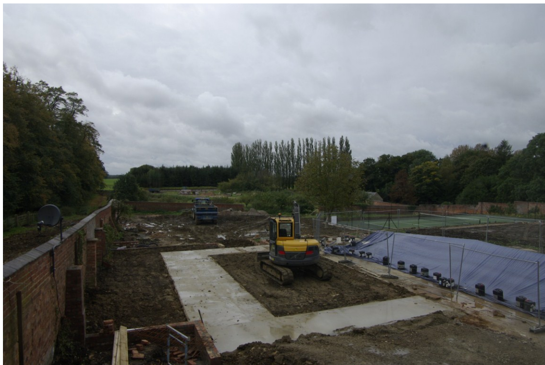
Figure 20. Walled garden seen from Bedroom 1 Looking west
