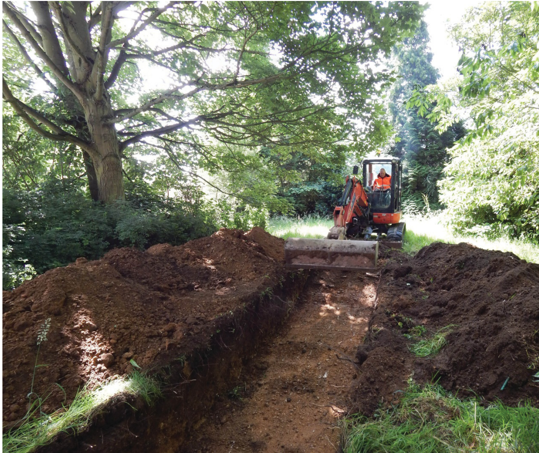
Plate 2: Work in progress, looking south
