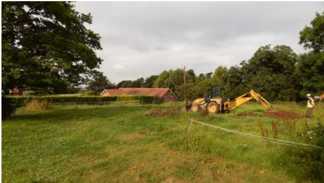
Plate 1: Work in progress on Trench 01, looking south-west
