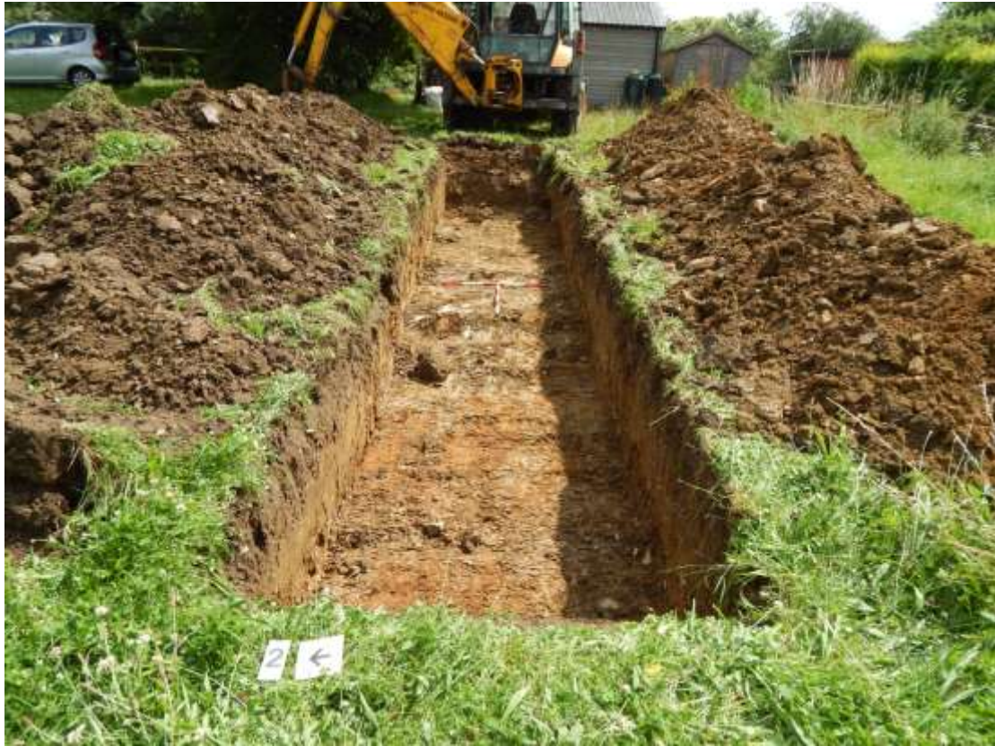
Plate 4: Trench 02, post-excavation, looking east
